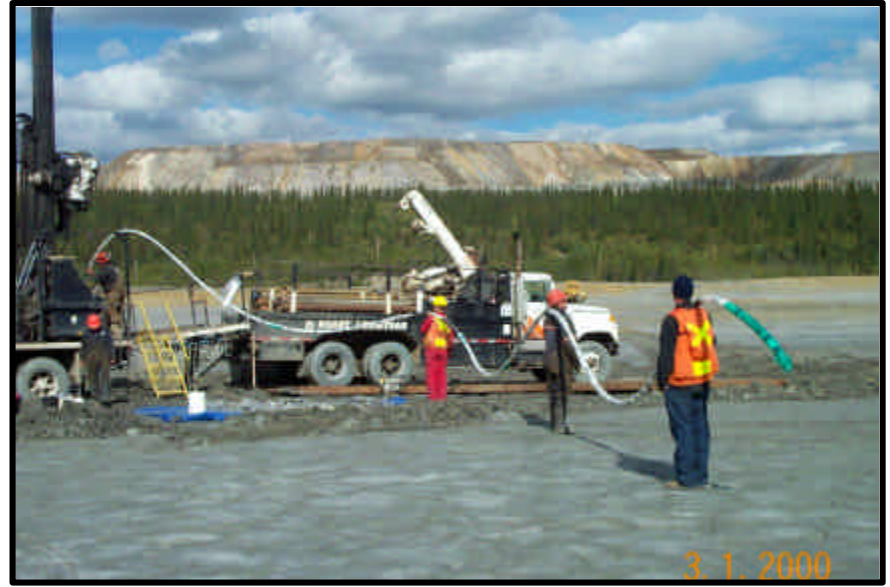
Installation of multi-level well down casing
