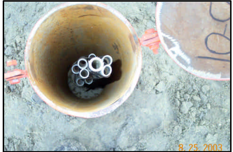
Completed multi-level well with steel protective casing
