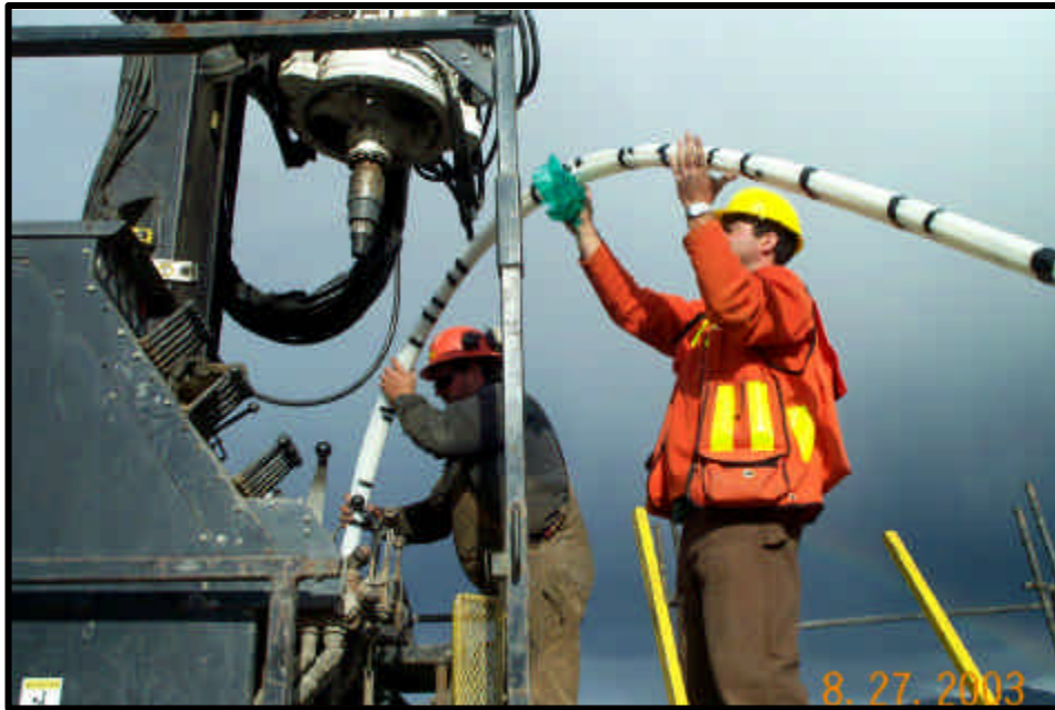
Installation of multi-level well showing removal of protective wrapping from screens prior to installation
