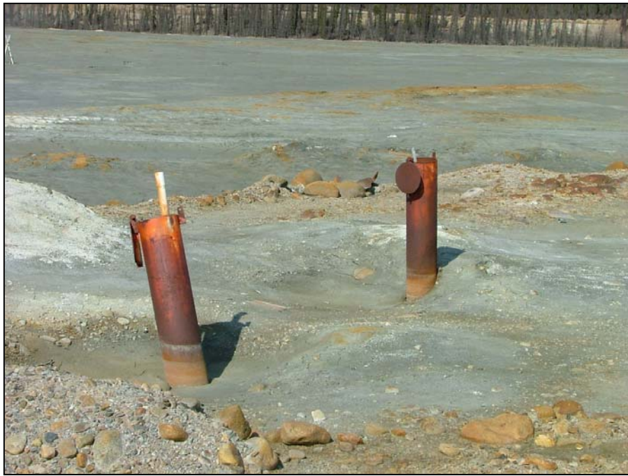
Old wells near P01-07. Casing and/or well appear to have heaved.
