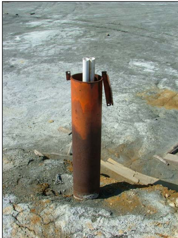
Old wells near P01-07. Casing and/or well appear to have heaved.
