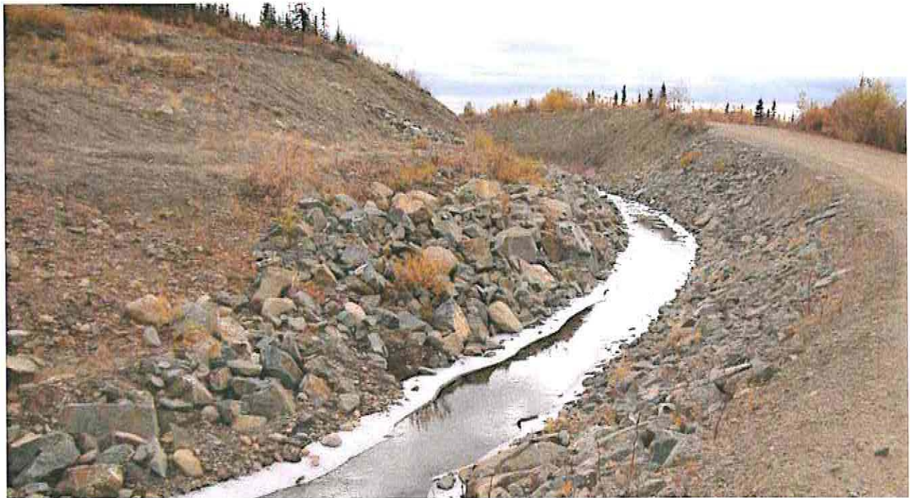
Photograph 9: Downstream view of stabilized channel conditions of Faro Creek Diversion Channel
