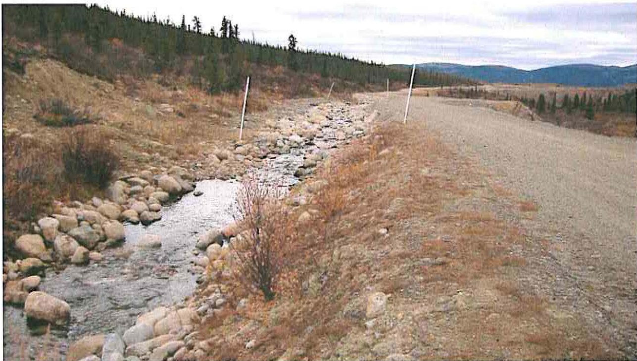
Photograph 8: Downstream view of lined channel conditions of Faro Creek Diversion Channel
