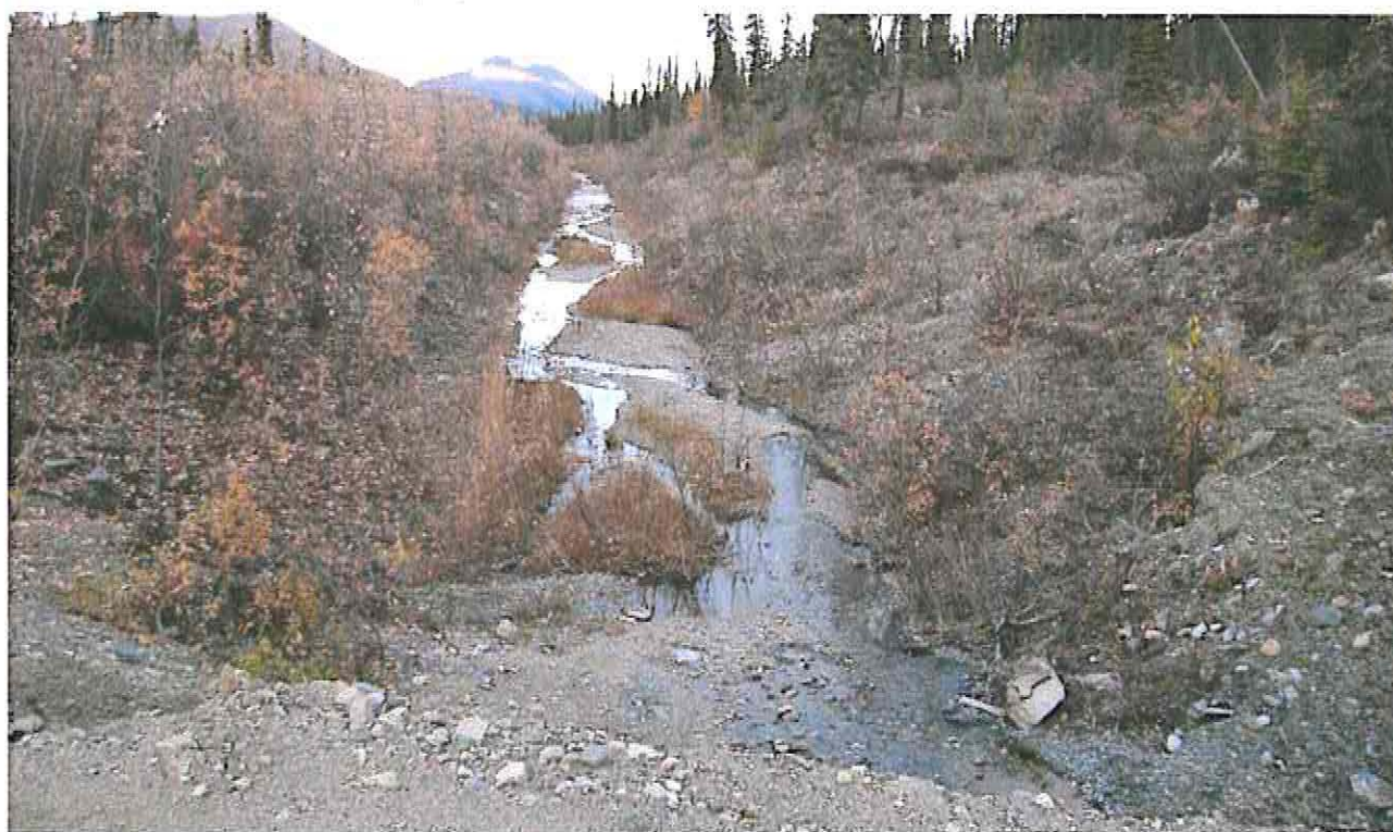
Photograph 2: Sedimentation downstream of well access crossing of North Valley Wall Interceptor Ditch
