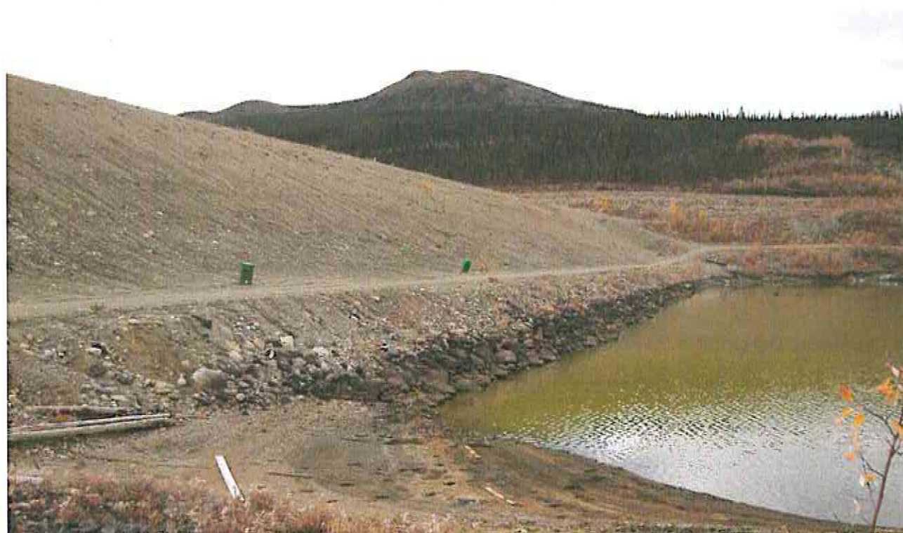
Photograph 4: Downstream drawdown operating conditions at Intermediate Dam
