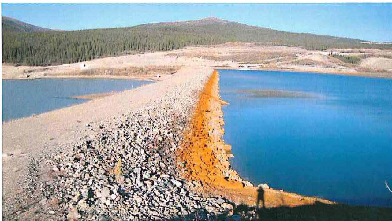
Photograph 3: Upstream drawdown operating conditions at Intermediate Dam
