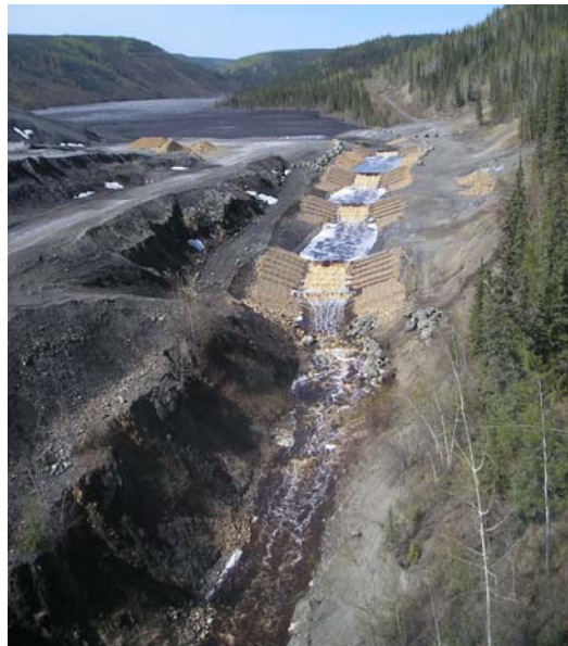
Gabion Drop Structures at Hudgeon Lake Outlet (2005)
