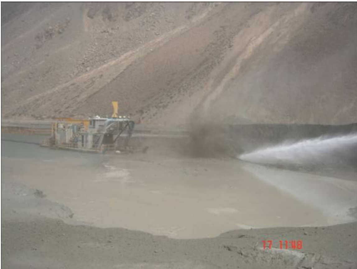
Figure 6.11: Operation of the dredge with monitor assisting. In order to speed up the process, monitors were put in place to enhance the density of the slurry reporting to the dredge. A cyclone station will be installed to thicken the slurry
