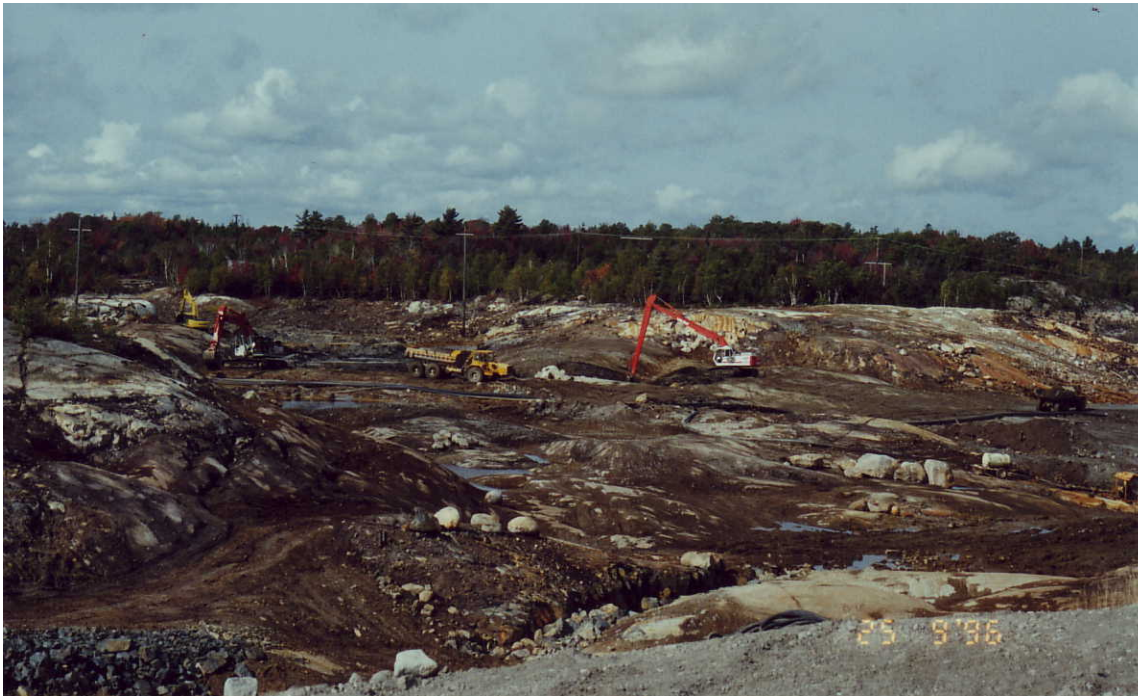
Figure 5.3: Excavators and articulated trucks removing tailings from bedrock
