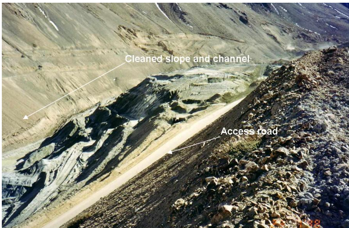
Figure 6.6: Copihues dam showing partial removal of tailings. Note the steps.
