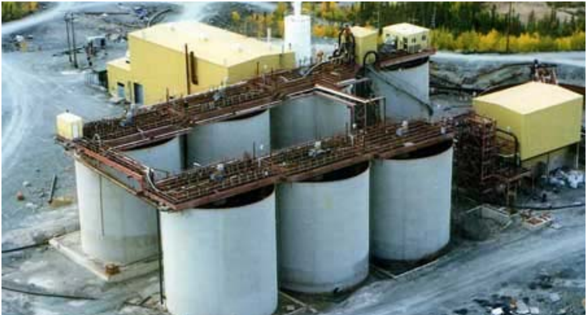
Figure 1.1: Giant Yellowknife TRP Carbon-In-Leach (CIL) tanks
