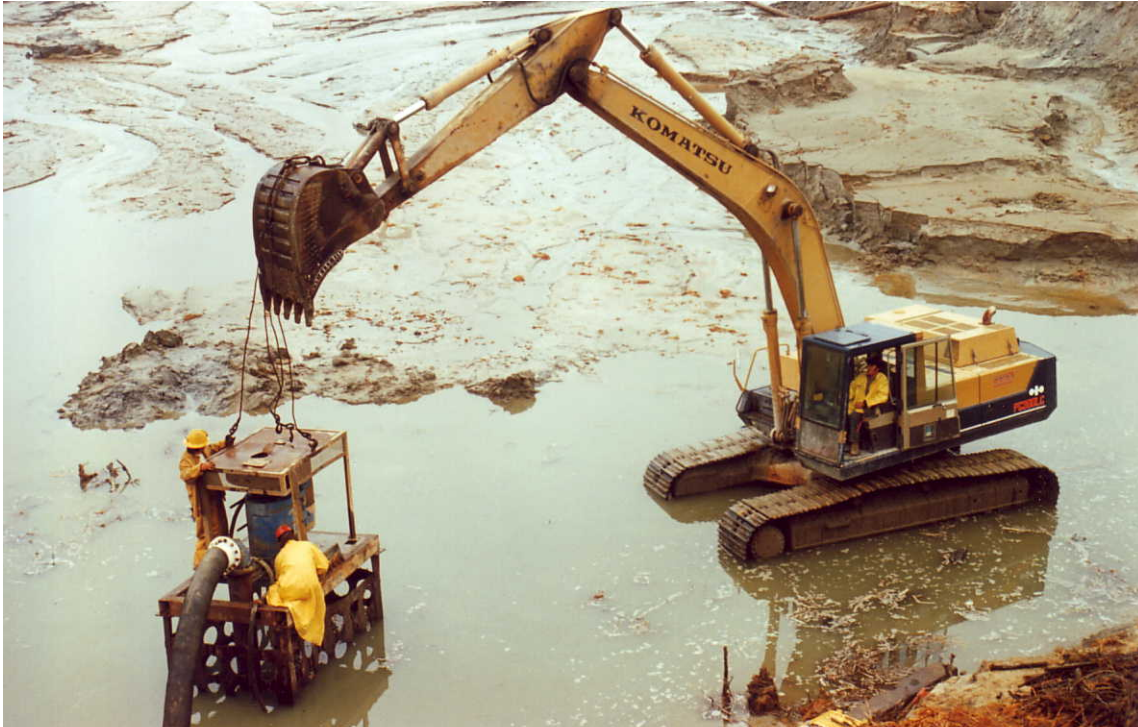
Figure 3.2 An example of a vertical cantilever sump pump and supporting perforated box being moved with an excavator. (Photo: Denison Environmental Services)
