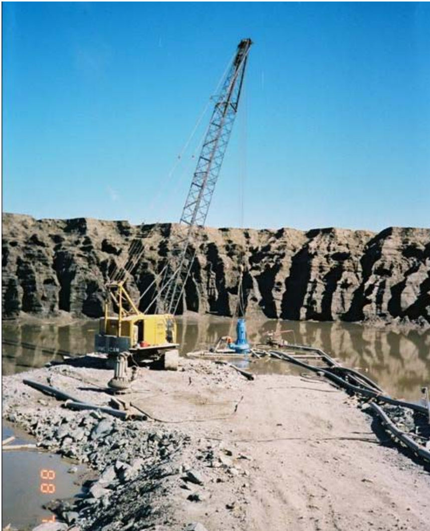
Figure 1.6: Crane and Toyo submersible sump pumps on rock-fill ramp
