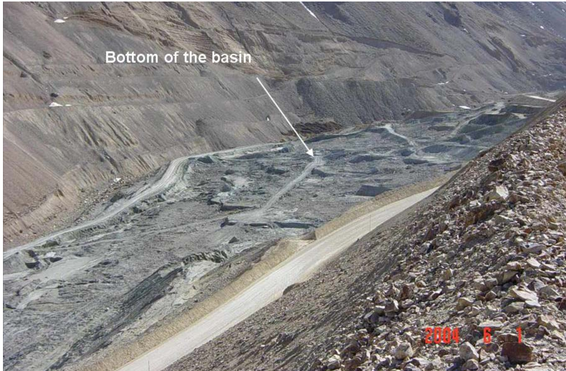
Figure 6.7: State of Copihues dam as at June 2004. Note the bottom of the basin is not completely cleaned as the monitors cannot remove the final layer of tailings due to limitations of hydraulic head to make it flow down stream.
