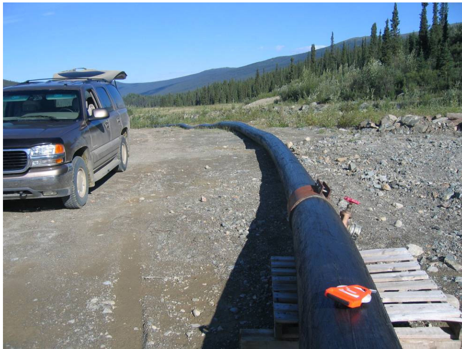
Photo II - 2 – Cross Valley Dam Syphon HDPE.
