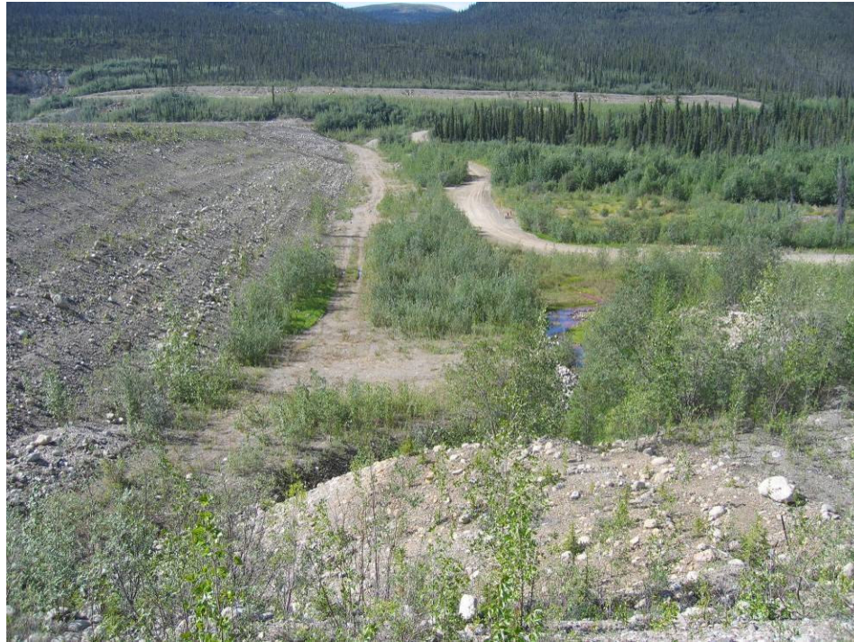
Photo II - 13 – Cross Valley Dam – Downstream slope from right abutment looking north. Note low trees on toe as shown on Photo II-5 from crest.
