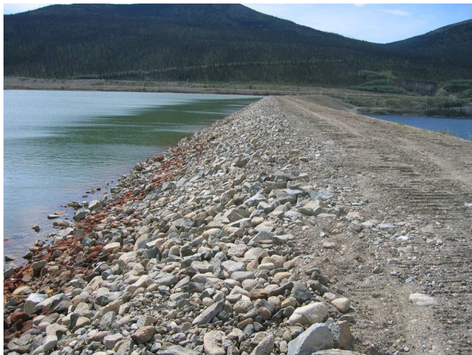
Photo II - 18 – Intermediate Dam – Upstream riprap looking south from right abutment.
