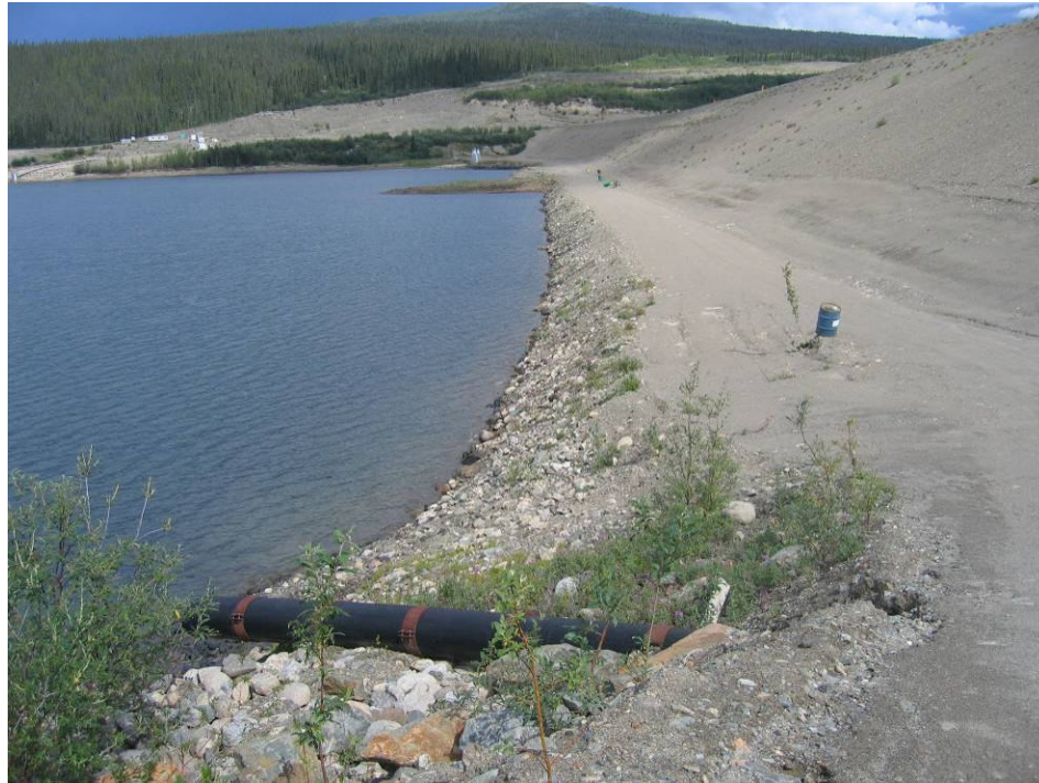
Photo II – 23 – Intermediate Dam – 1031m berm looking north. No erosion of berm at waterline, no riprap.
