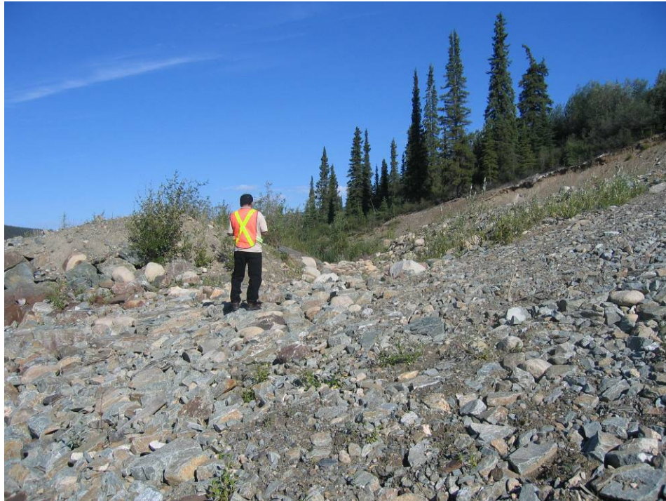
Photo II - 3 – Cross Valley Dam – Rockfill-lined Spillway.
