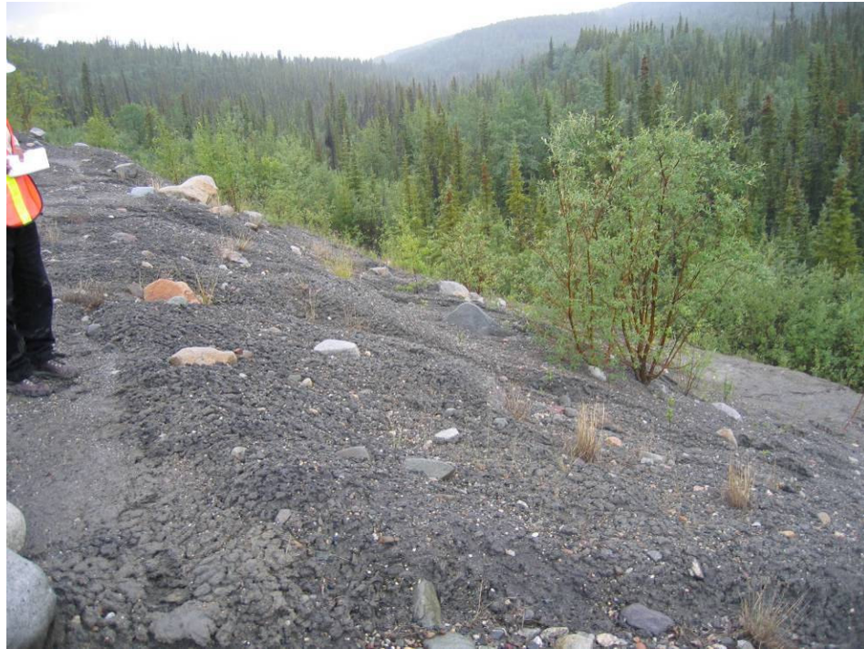
Photo II – 27 – Little Creek Dam – Downstream slope, note slumping.
