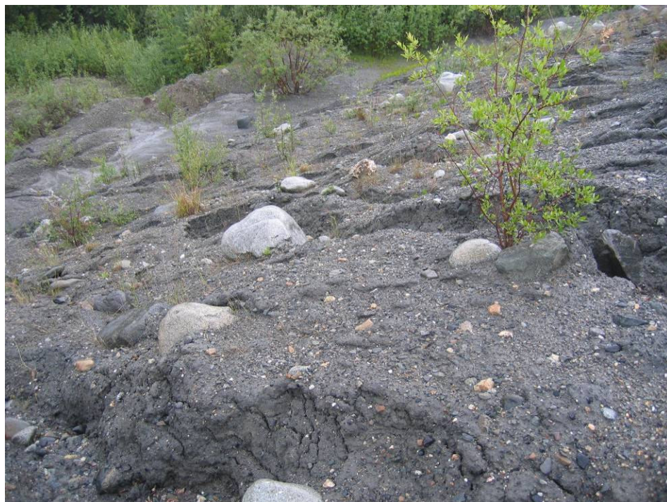
Photo II – 28 – Little Creek Dam – Slumping and erosion of slope at downstream toe.
