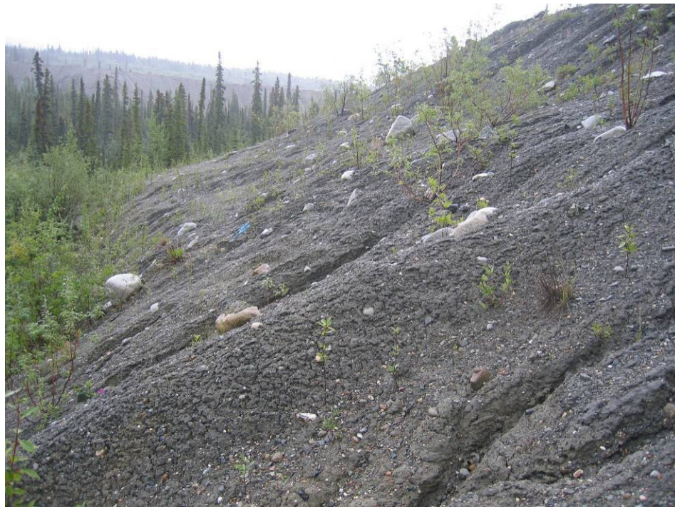
Photo II – 29 – Little Creek Dam – Slumping and erosion of downstream slope.
