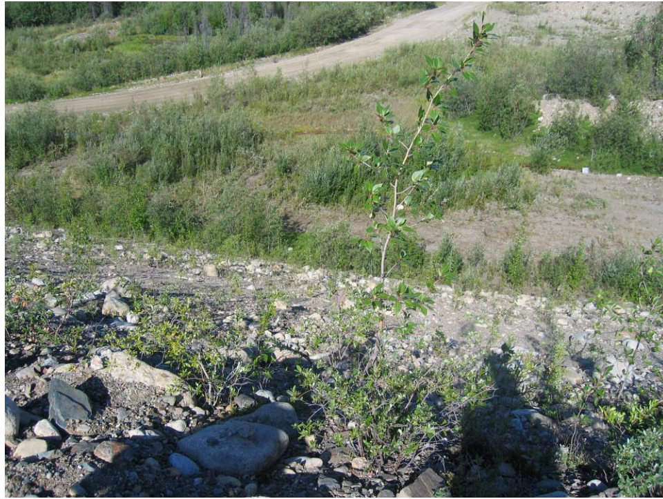
Photo II - 5 – Cross Valley Dam – Vegetation on Downstream slope near toe.
