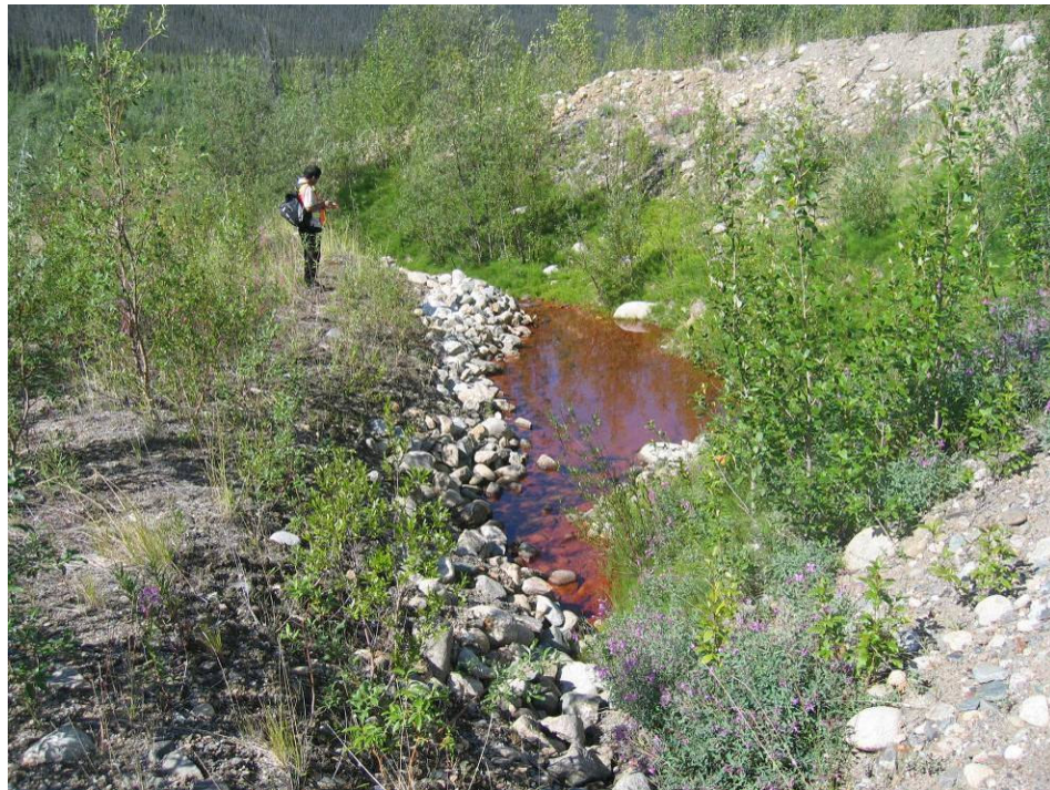
Photo II - 12 – Cross Valley Dam – Rockfill lining at toe of berm on right abutment.
