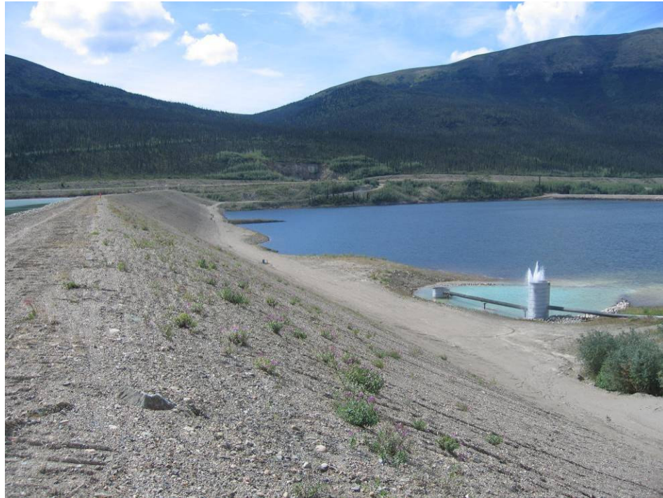
Photo II - 17 – Intermediate Dam – Outlet at toe at Intermediate Dam.
