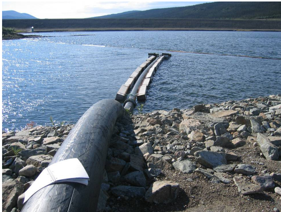
Photo II - 1 - Cross Valley Dam Floating Syphon Inlet.
