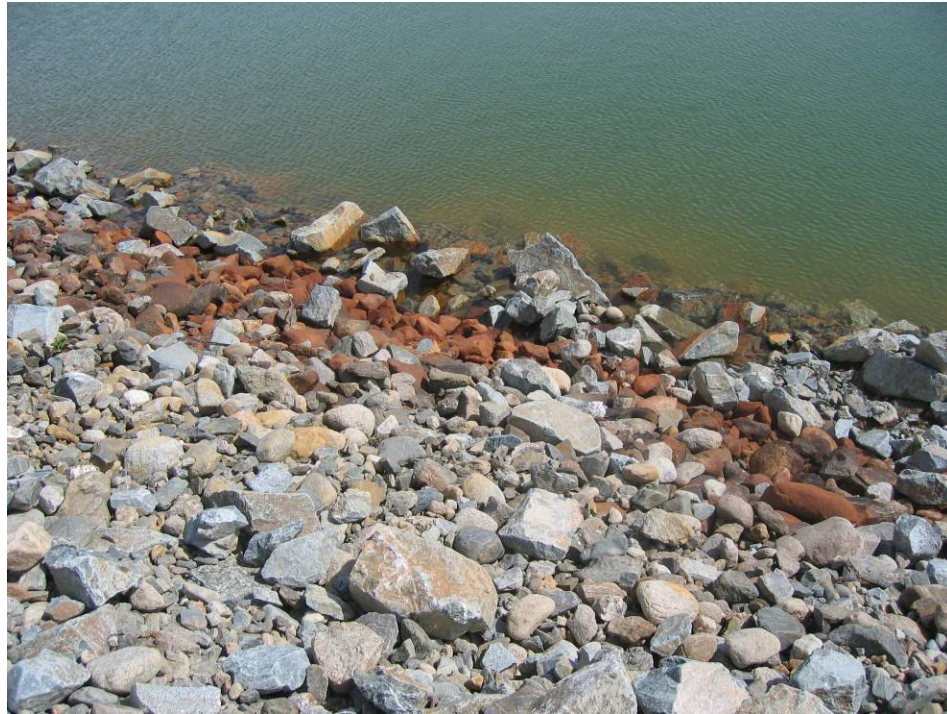
Photo II - 19 – Intermediate Dam – Riprap beaching.
