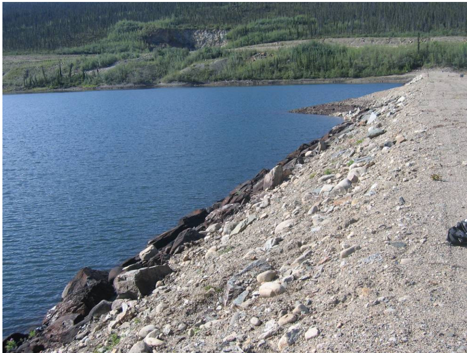
Photo II - 6 – Cross Valley Dam – Upstream slope without riprap above high water mark – looking south from right abutment.
