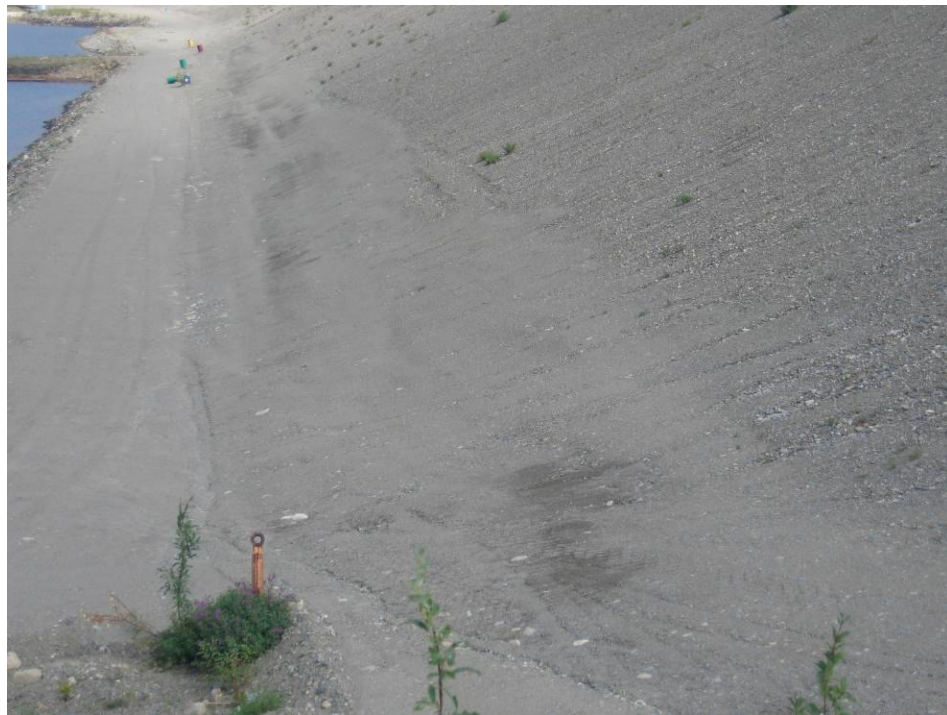
Photo II – 22 – Intermediate Dam – Downstream slope looking north along 1031m berm. Note drain exposure and minor erosion rills above drain.
