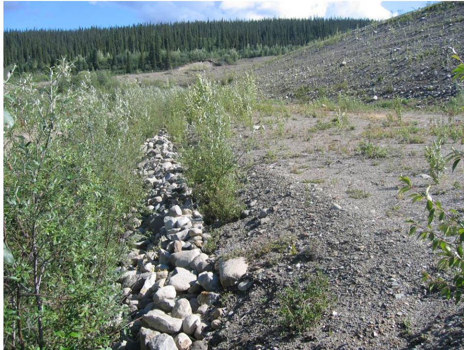
Photo II - 11 – Cross Valley Dam – Rockfill lining at toe of berm.
