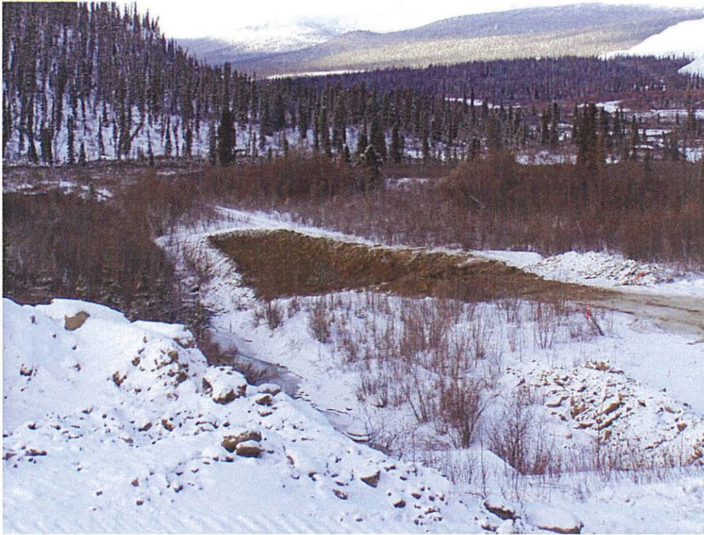
Photo 9 – Bulk excavation at the downstream limit of the breach. Fresh water channel in foreground, Nov. 23, 2003.
