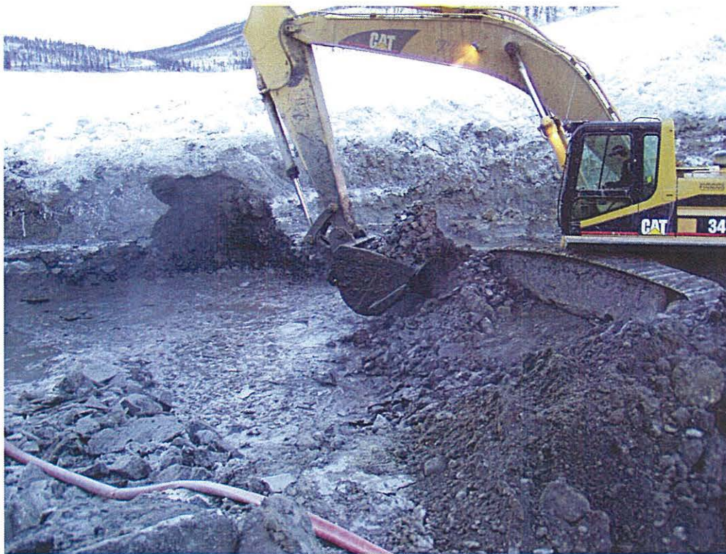
Photo 21 – Excavation for the placement of the inlet structure, Dec. 14, 2003.
