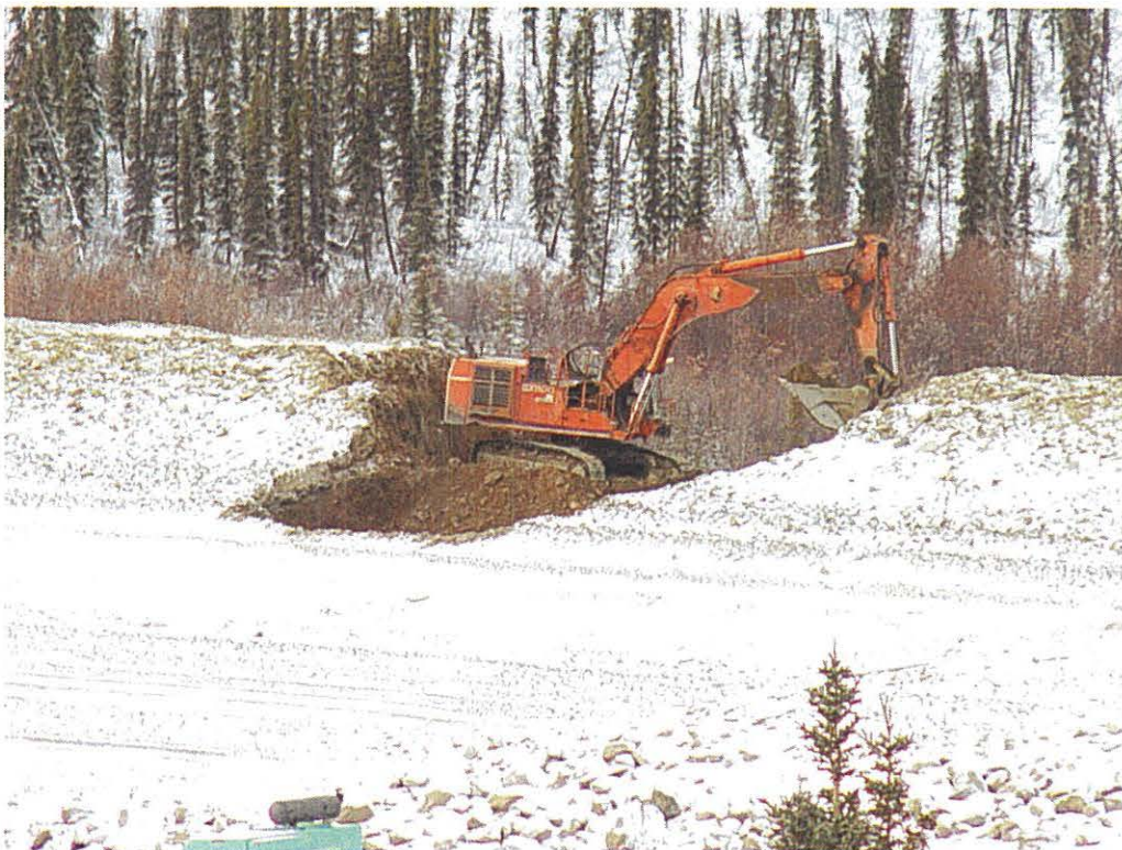
Photo 4 – Excavation of the breach through the upstream face, Nov.11, 2003.
