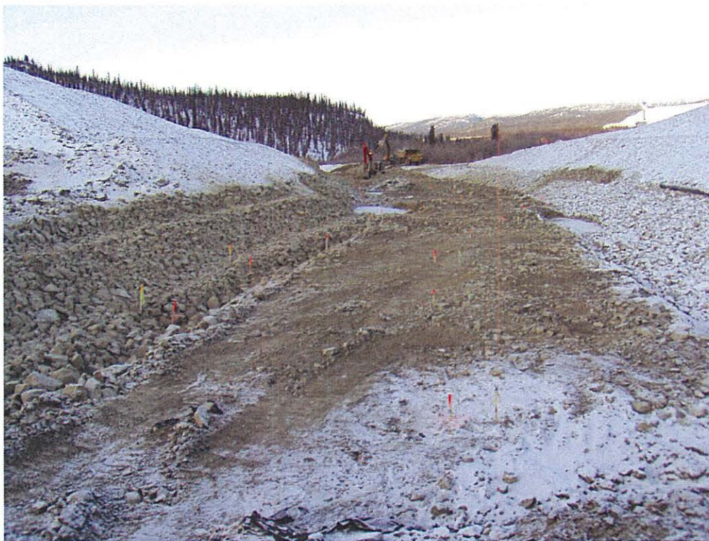
Photo 15 – View of floodplain, erosion protection riprap installed, prior to channel excavation, Dec. 4, 2003.
