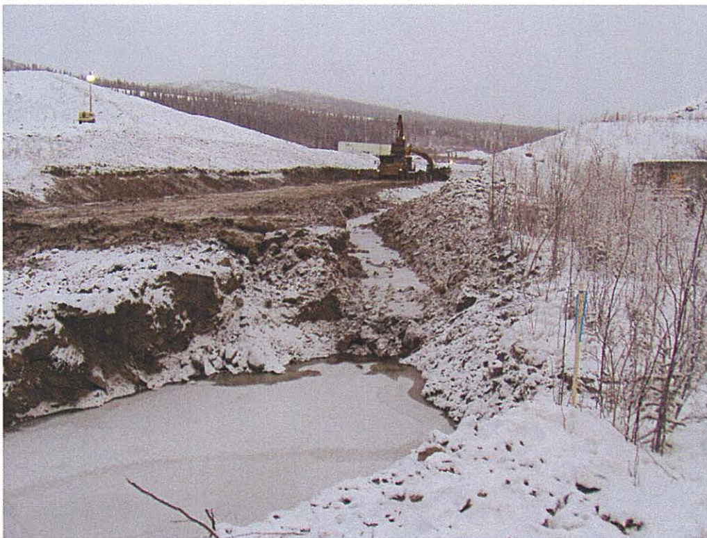
Photo 12 – Excavation for erosion protection, left side of floodplain, Nov. 29, 2003.
