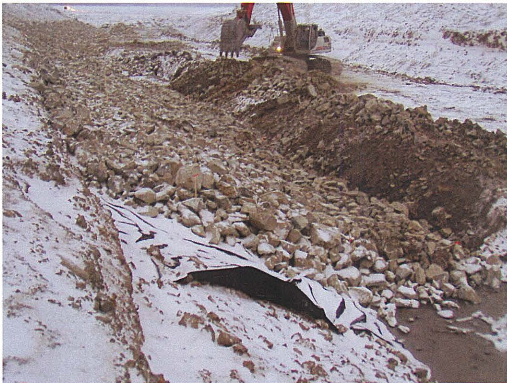
Photo 14 - Installation of rip rap within erosion protection, Dec. 2, 2003.
