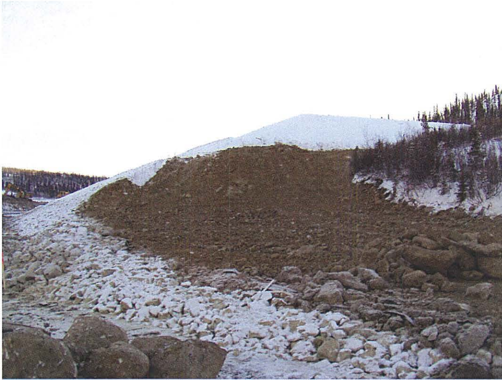
Photo 19 – Valve house removed and fill placed in fresh water channel, Dec. 11, 2003.
