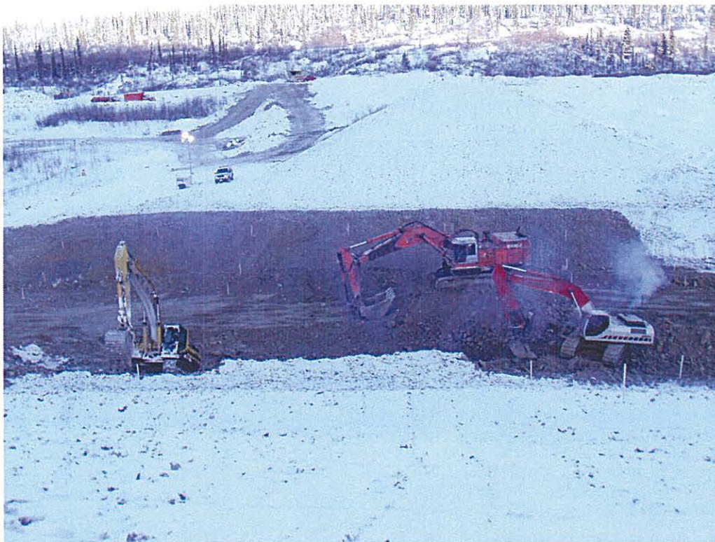
Photo 10 – Northward view of final excavation to floodplain level and slope trimming, Nov. 25, 2003.
