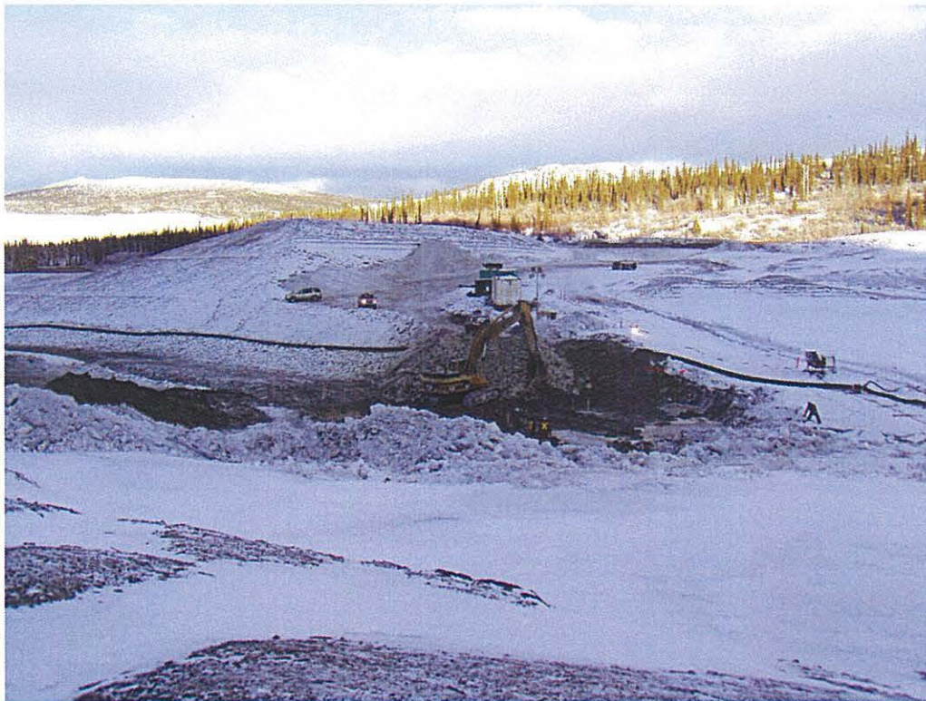
Photo 20 – Excavation of final portion of the channel at the location of the cofferdam, Dec. 13, 2003.
