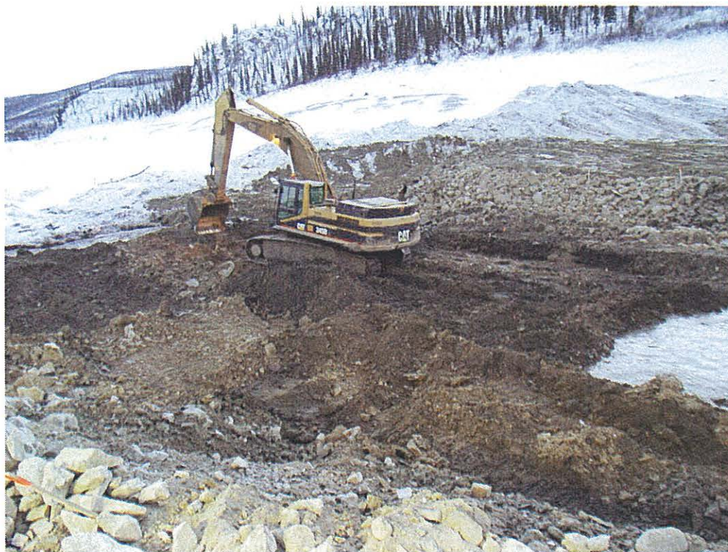
Photo 22 – Excavation for the downstream apron of the inlet structure, Dec 15, 2003.
