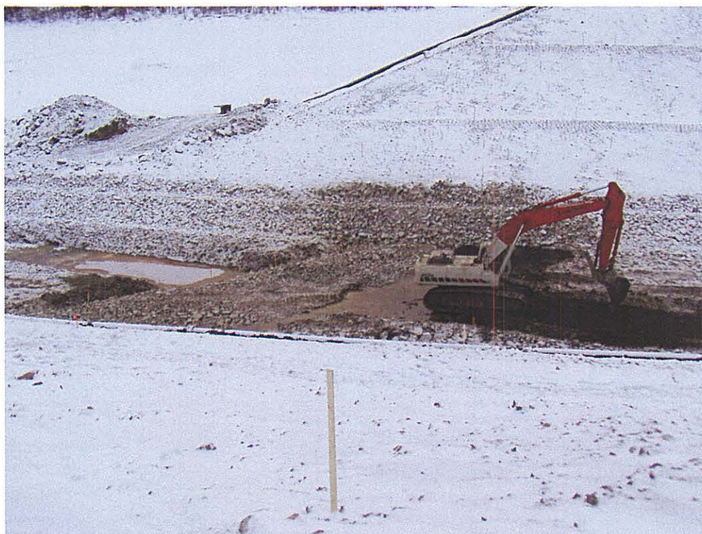
Photo 16 – Completion of the rip rap surface at riffle 1 (southward view), Dec. 7, 2003.
