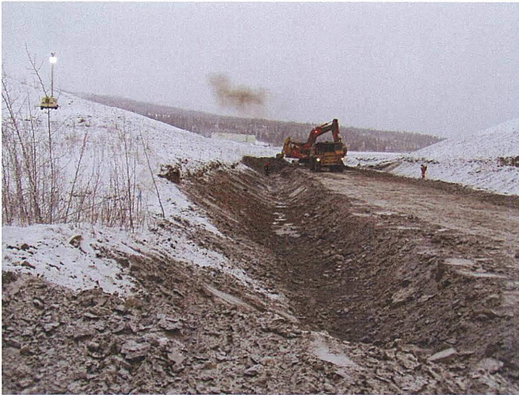
Photo 11 – Excavation for erosion protection, on right side of floodplain, Nov. 29, 2003.
