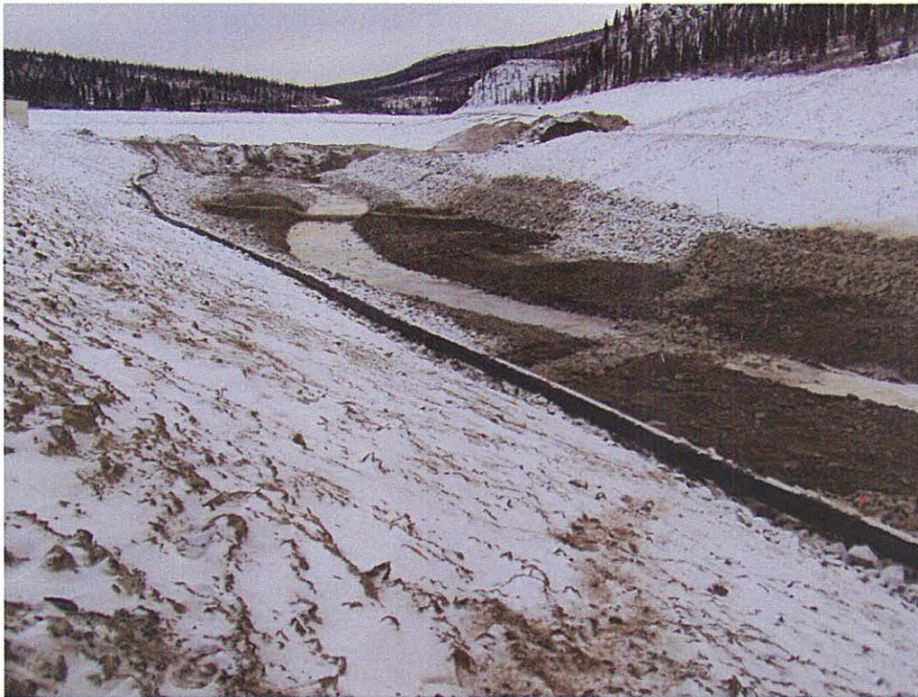
Photo 17 – View of upstream portion of completed channel, erosion protection and riffles 1 & 2, Dec. 9, 2003.
