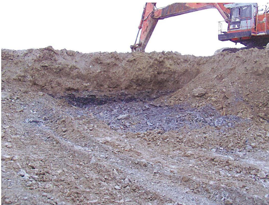
Photo 7 – Exposure of the 1969 berm, at downstream toe. The lighter grey material was taken to the PAG spoil area, Nov. 18, 2003.
