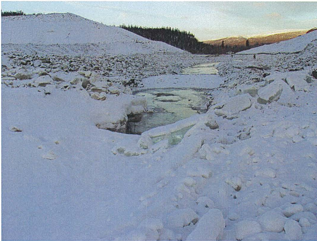
Photo 27 – View looking downstream at the completed breach. Photo taken from upstream of the inlet structure, Dec. 16, 2003.
