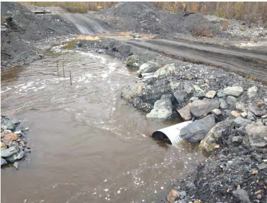
2.4 m 3 /s at 5:00pm after pumps turned on. Pumps account for ~1.1 m 3 /s.
