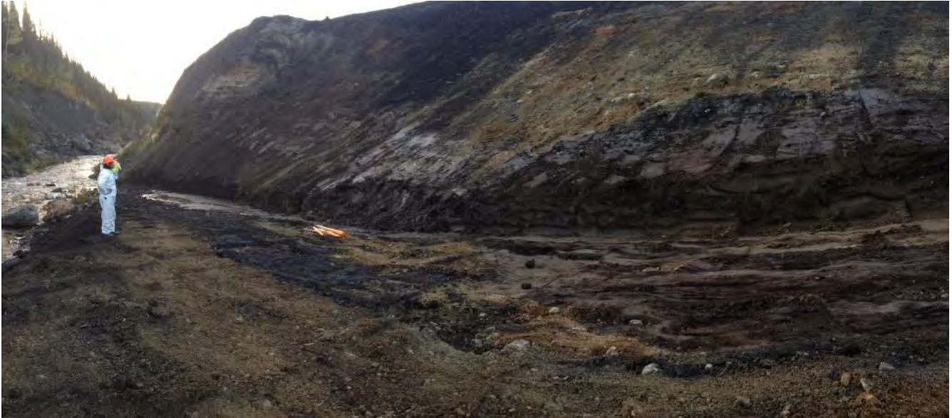
Looking east: Permafrost layer along toe of excavated slope (dark brown area). Bottom 2-4 meters approximately.
