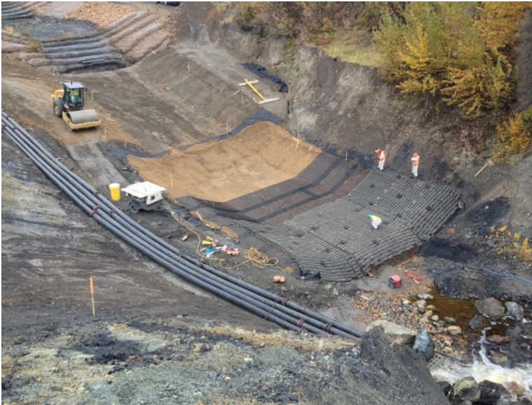
Photo M Placing Geosynthetics, Gravel Base, and Armorflex Mats (September 14, 2015, looking northwest)
