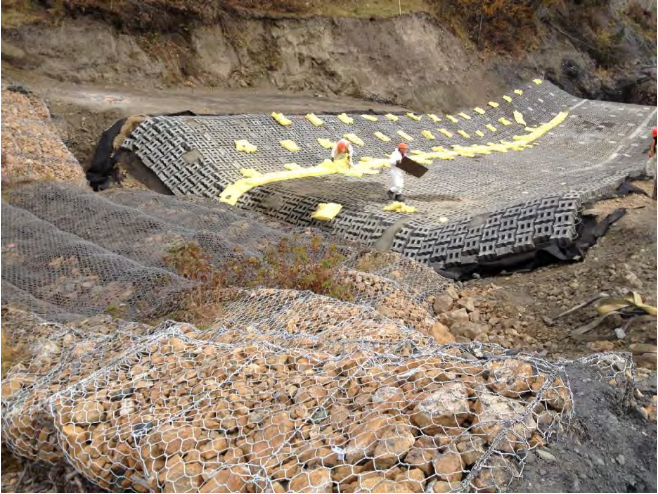
Looking northeast: transition from gabions to Armorflex
