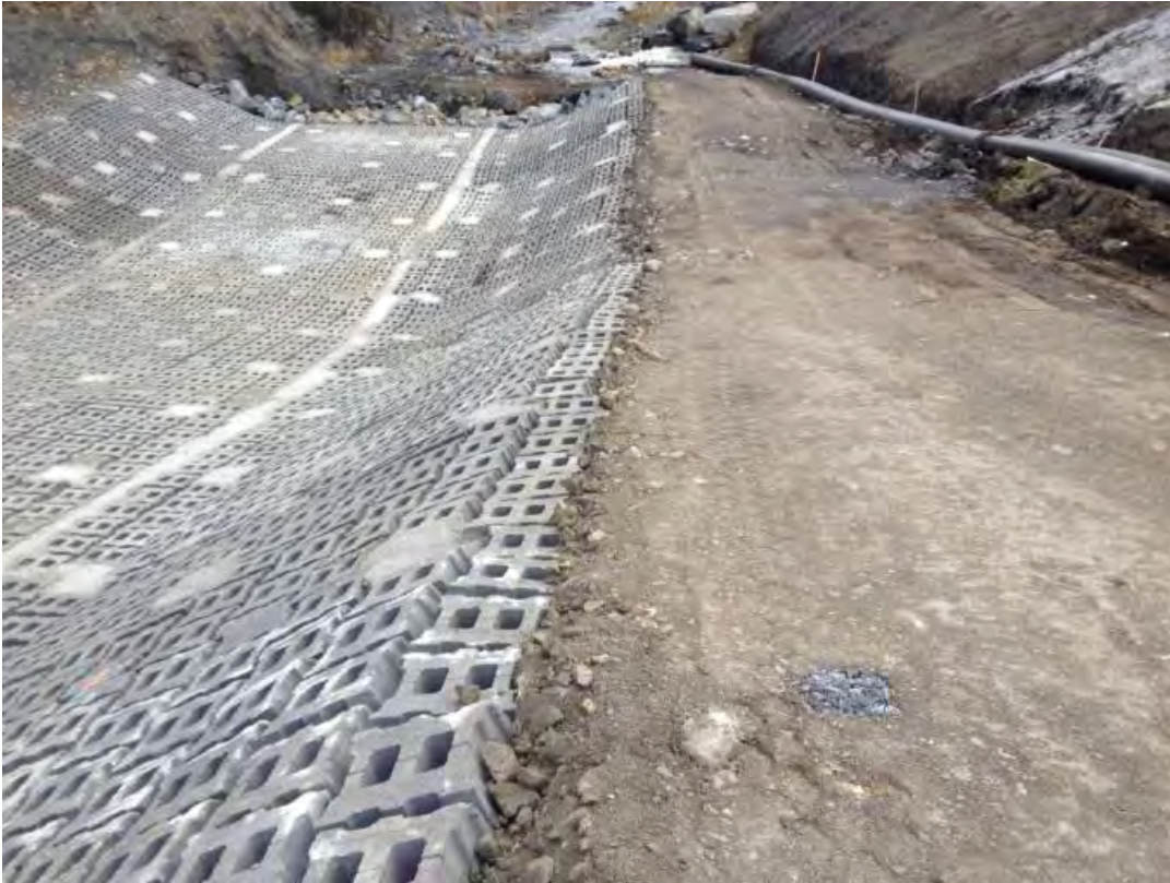
Looking east: Most of south side anchor trench looks ok, but some areas are below top of armorflex or not covering geogrid.
