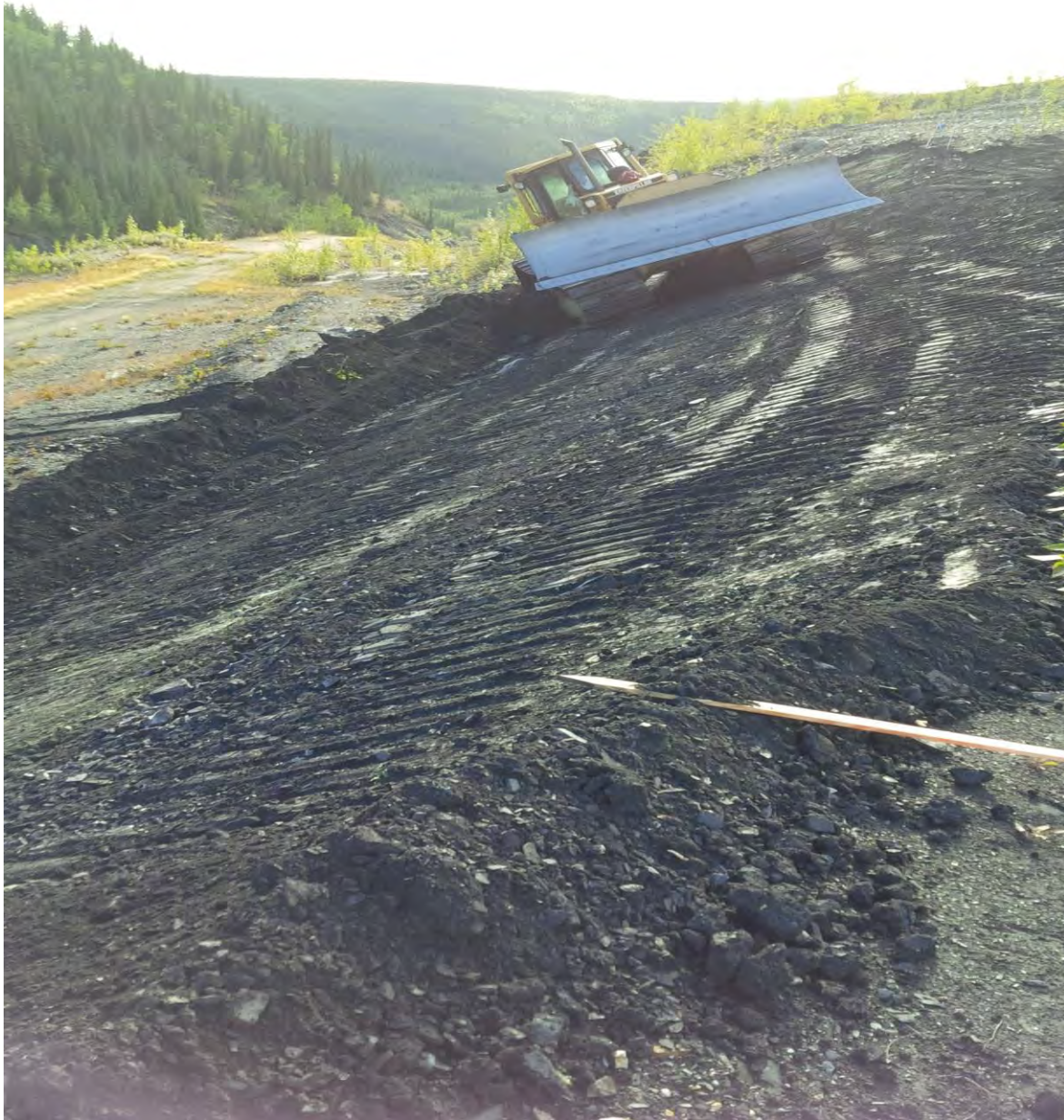
Looking East: the D6M dozer cutting the slope
