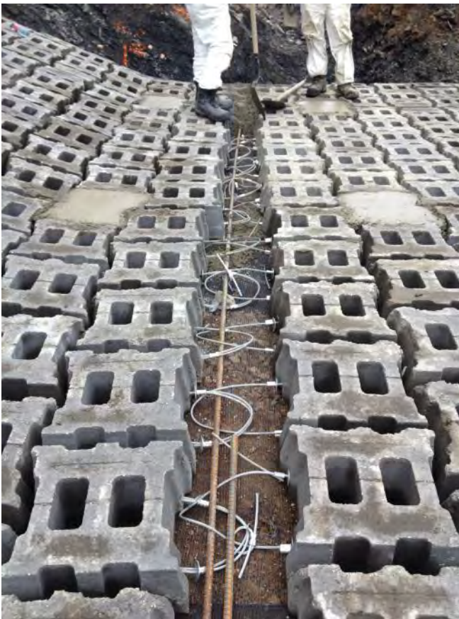
Looking east: Loose cables to be tucked in, should not stick out of grouted trench
