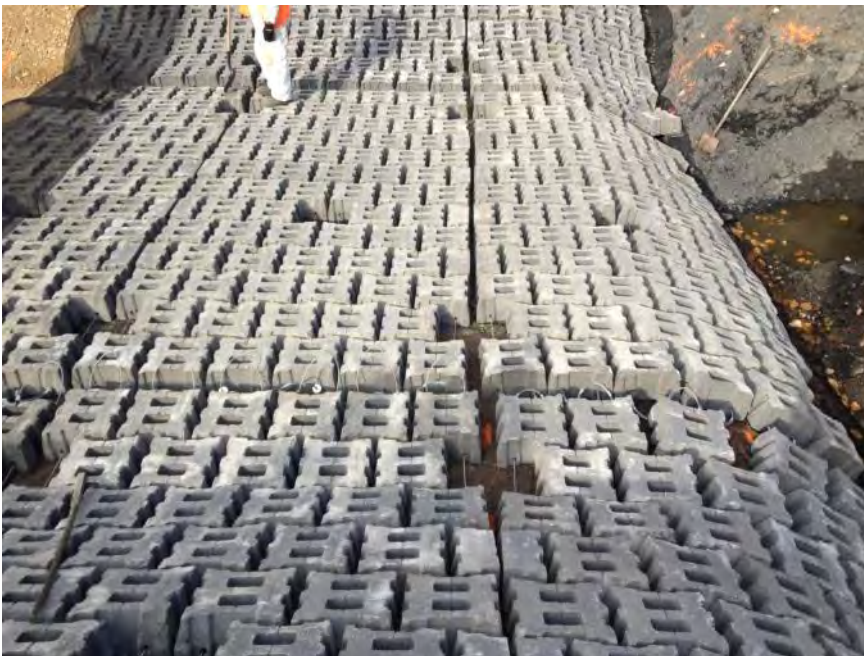
Looking north: Targeting less than 5cm gap between adjacent mats along channel. Will grout gaps greater than 5cm.
