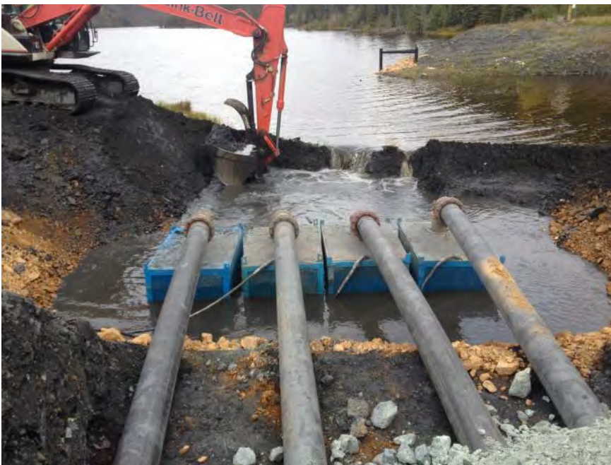
Looking west: Pump sump being connected to lake.
