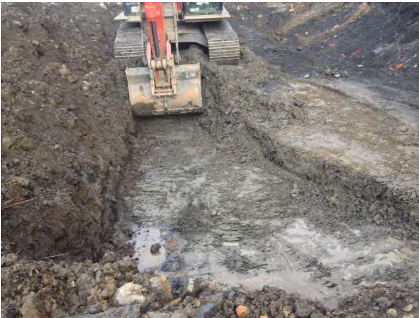
Looking west: Subexcavation on RHS of channel between station 0+50 and 0+65. 0.5 m deep
