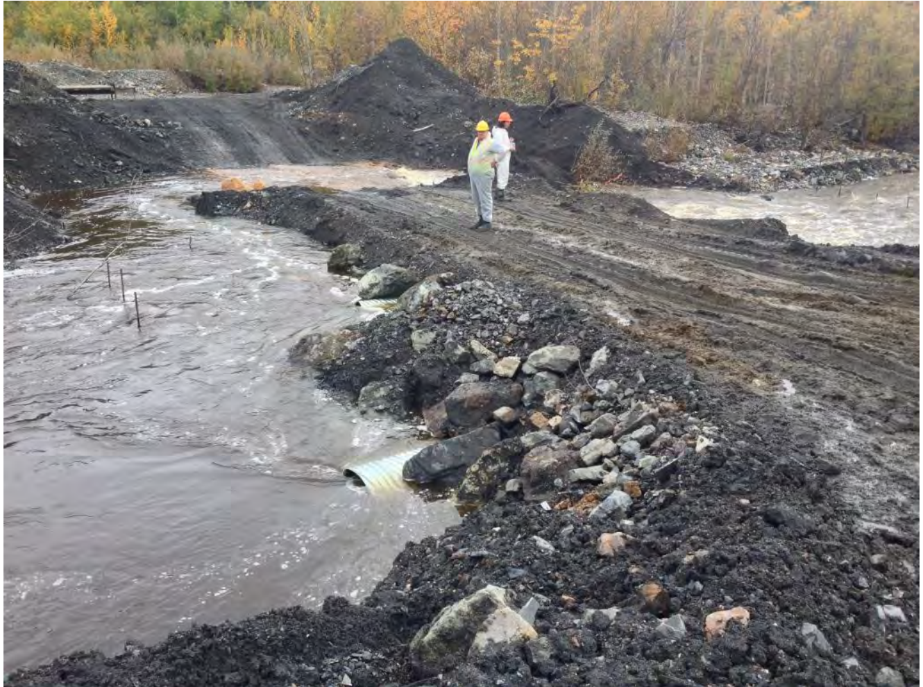
Looking North: Fording with one 1000mm culvert (closest), four 600mm culverts and a fording (farthest). Approx. 3.4 m 3 /s
