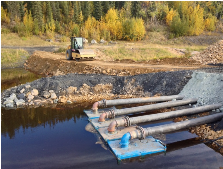
Photo E Pump Intake and Dam at Hudgeon Lake Outlet (September 3, 2015, looking northeast)
