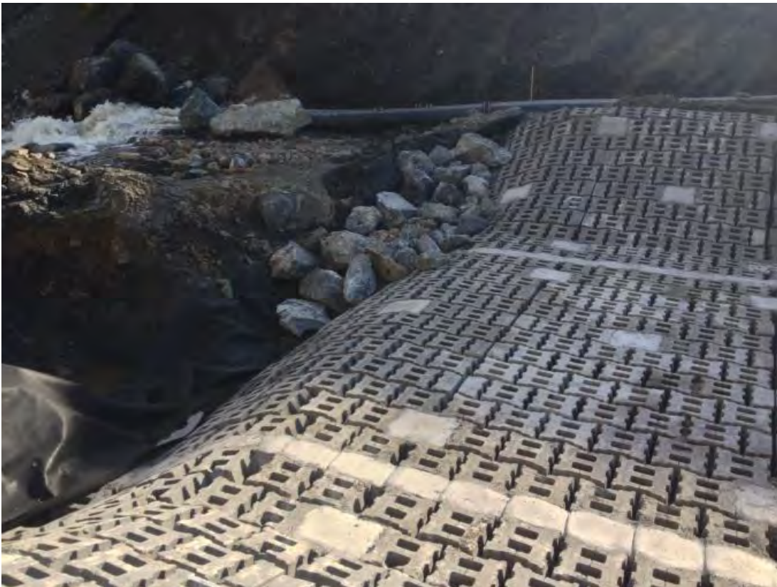
Filled half of downstream anchor trench with riprap
