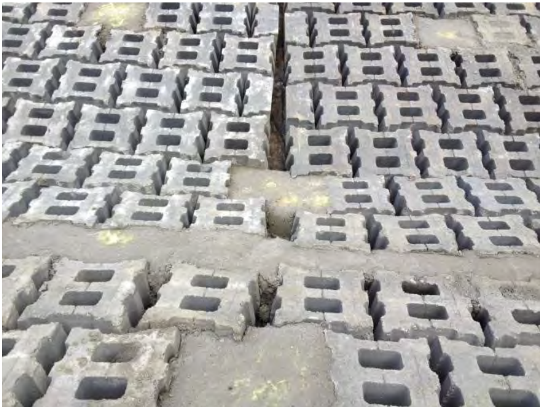
> 5 cm gap between mats to be filled with grout
