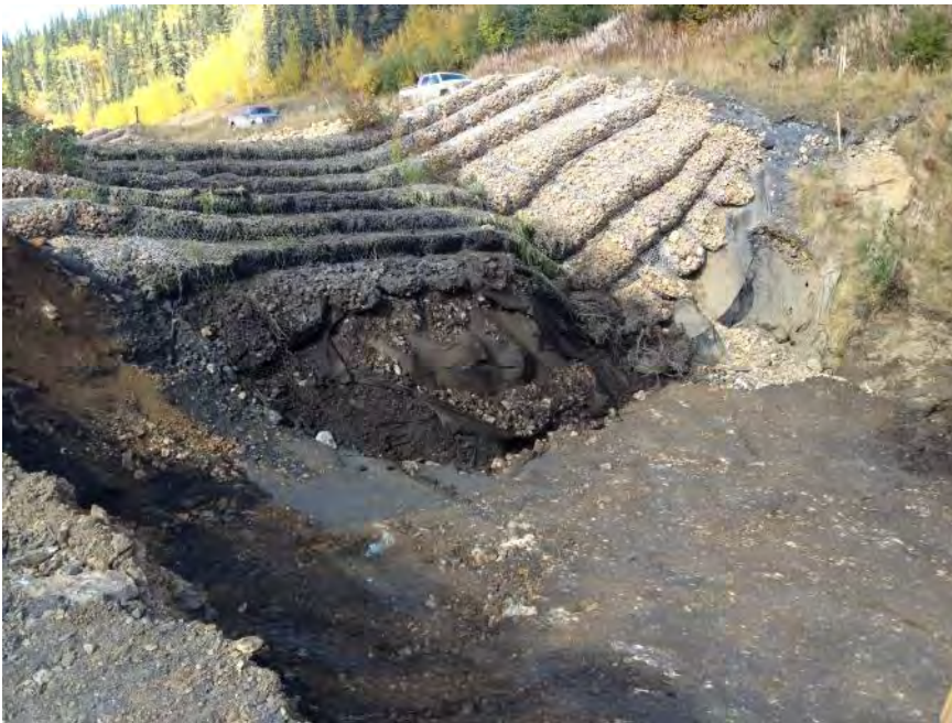
Looking northwest: Damaged gabion baskets removed. Top of Armorflex will tie into first level of intact gabions (second level shown).
