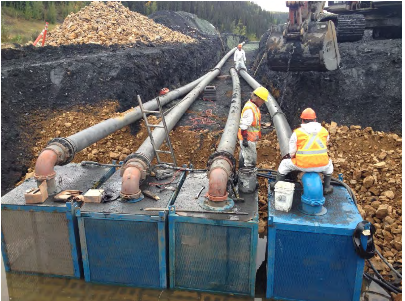
Looking East: Pumping diversion, four 10" pumps connected to 12" hdpe. Sitting on old armorflex mat
