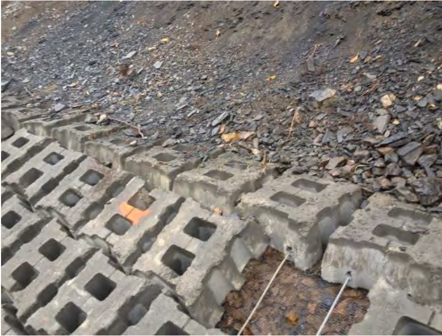
Looking northwest: Filling north side of channel along 1:1 cut to top of Armorflex blocks
