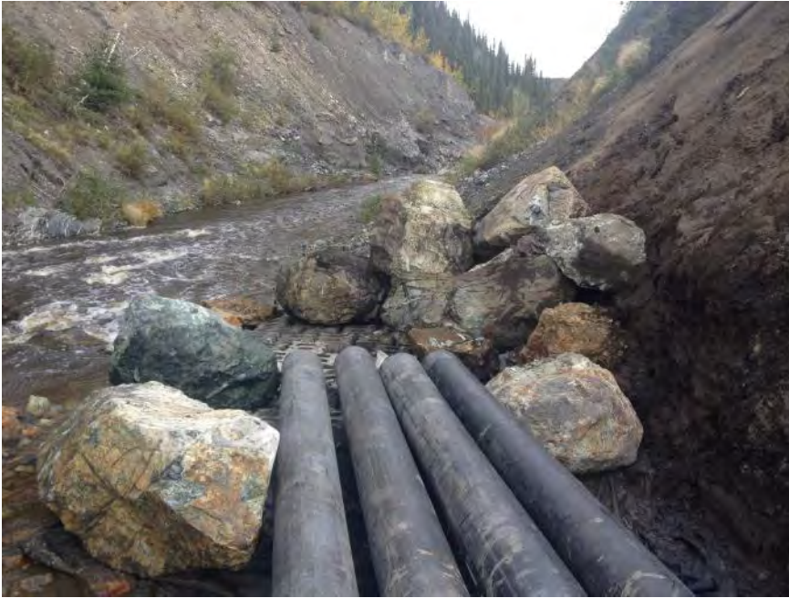
Looking east: Pipe outlet with armorflex and riprap
