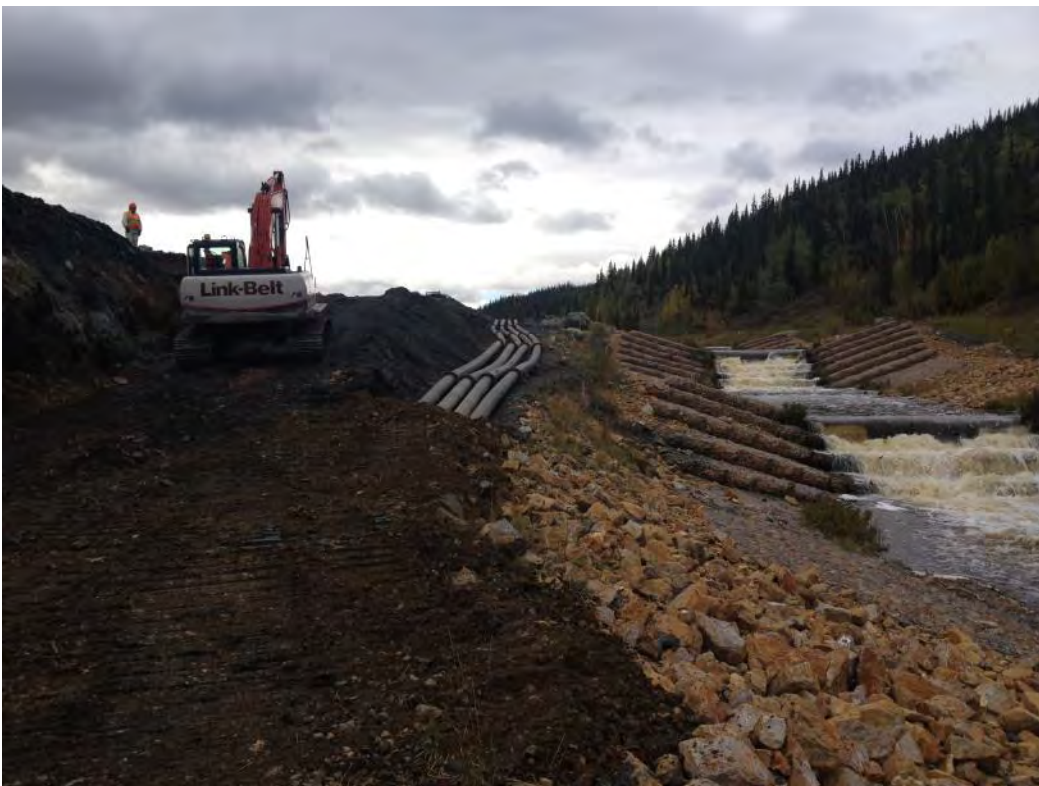
Looking west: 4x 165 meters of 12: HDPE pipe placed for diversion.
