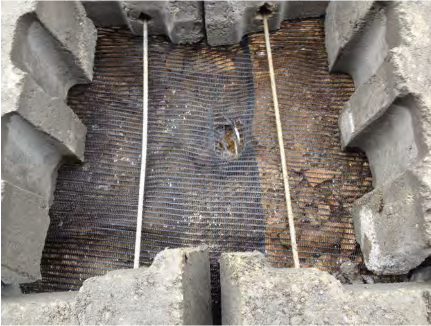
End of duckbill anchor (before setting)
