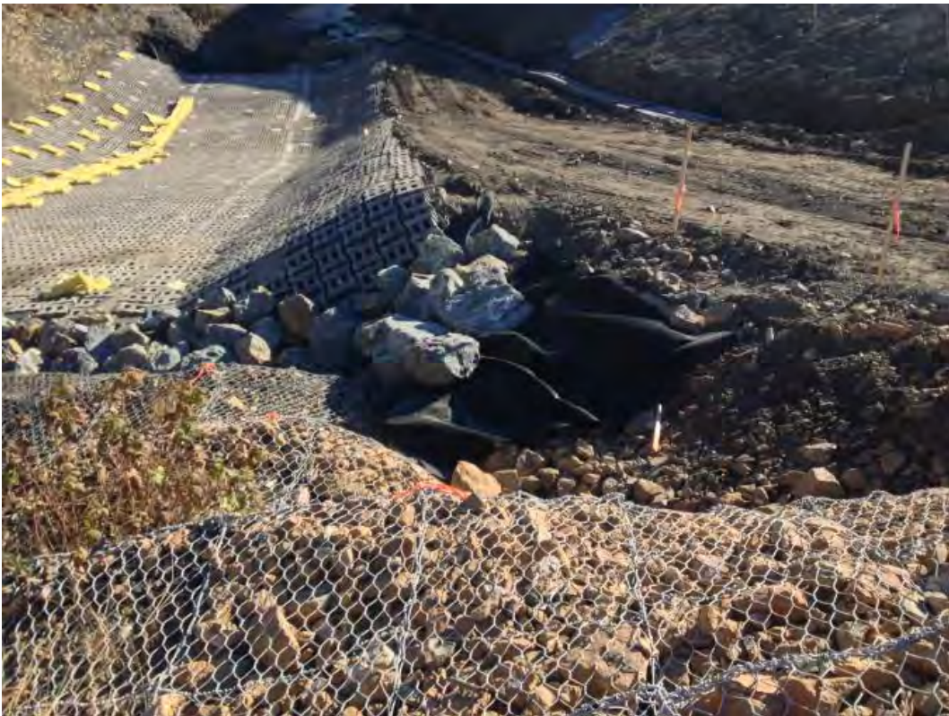
Looking east: South side of gabion-to-armorflex transition. Road to be built up to flagging on lath. Riprap to be placed out to flagging tied to gabions
