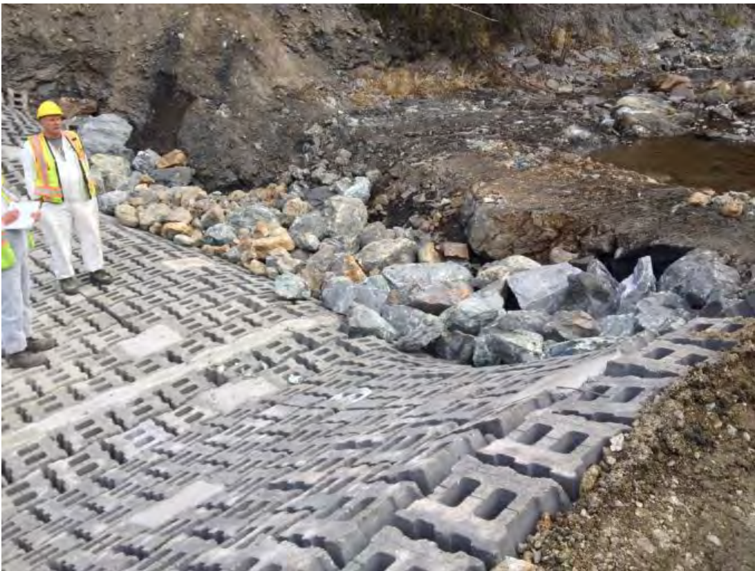
Looking northeast: Riprap at outlet (berm located behind riprap)
