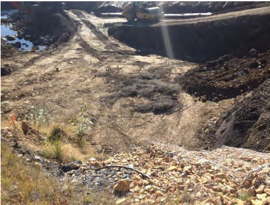
Looking southeast: Burying damaged gabion baskets in middle of channel infill.
