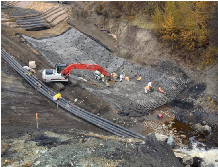
Photo N Mixing and Placing Grout (September 17, 2015, looking northwest)
