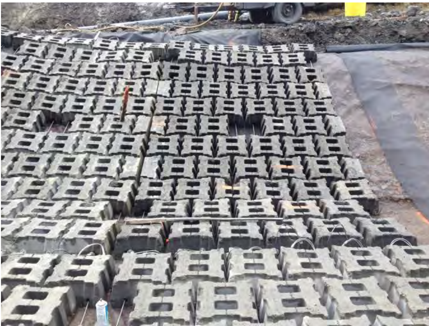
Looking south: 5 th mat from end is typical of generally poor concrete. 3 blocks cracked during placement.
