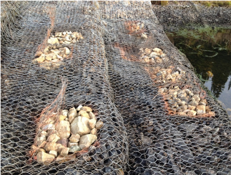
Photo T Cutting and Filling Gabion Baskets with Rock (September 11, 2015, looking north at DS3)
