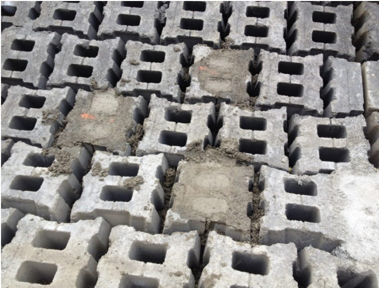
Photo O Broken concrete blocks grouted in place (September 21, 2015)
