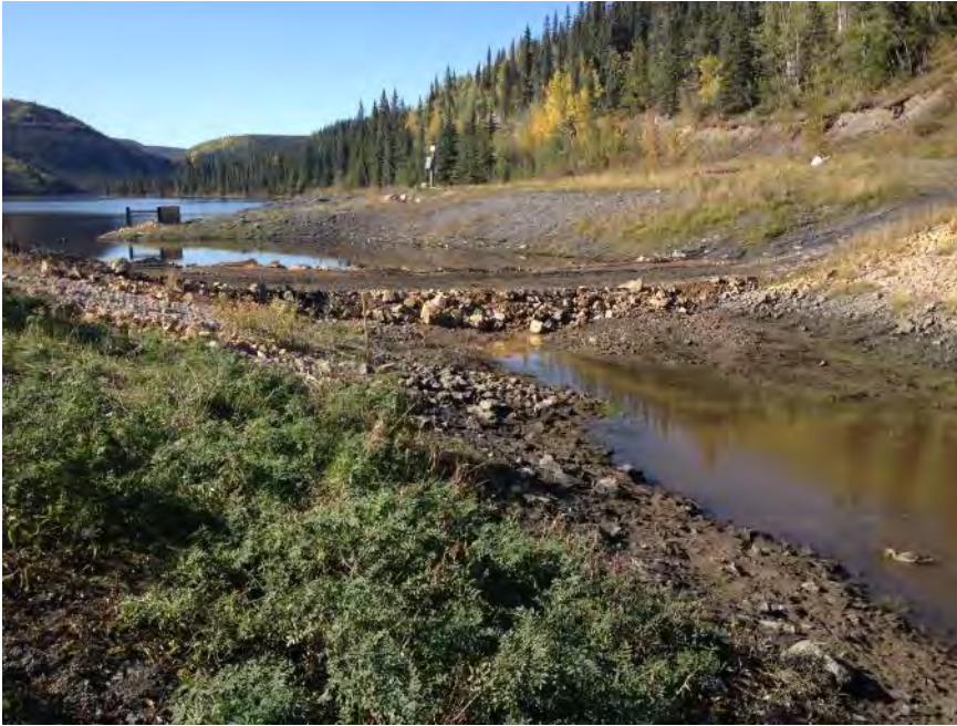
Looking west: Coffor dam. ~5 m wide. Not constructed to full height.
