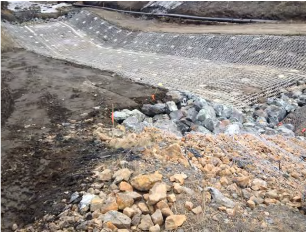
Looking southeast: North anchor trench completed. Some orange rocky fill to be brought in to build up north access road to orange flagging on the lath and compacted with roller compactor.
