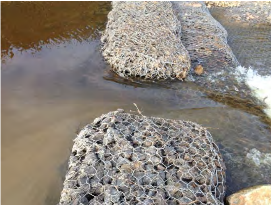
Looking north: Minimum 200 L/s achieve as measured at notch in DS1. Weir flow: 0.8m wide, ~0.35 m deep.
