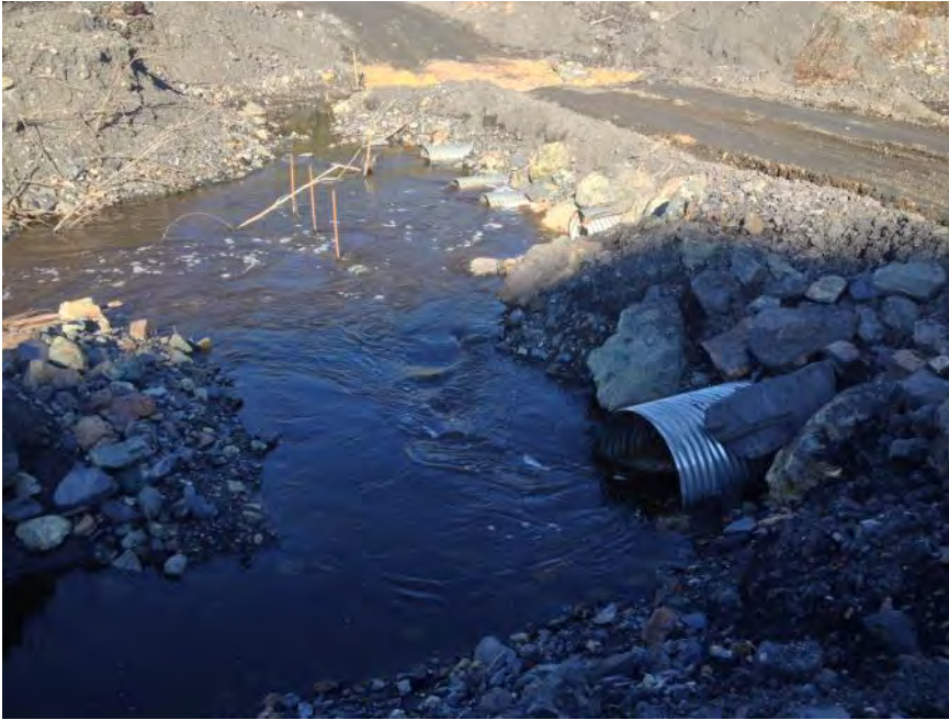
1.1 m 3 /s at 5:30pm. Cofferdam in place. Flow around construction area is completely diverted
