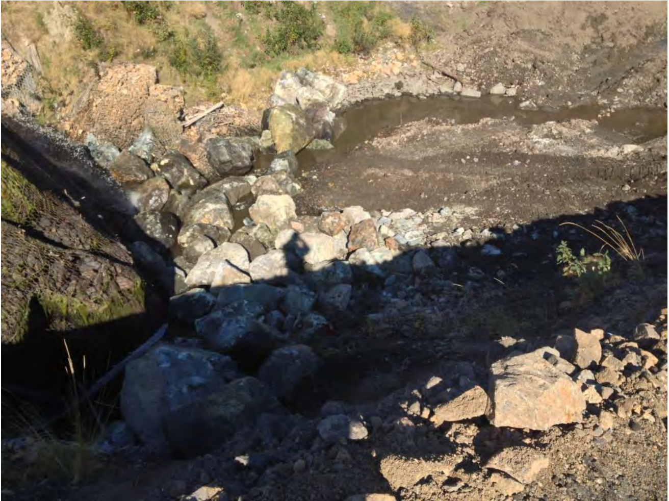
Looking northeast: Subgrade prior to fill. Rocks collected to deepest fill, beneath gabions.
