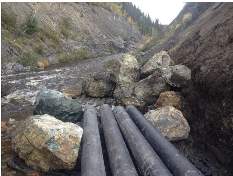
Photo F Diversion Pipe Discharge, Erosion Protection (September 1, 2015, looking east)
