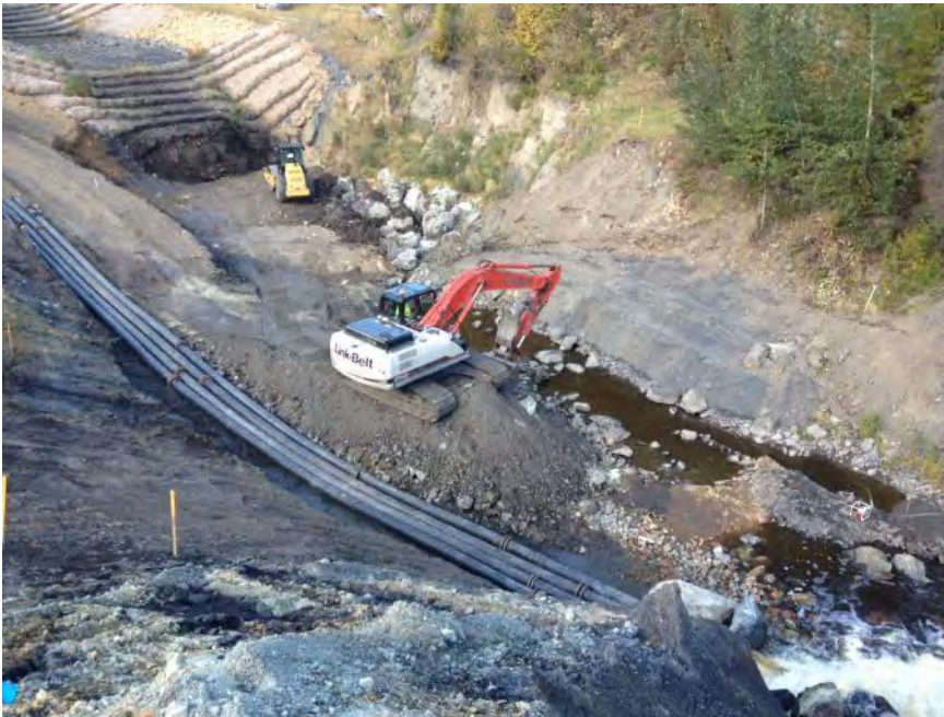
Looking northwest: Instream work area at 4pm – removing some poorly compacted fill.
