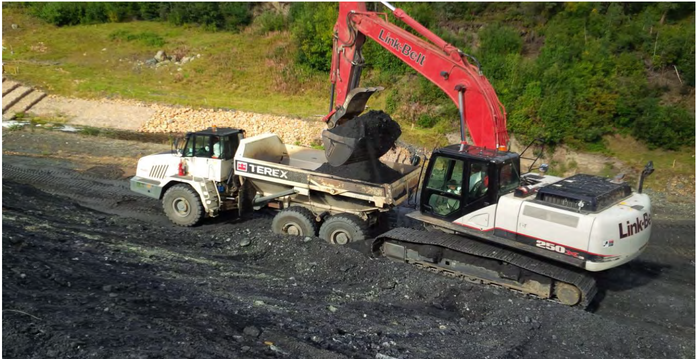
Looking North: the excavated waste rock is taken away to the dump area
