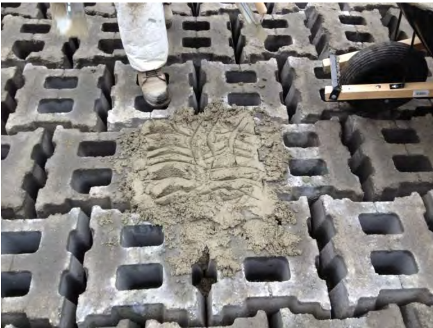
Filling void with grout using shovel
