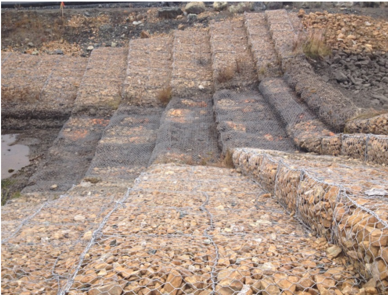
Photo U Finished Gabion Basket Repair (September 20, 2015, looking south at DS2)
