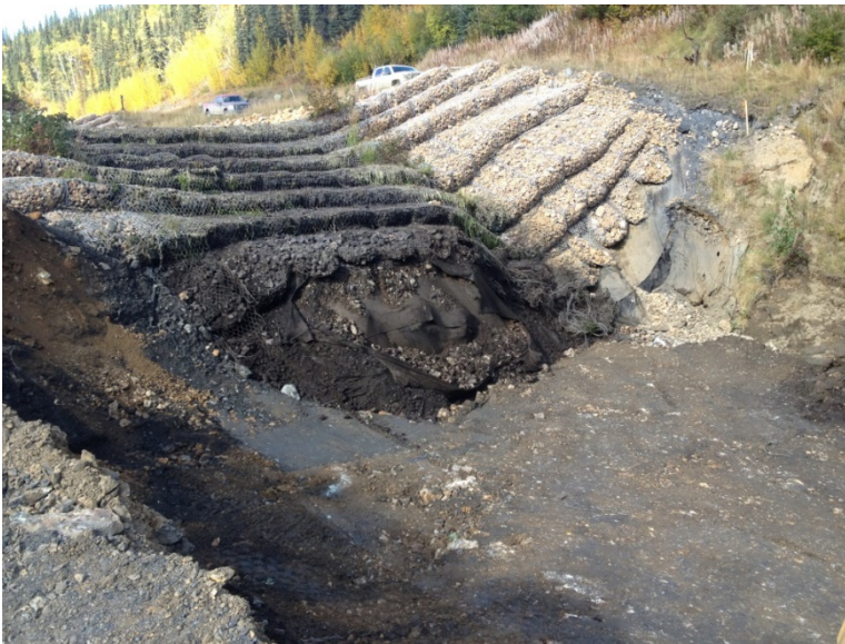
Photo J DS4 after Removing Damaged Gabion Baskets (September 5, 2015, looking northwest)
