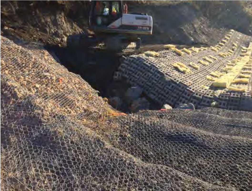
Looking east: North side of gabion-to-armorflex transition to be filled with riprap
