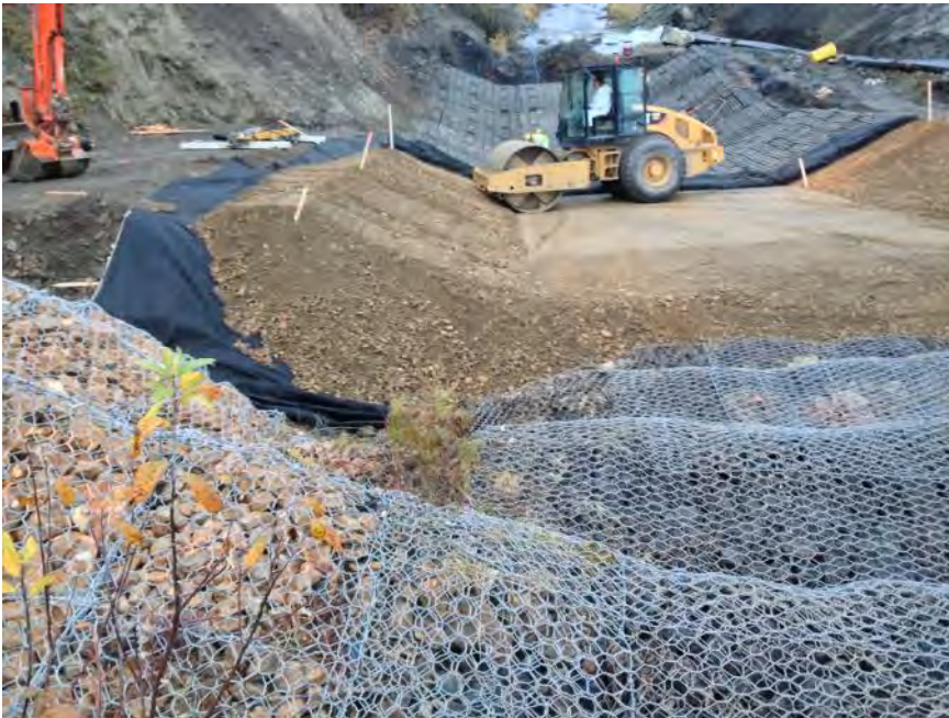
Looking east: Transition from Gabions to Armorflex
