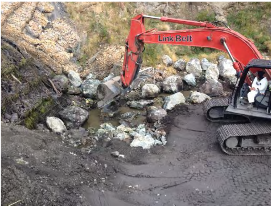
Looking north: Spacing out boulders to minimize voids in fill, 11am.
