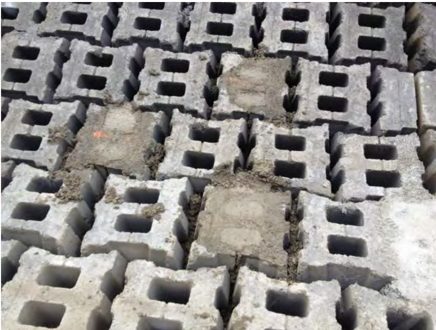
Repair of broken Armorflex blocks – fill both voids with grout
