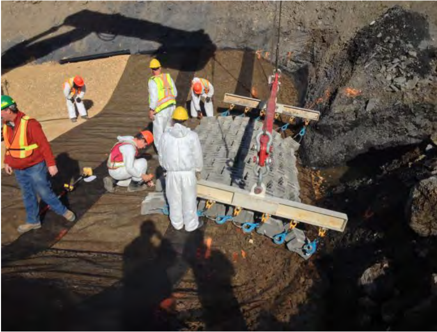
Looking north: Placement of first Armorflex mat, ensuring min. 2 blocks buried.
