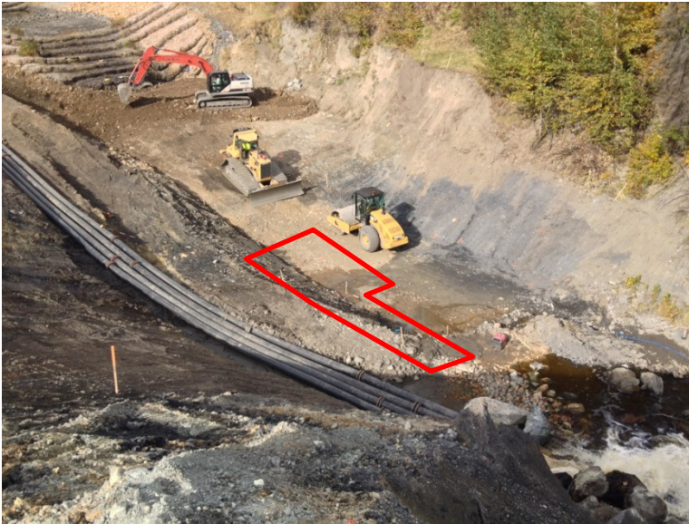
Photo L Placing and Compacting Fill - Red line shows approximate extent of subgrade excavation. (September 9, 2015, looking northwest)
