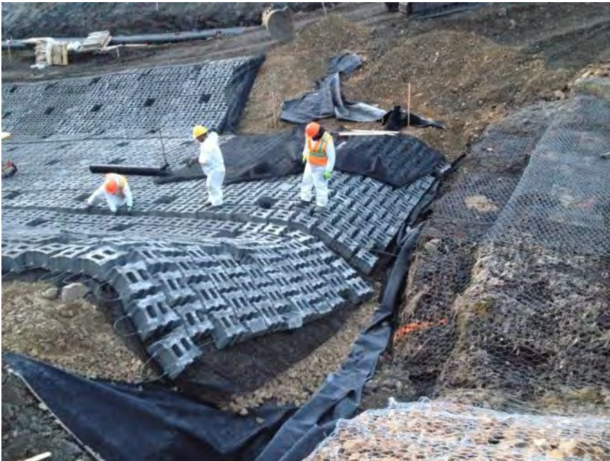
Looking south: upstream anchor trench at 7am, following day
