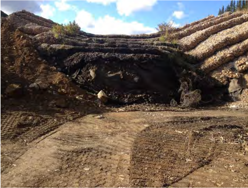
Looking west: 2 nd lift placed in channel.
