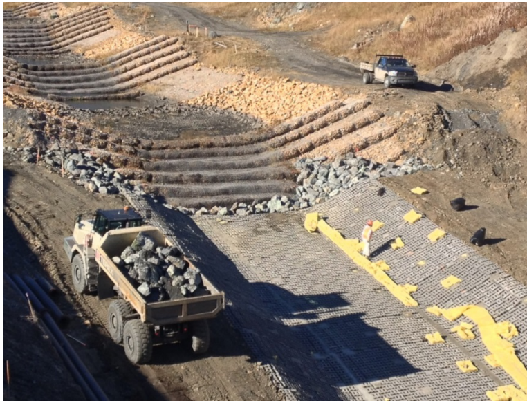
Photo P Placing Large Diameter Rock (September 22, 2015, looking northwest)
