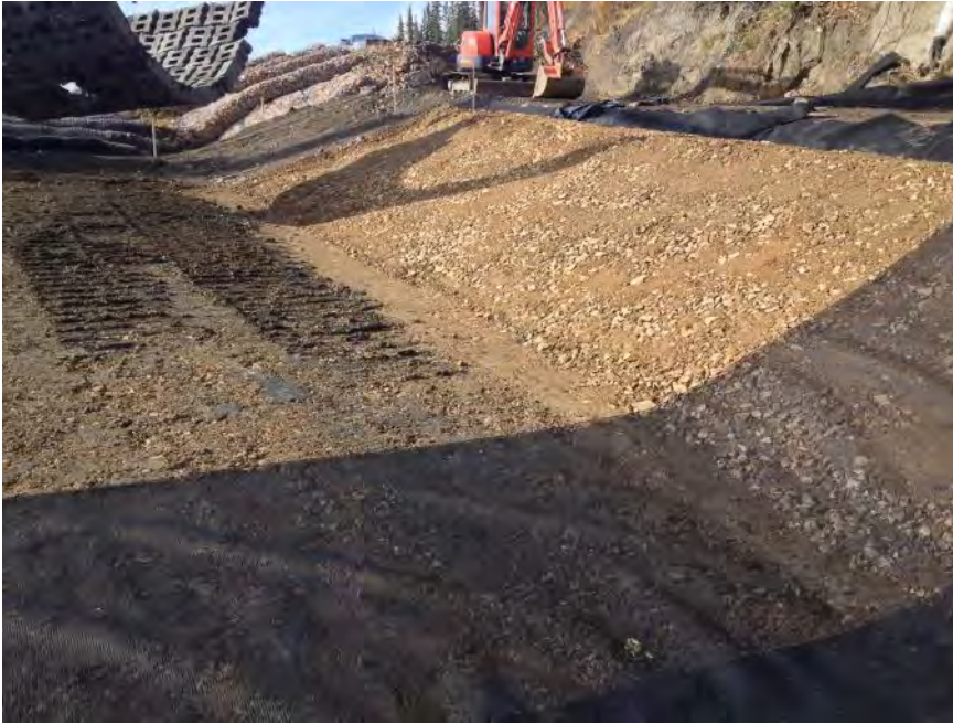
Looking northwest – Typical base for Armorflex. Generally smooth but difficult to have all blocks sit flat.
