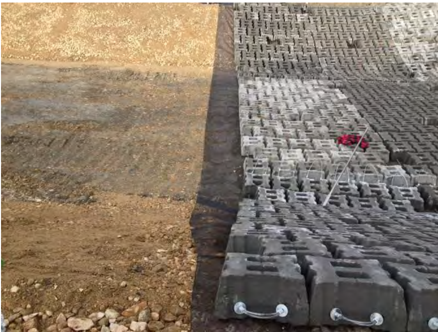
Looking north – 9 th mat from end. Side mats are starting to get slightly rotated. Will try to correct with next row of mats.
