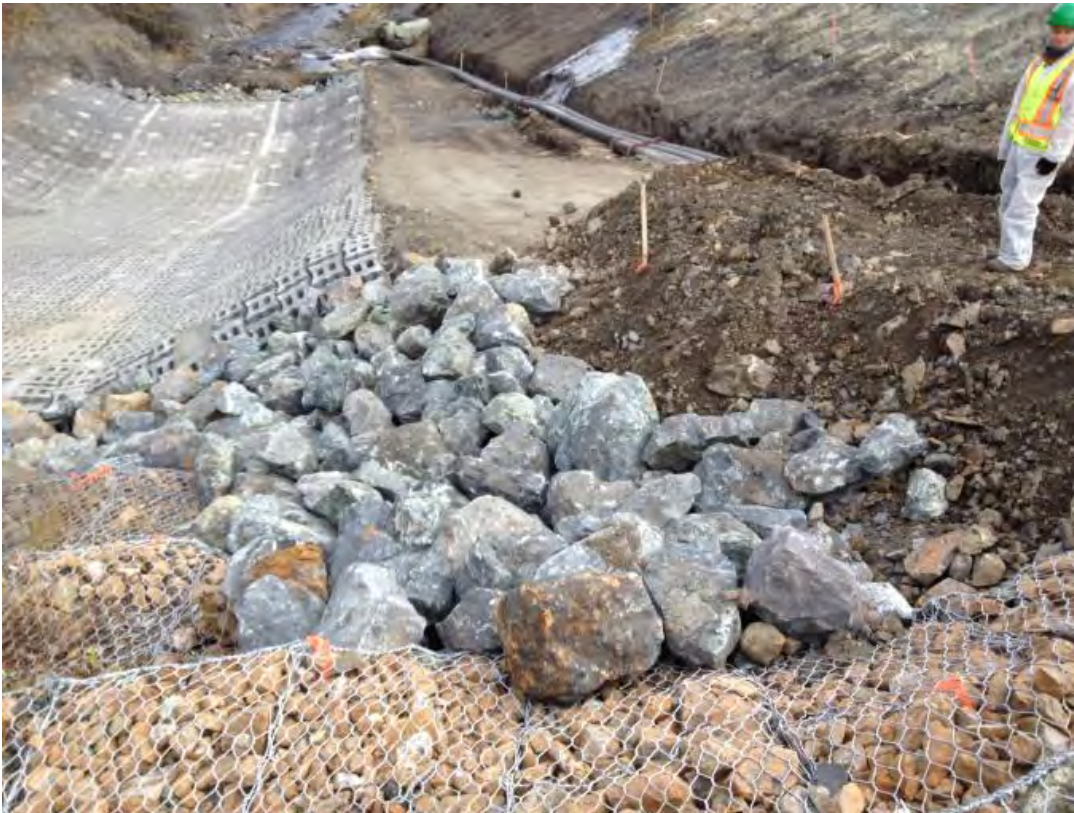
Looking east: South access road to be built up to orange flagging on lath with rocky fill and compacted with roller compactor.
