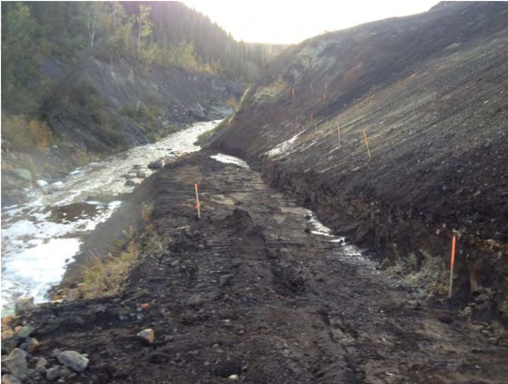
Looking east: Top of permafrost region marked with survey stakes.
