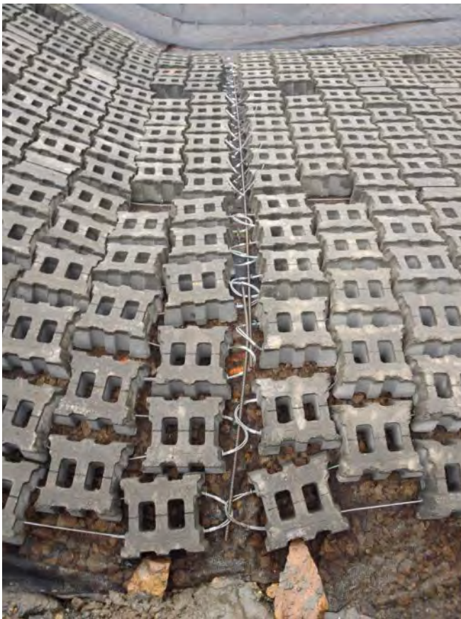
Looking west: 20m rebar between Armorflex mats
