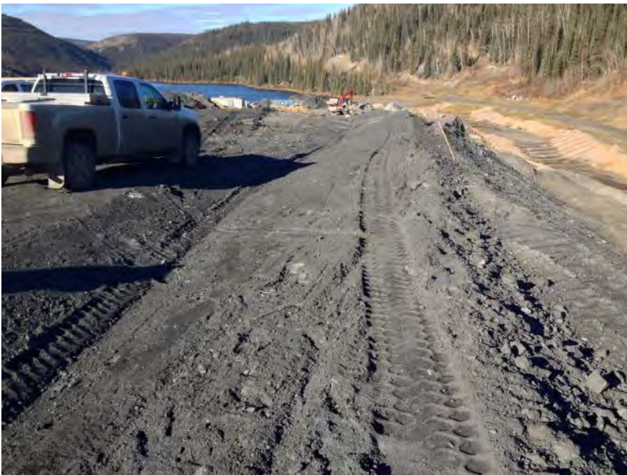
Looking west: Drainage ditch at top of 2:1 slope
