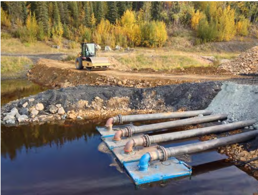
Looking north: pumps and finished coffer dam at lake outlet.
