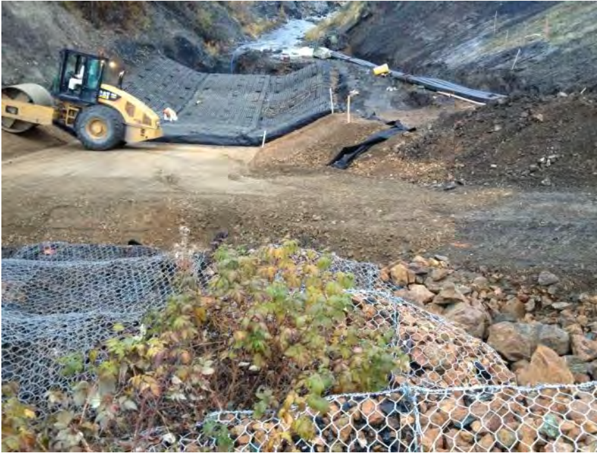
Looking east: Transition from gabions to Armorflex
