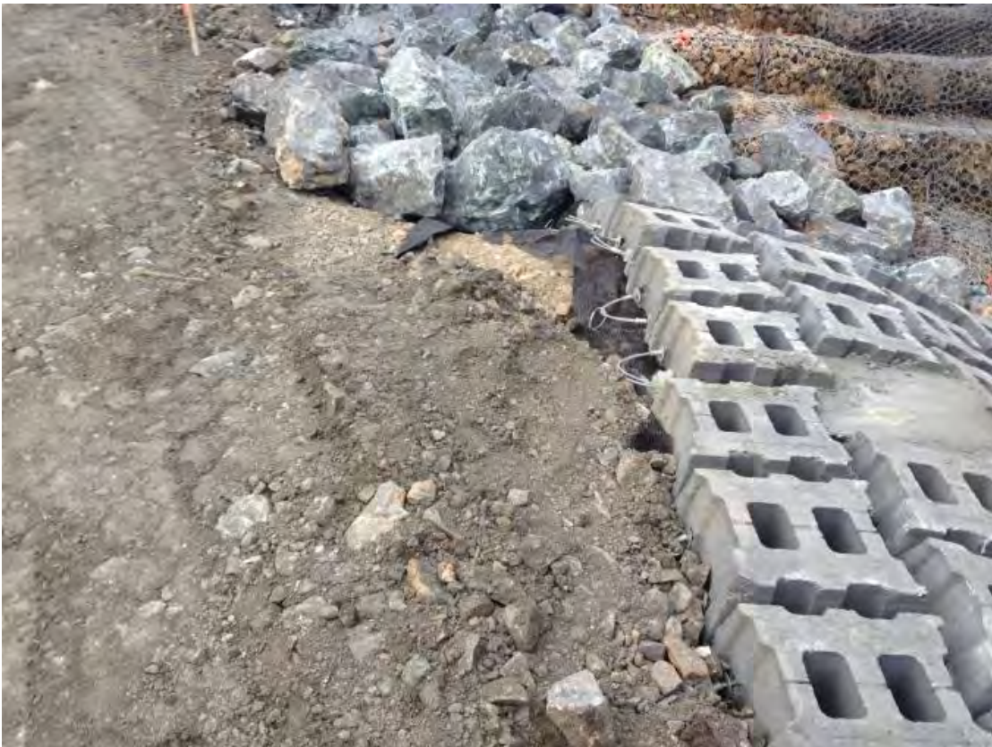
Looking west: Some of geogrid on south side not covered and compacted
