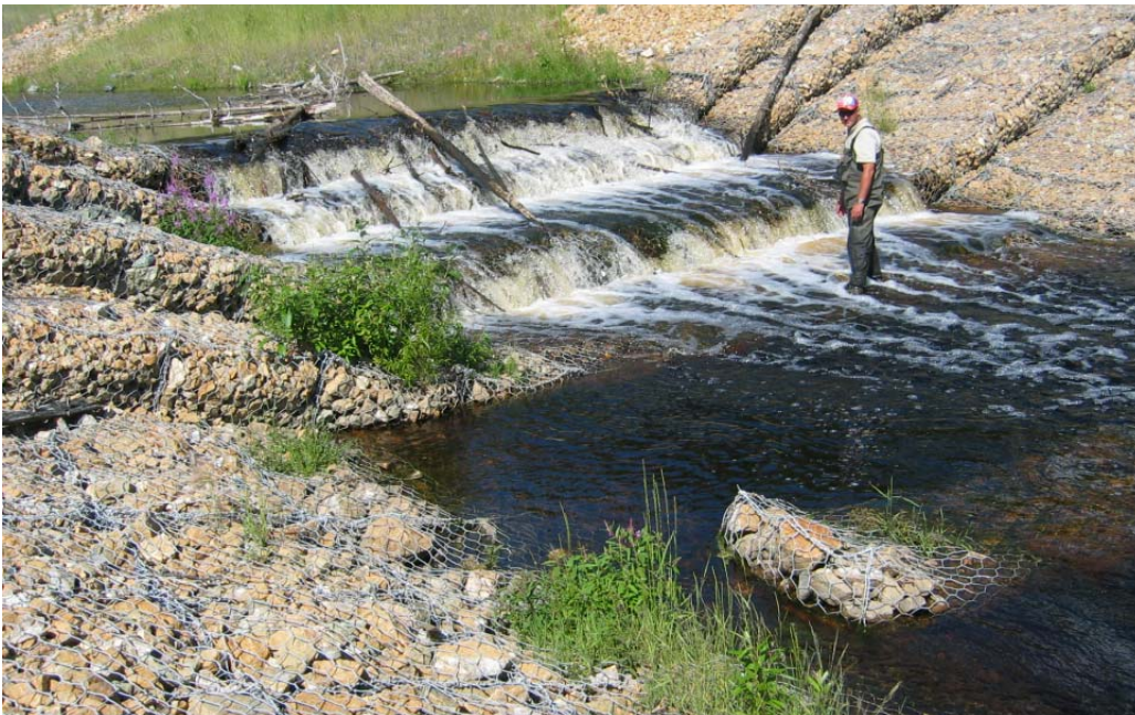
Photo : The upper most constructed rapid during July. The benthic baskets were placed immediately in front of the technician on the wide bench.
