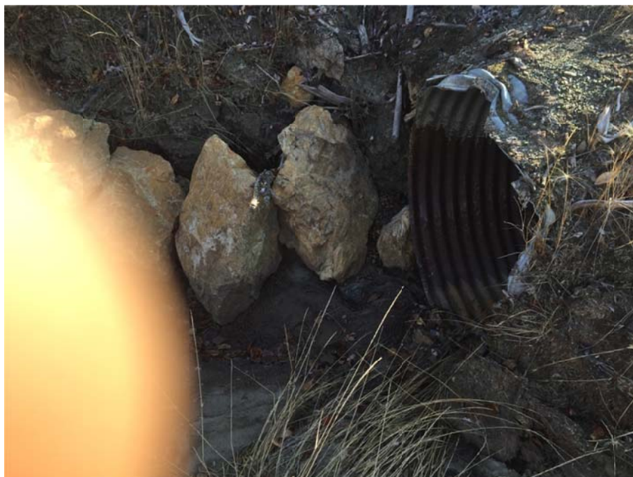
Photo 2 – Culvert near the gate following debris removal
