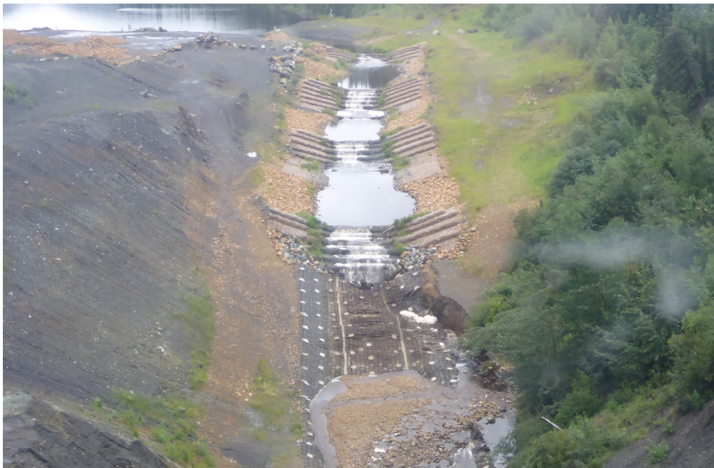
Photo 10: Aerial view of the gabion structures at Reach 10, with Hudgeon Lake in the background. Photo taken July 16, 2018.
