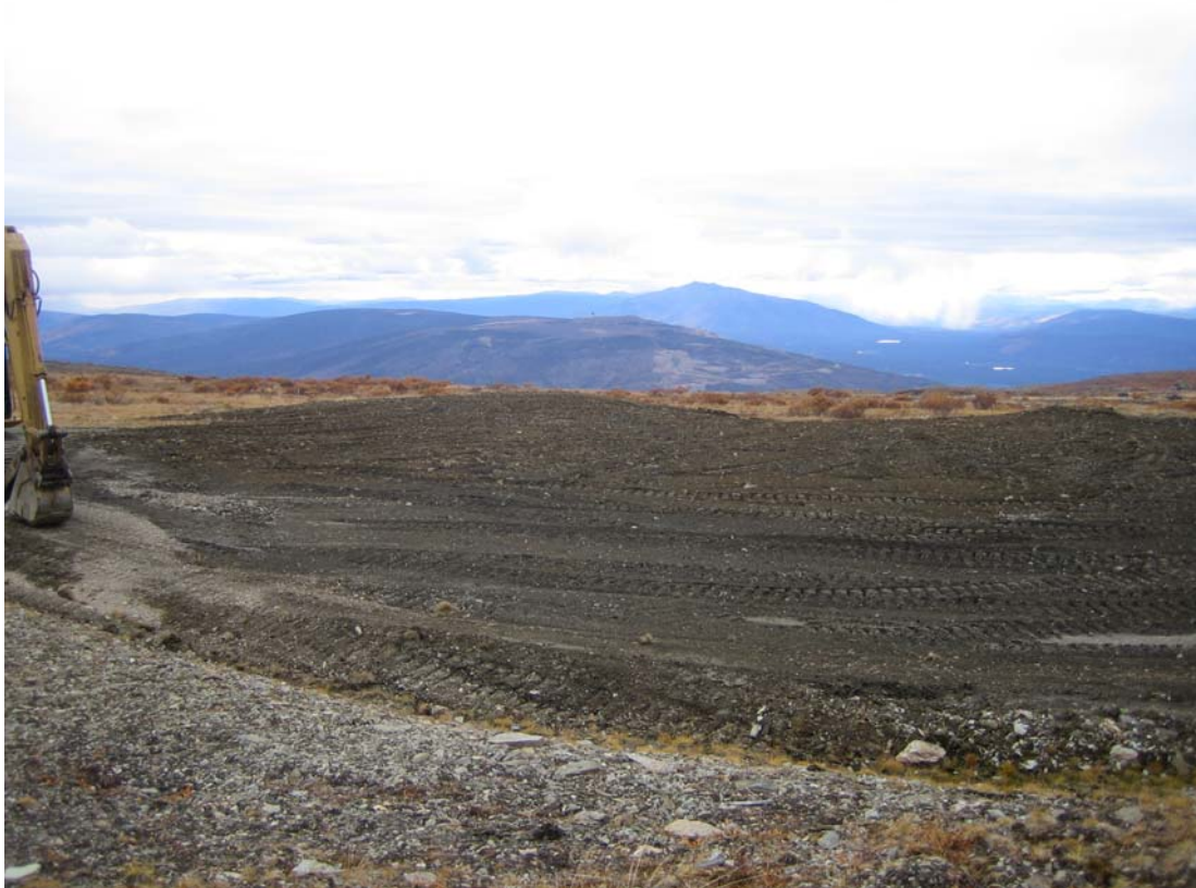
Photo 10: Photo 8: View of Shamrock J vent shaft filled and mounded with building removed.
