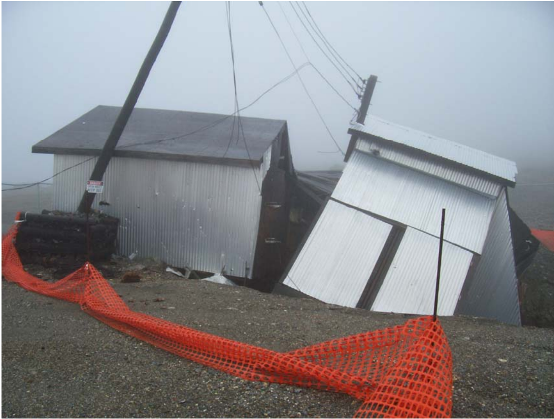
Photo 9: View of Shamrock J building partially collapsed over open vent raise.
