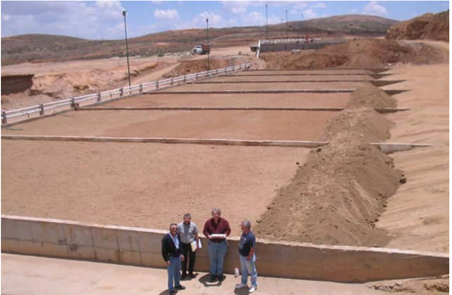
FIGURE 4. EXAMPLE OF TAILINGS VAT LEACH SYSTEM
