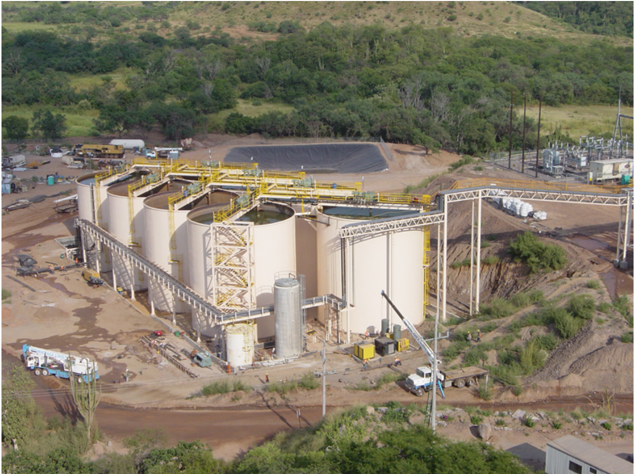
FIGURE 5. EXAMPLE OF CIP/CIL SILVER RECOVERY CIRCUIT
