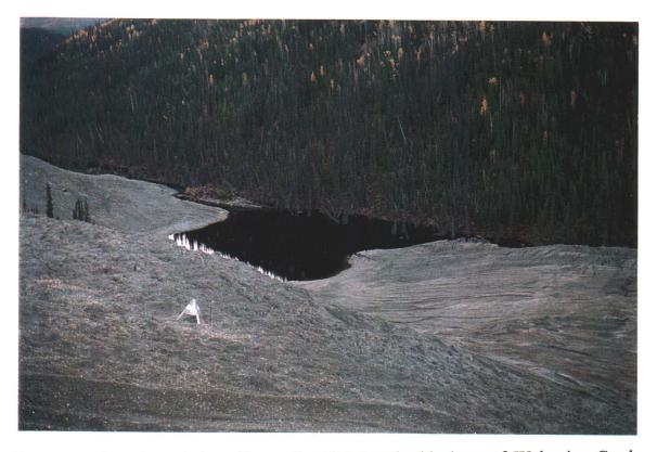
Photograph 2-8: Toe of the tailings piles showing the blockage of Wolverine Creek resulting in the formation of two ponds
