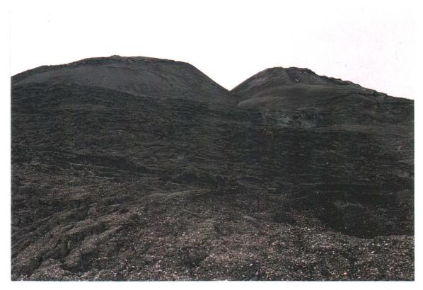
Photograph 4.7: Southeast slope of tailings pile from Wolverine Creek showing barren surfaces absent of any groundcover.
