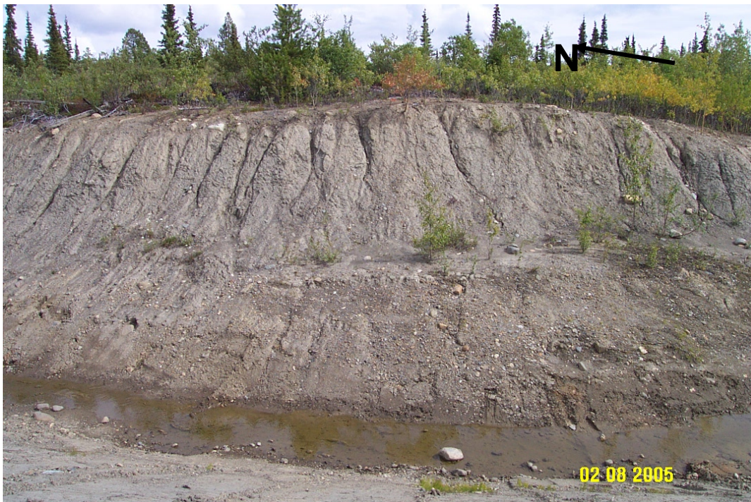
Photograph 2: Station JD7. Interception Ditch is approximately 3 m deep into till blanket overlying weathered phyllite.
