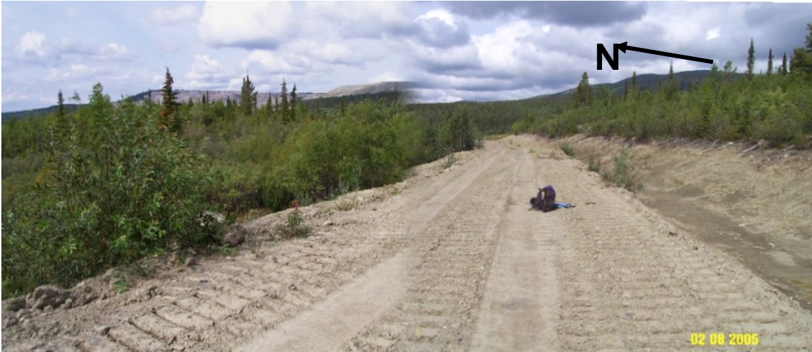
Photograph 3: Station JD4. Berm constructed on downslope side of shallow Interception Ditch is about 1 m deep into till blanket.
