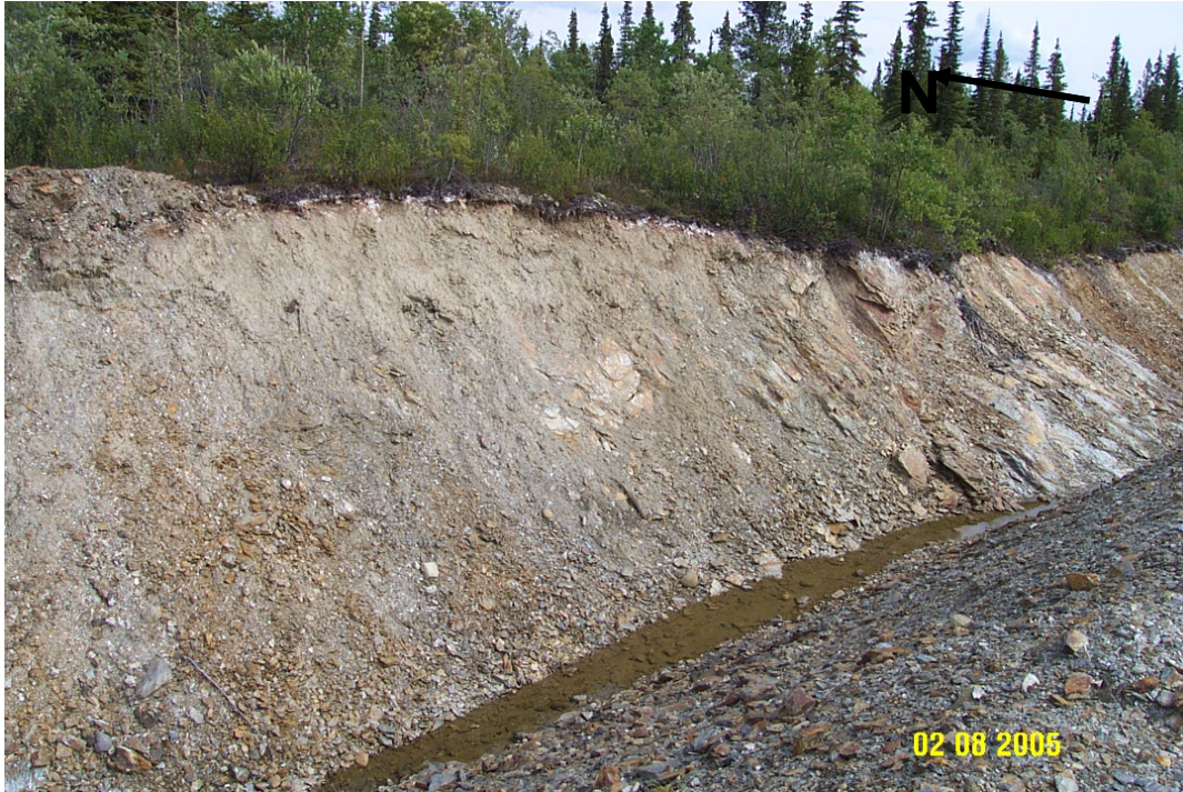
Photograph 1: Station JD1. Interception Ditch is approximately 4 m deep into rusty weathering, steeply dipping ( \sim 45^\circ SW) fissile phyllite.
