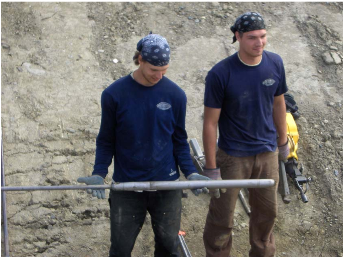
Photo 8: Drillers with split spoon sampler
