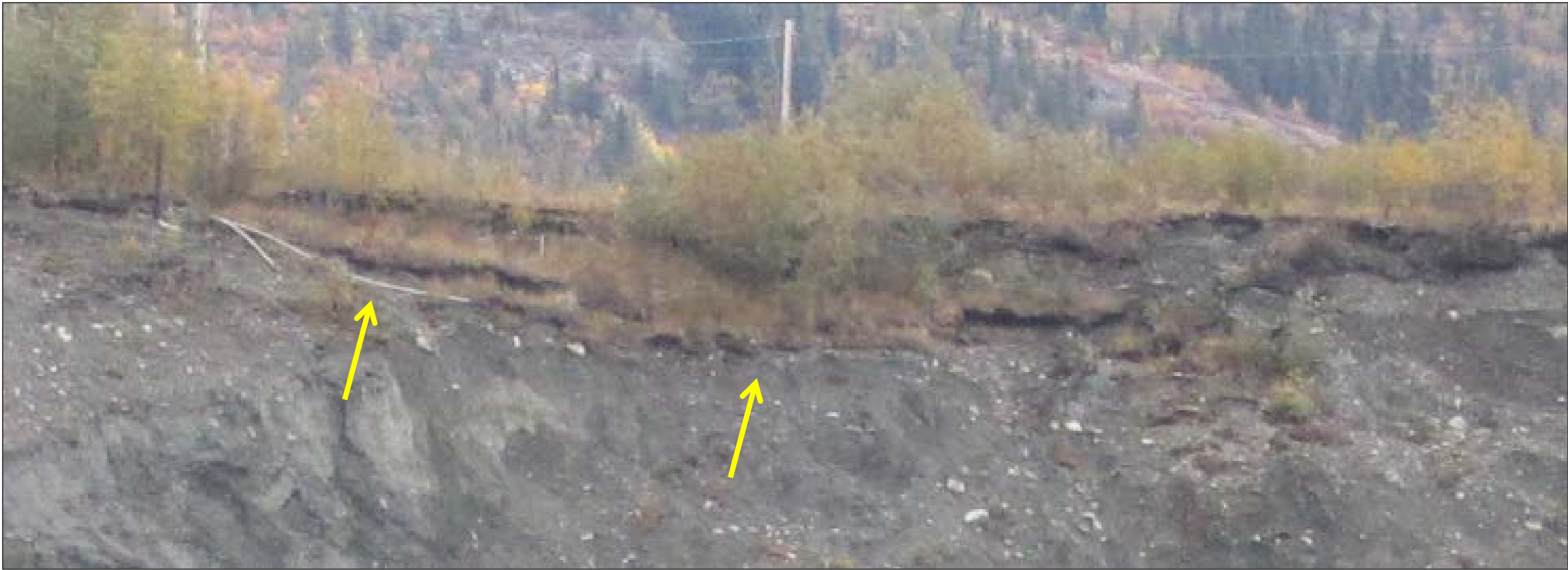
2015 PHOTOGRAPH OF CREST OF EAST WALL, BACKSCARP OF INSTABILITY ZONE, VIEW LOOKING EAST
