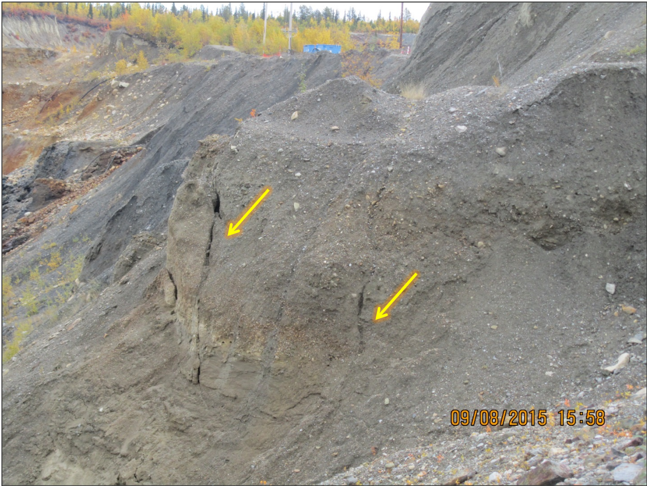
NORTH SIDE OF WEST WALL, VIEW LOOKING SOUTH FROM CREST ARROWS INDICATE CRACKS
