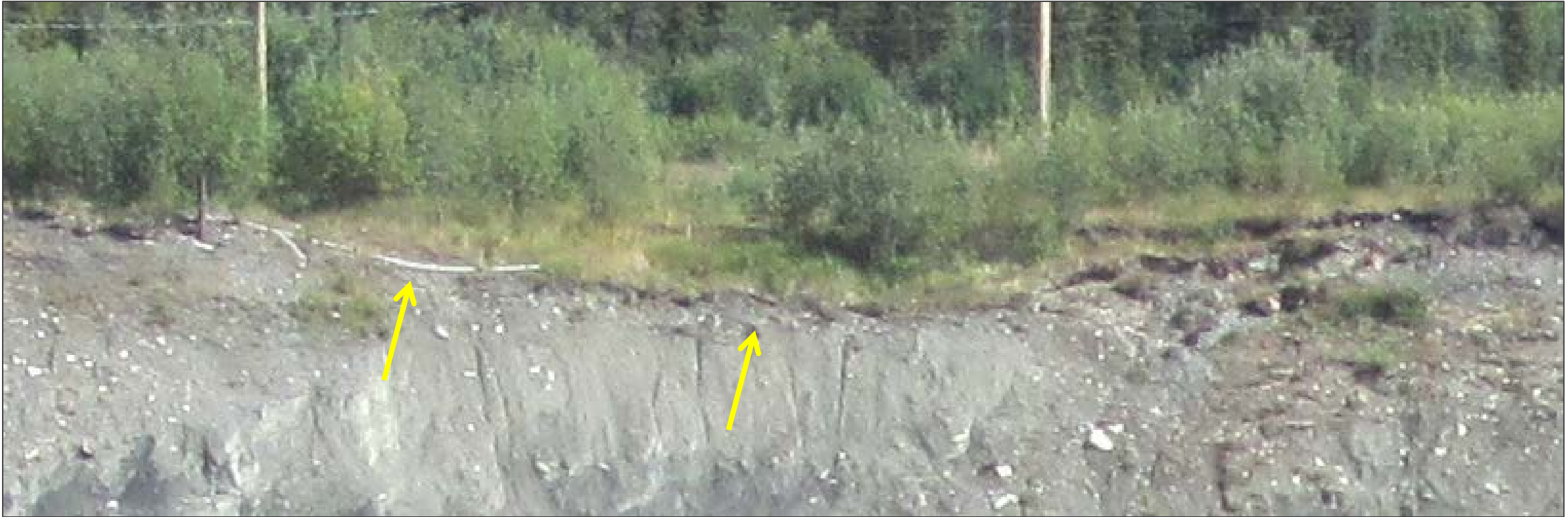
2014 PHOTOGRAPH OF CREST OF EAST WALL, BACKSCARP OF INSTABILITY ZONE, VIEW LOOKING EAST
