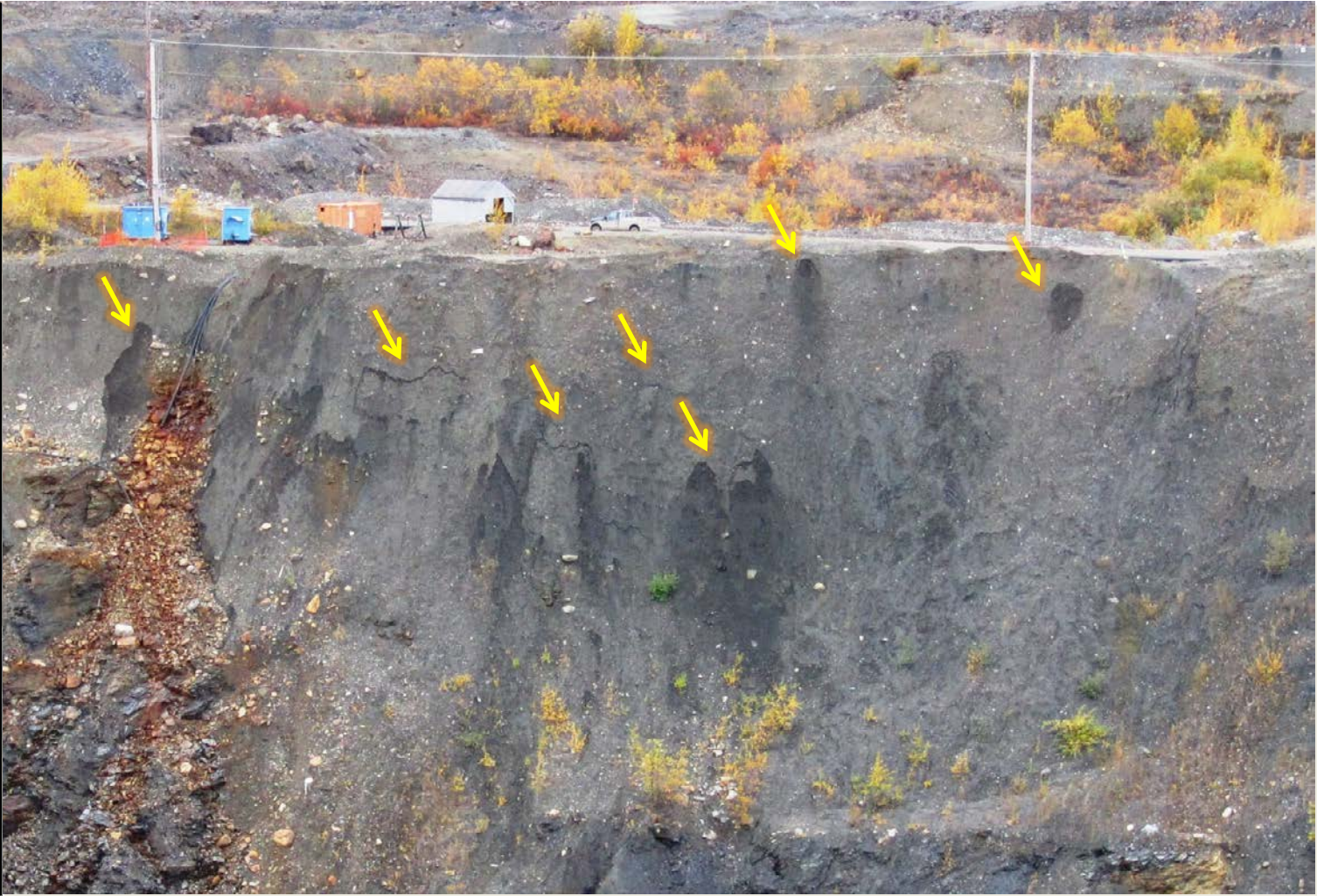
2015 - SOUTH SIDE OF UPPER WEST WALL, VIEW LOOKING WEST YELLOW ARROWS SLUMPED AREAS
