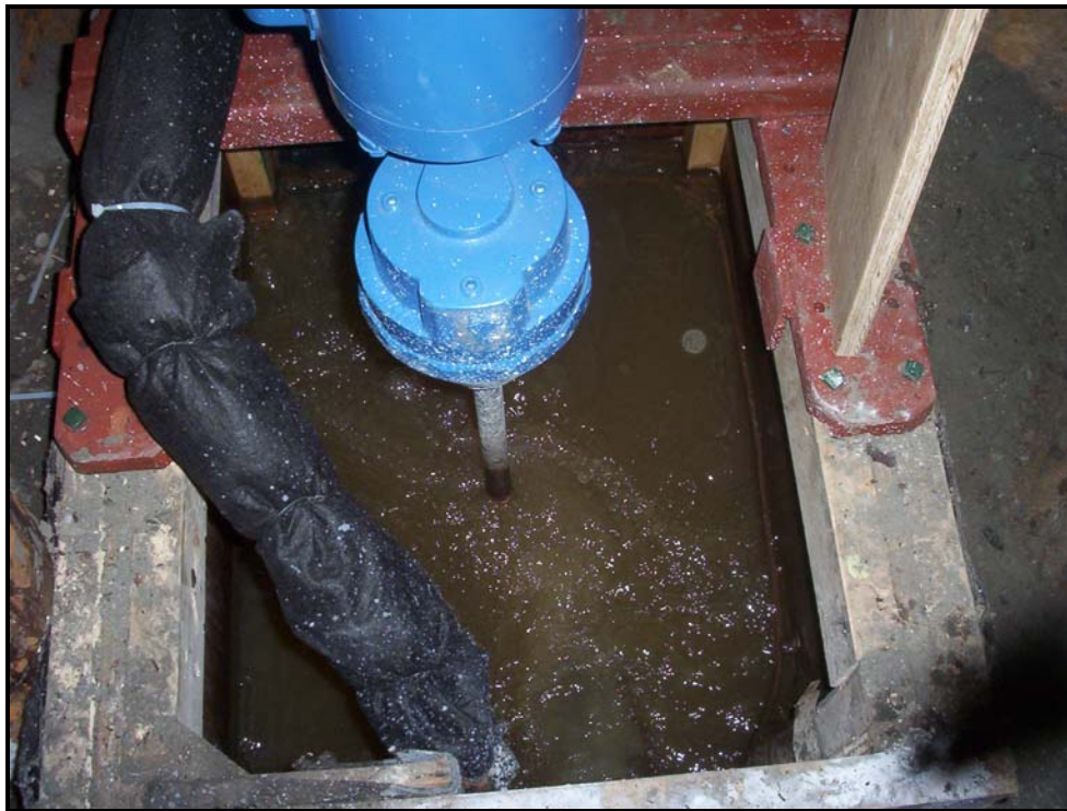
Plate 3 New mixing box for G300 adit flow (immediately below weir).
