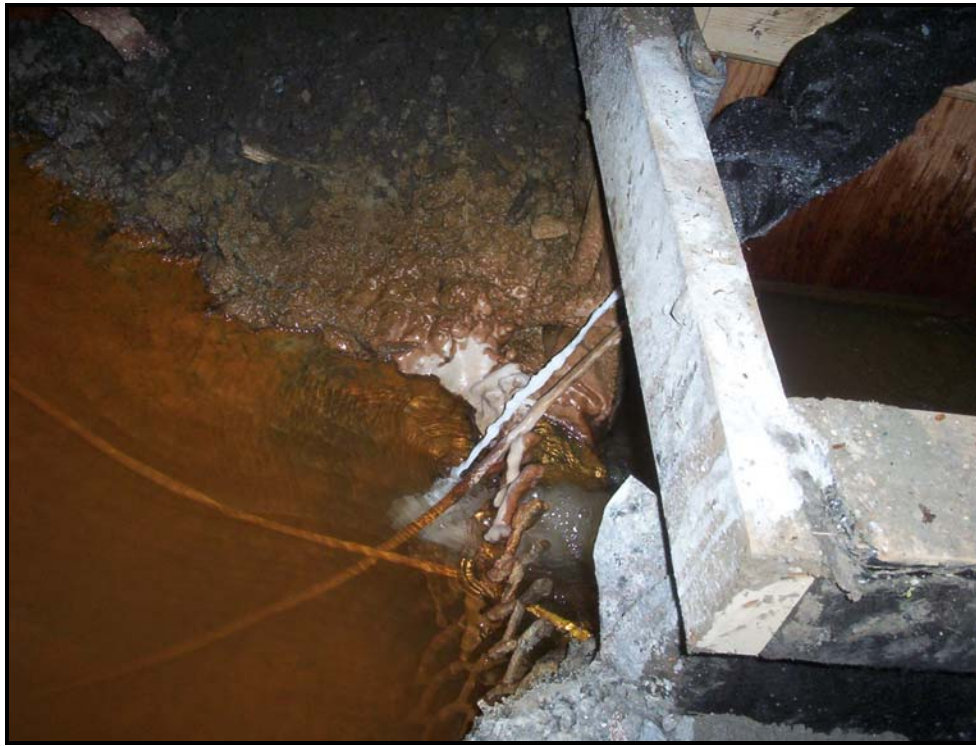
Plate 2 Lime slurry application point and mixing box in G300 adit.
