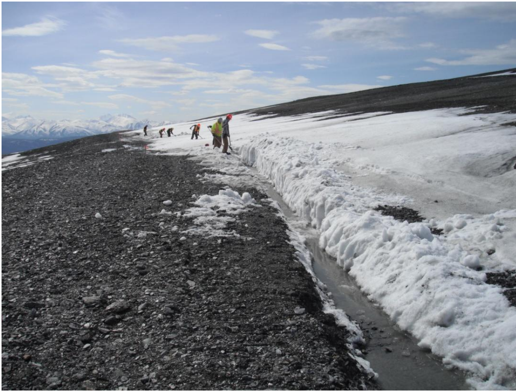
# 7 May 17, 2011 – Hand excavation of east side of Bench 4 ditch.
