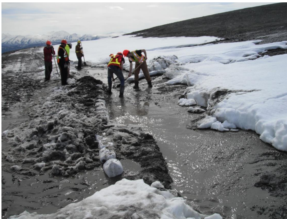
# 6 - May 16, 2011 – Bench 5 ~ Station 0 + 080 Sand-bagging to redirect overflow.
