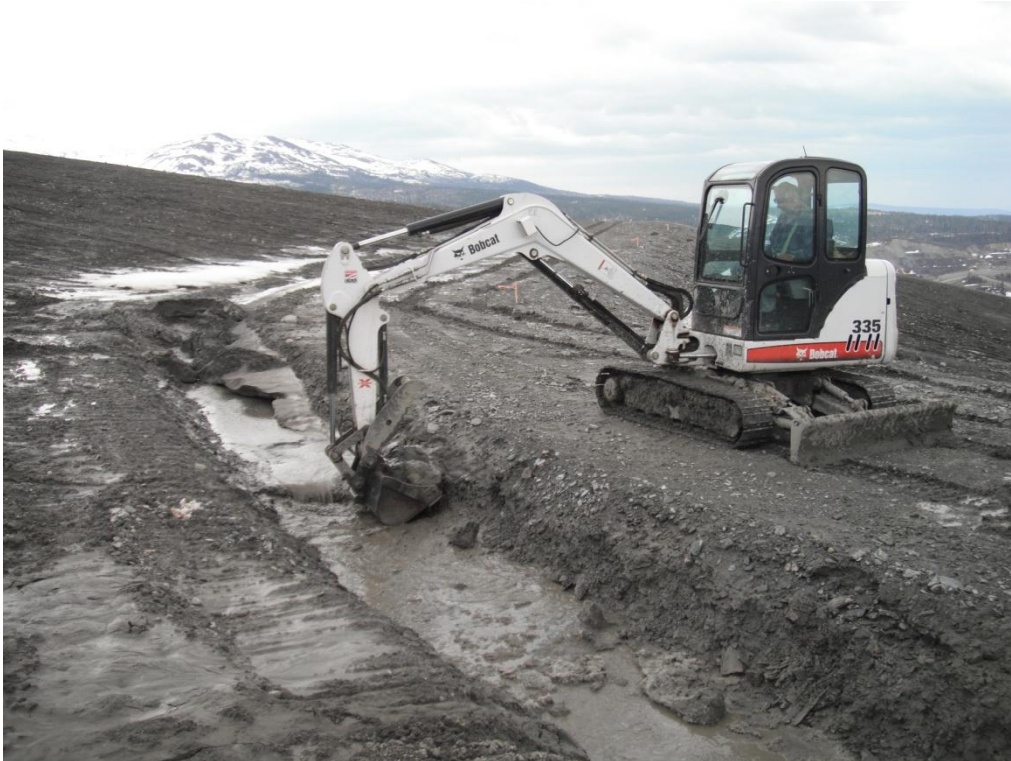
# 12 - May 19, 2011 – Excavating ditch sediment from Bench 4 ditch.
