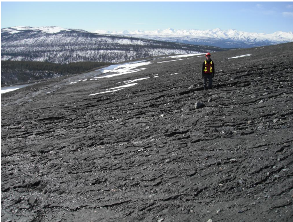
# 4 - May 16, 2011 – Erosion rills on cell cover below east side of bench 5.
