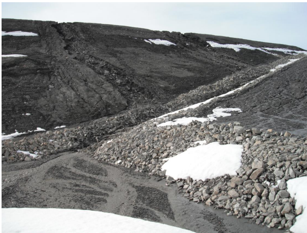
# 5 - May 16, 2011 – Toe Berm conditions. Note sediment and erosion gullies.
