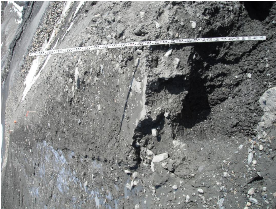
# 9 - May 17, 2011 – Erosion gully at Toe Berm Crest ~ Station 0 + 080.
