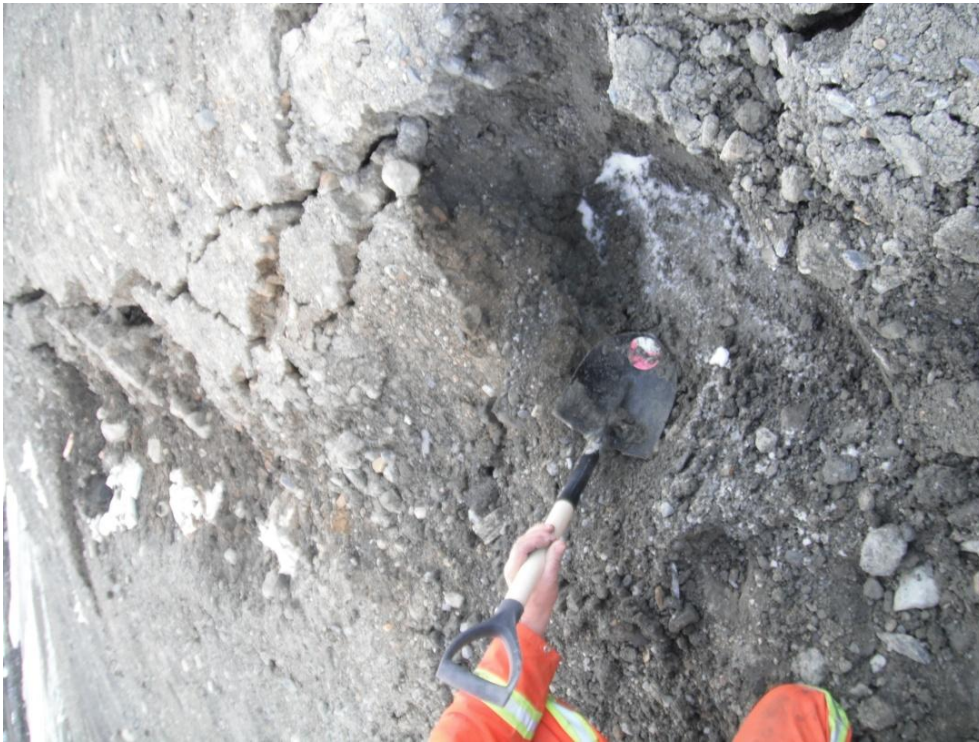
# 3 - May10, 2011 – Toe Berm conditions near liner elevation. Note buried snow.
