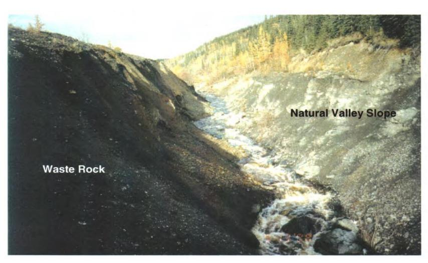
View of the Clinton Creek Waste Rock Dump circa 2000, up against the north slope of the Clinton Creek valley. Note there has been downcutting through the waste rock and into the north valley slope.
