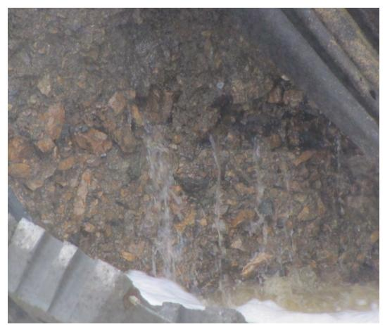
Figure 8: Observed localized flow and probably internal erosion during the Fall 2019 field program.
