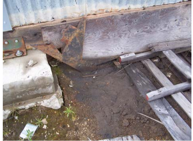
Photo 50: Example of soil staining
