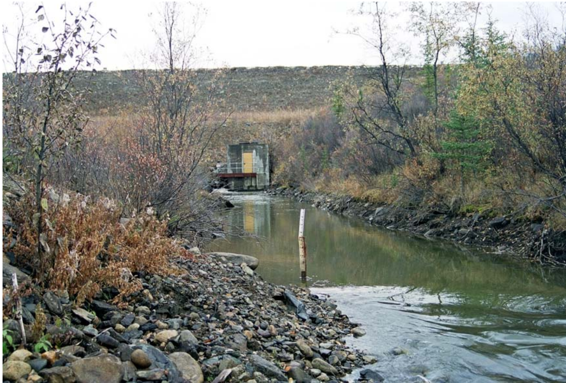
Photo 11. Riparian outflow channel from the Fresh Water Supply Dam (FWSD) to South Fork Rose Creek, with the valve house in the centre of the photo. A notch will be cut through the embankment to the left of the photo to permanently lower reservoir water levels.
