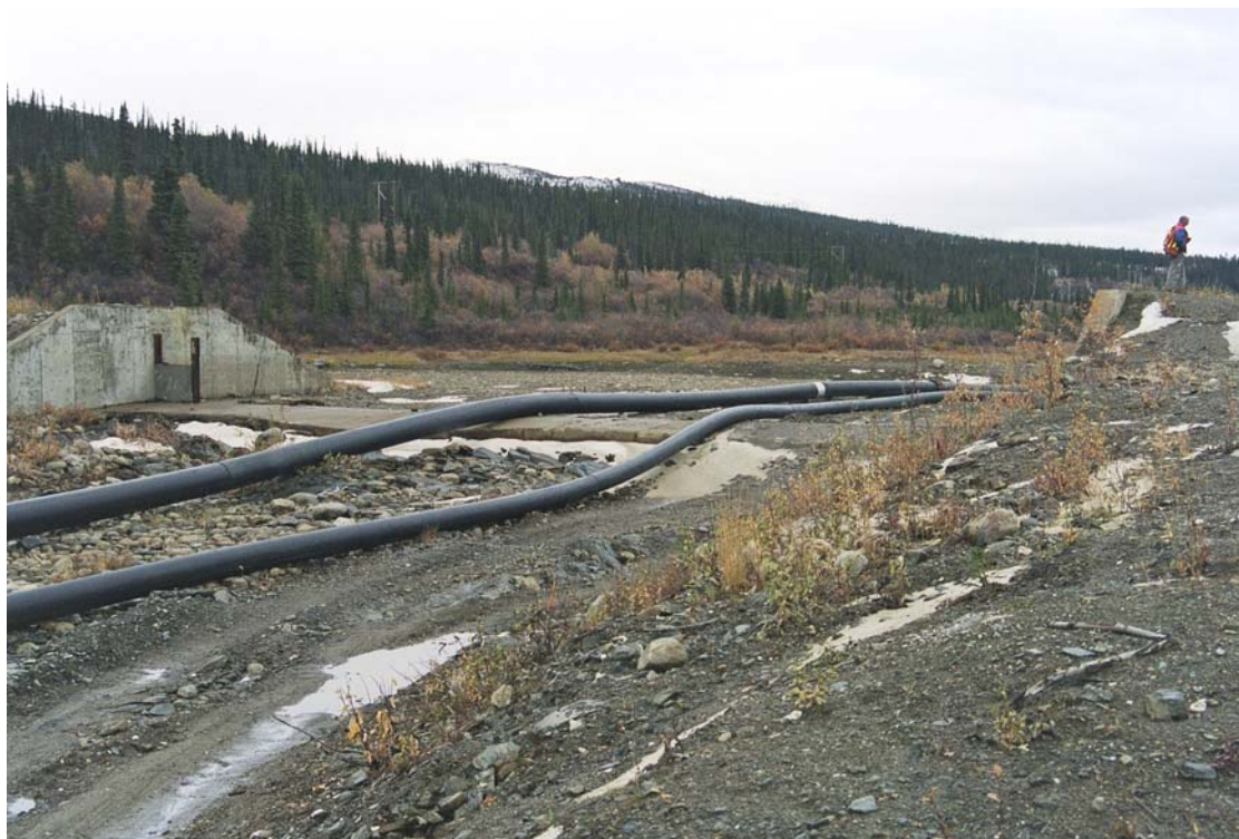
Photo 10. The Fresh Water Supply Dam (FWSD) spillway showing the syphon pipes used to lower the reservoir water level.
