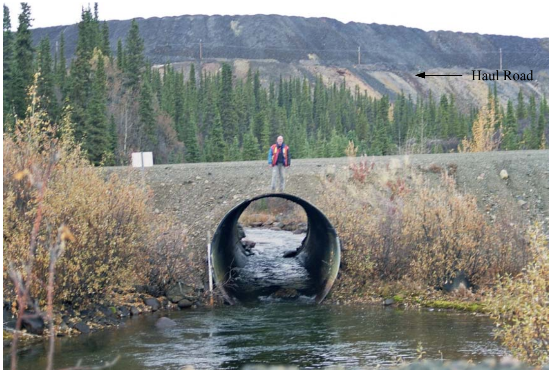
Photo 13. North Fork Rose Creek flowing through the 14 ft (4.3 m) culvert through the main access road to the Mine Site. The Mine Haul Road is in the background.
