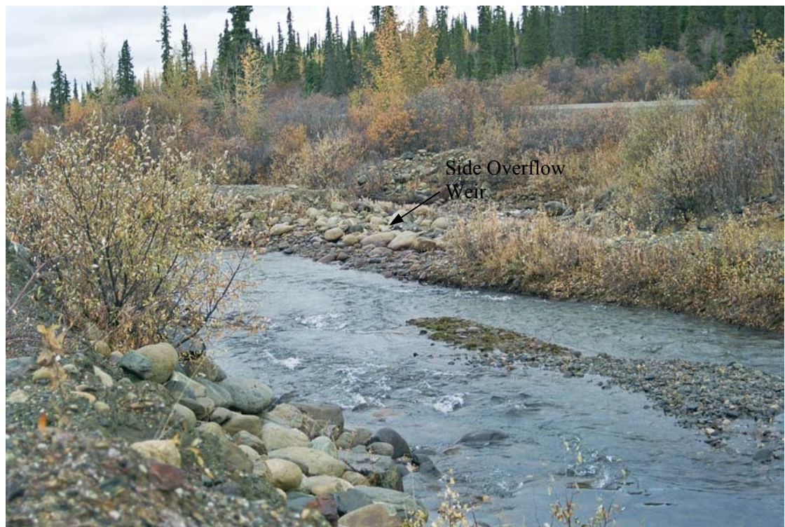
Photo 14. View across North Fork Rose Creek to the side overflow weir in the centre of the photo, that allows excess flow to enter the North Fork Diversion. Creek flow passes into the downstream series of four Recharge Ponds and finally the Pumphouse Pond.
