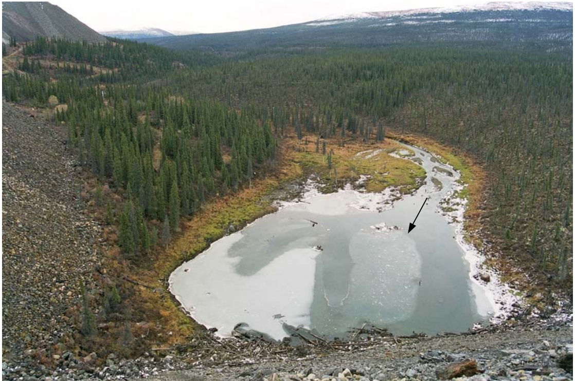
Photo 7. Upstream view of North Fork Rose Creek from the Haul Road with water ponded at entrance to flow-through rock drain. Mine rock dumps are visible along the left side of the photo.
