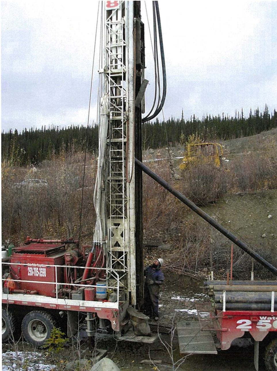
Photo I-1 Truck mounted drill rig at DHKC07-1. A 6" casing is being hoisted into position. Note the outcrop of silty gravel on the right.
