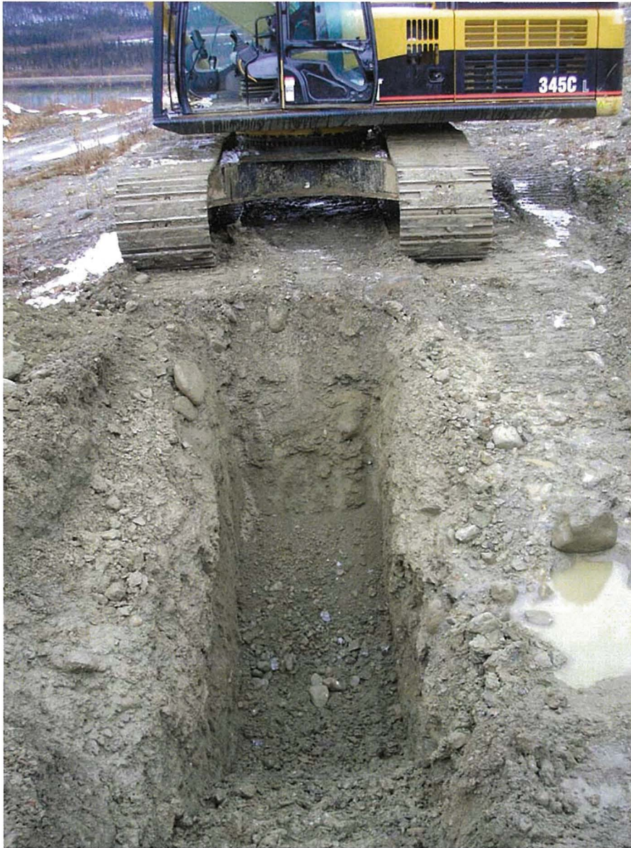
Photo I-9 TPKC07-1 exposed schist bedrock at 3.2 m below surface.
