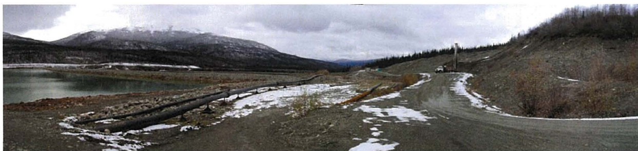
Photo I-6 DHKC07-3 and the intermediate dam. Bedrock is at 5.1 m depth in DHKC07-3. Note the 4 m high roadcut of sand and gravel on the right.
