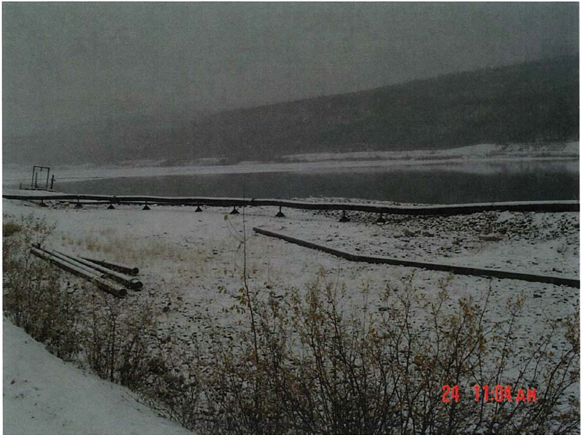
Photo II-5 Inlet of Existing Intermediate Dam spillway channel, looking upstream into impoundment. Note treated water effluent line across spillway channel.
