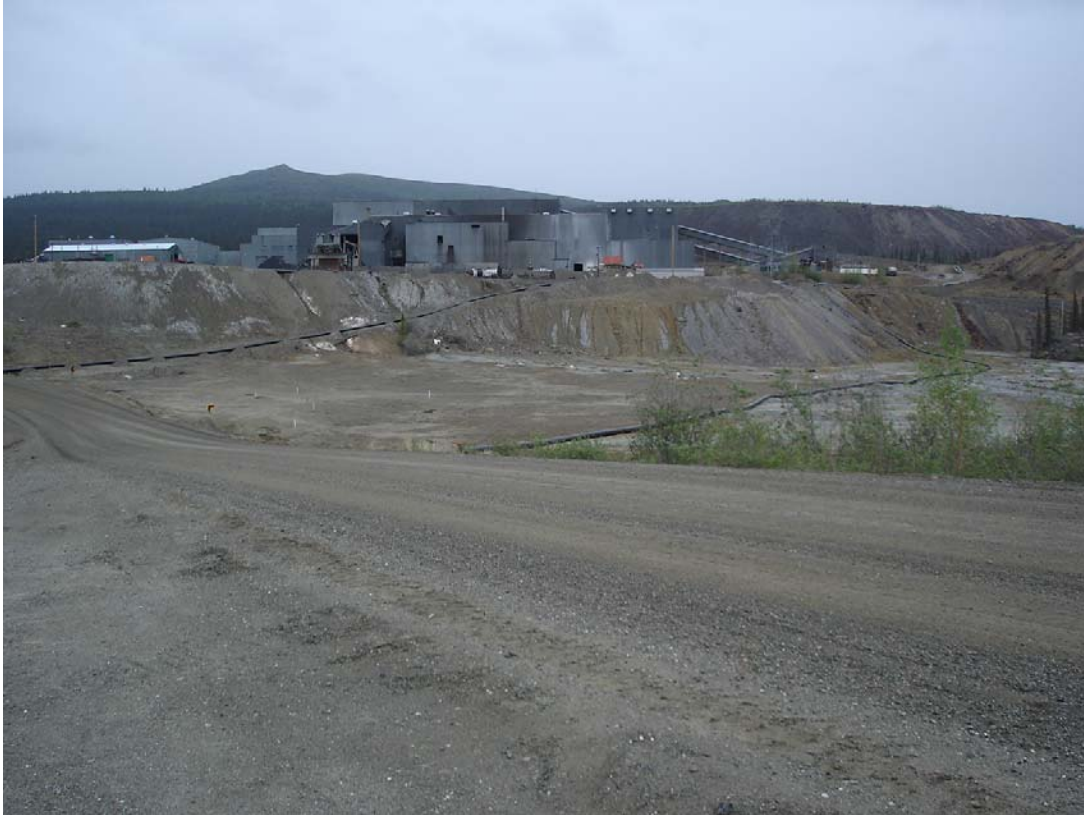
Photo 7: Northwestward view from the access road. The pipes on the surface of the ETA are piezometers installed during the drilling campaigns. June 2006.
