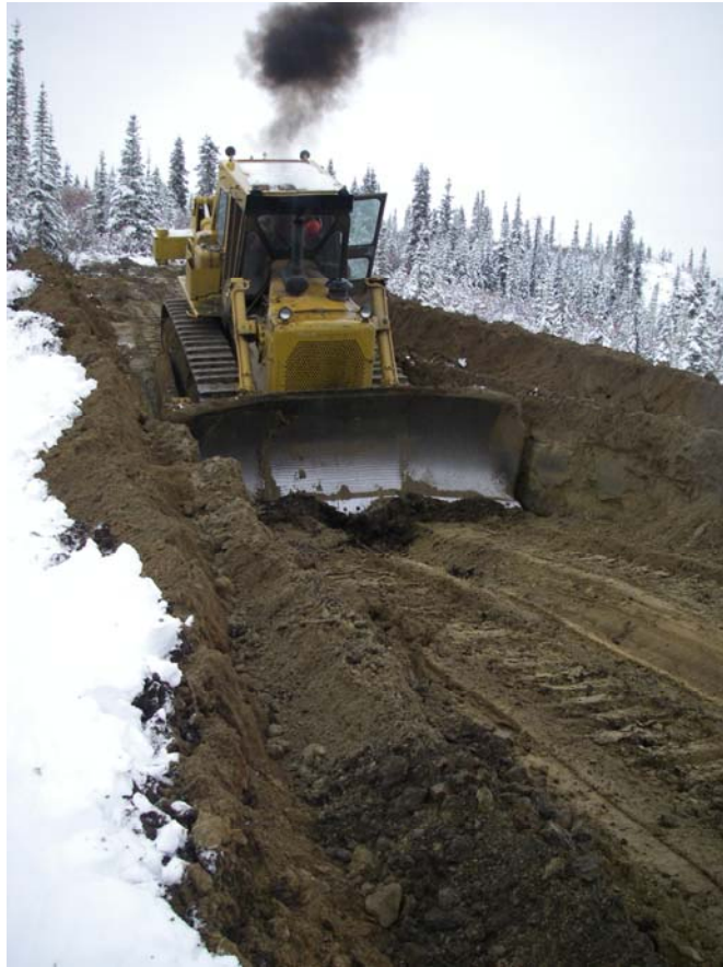
Photo #1: Excavating test pits at Wernecke tailings
