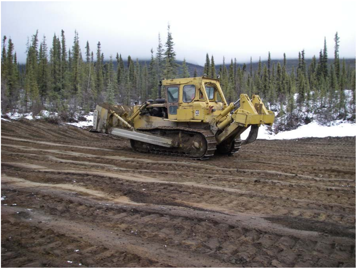
Photo #11: Compacting tailings after test pit excavations
