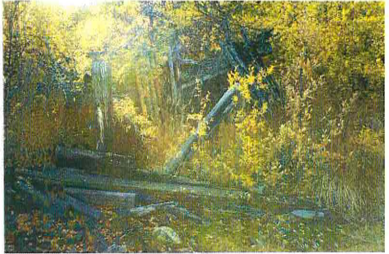
Photo 11-5. Galkeno 200 level adit. Portal is open but is unsafe. The timbers of the portal are collapsing.
