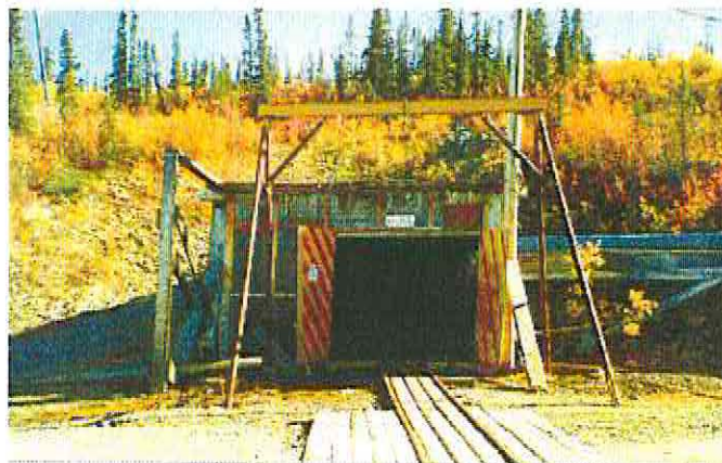
Photo 6-15 : Ruby 400. Adit structure with rail tracks extending from the structure and utilidor on right..
