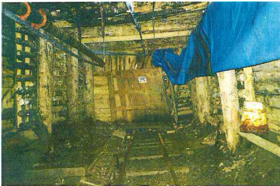
Photo 25-8: Interior of portal. Note drainage ditch to bottom left and partially collapsed door. Azimuth 060°)
