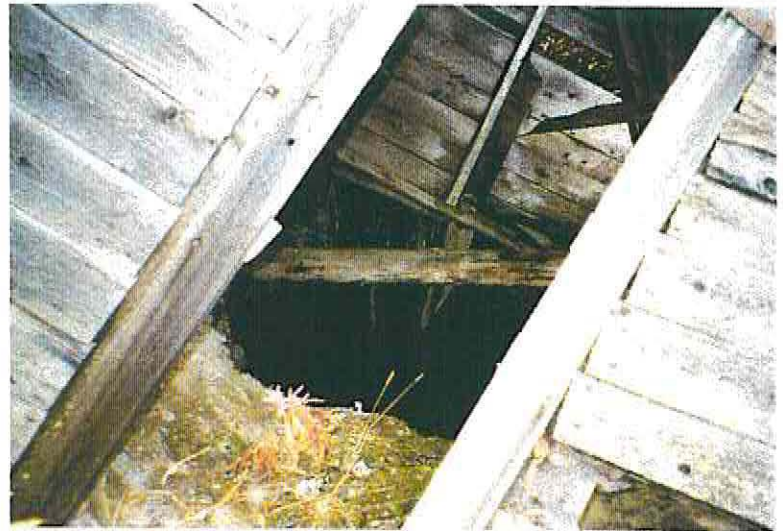
Photo 22-11: Collapsed structure enclosing shaft across Sourdough Hill Road from Bellekeno 100 level adit
