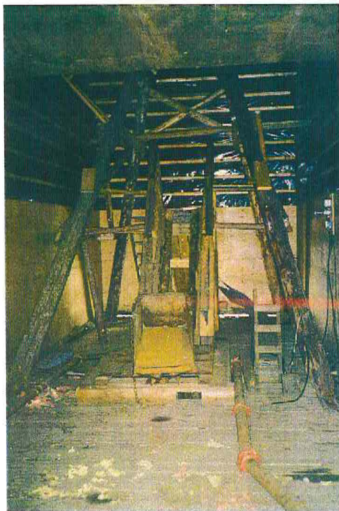
Photo 26-7: Interior of Lucky Queen headframe building (Bldg. 26-A) showing open manway and boarded shaft opening.
