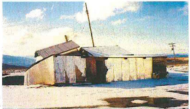
Photo 36-2 : Keno No.9 Shamrock J18 Vein Raise Building (36-A). Note collapse of building into falling underground workings and fencing around opening. Also, transformer on power pole in background. (Azimuth 290o).
