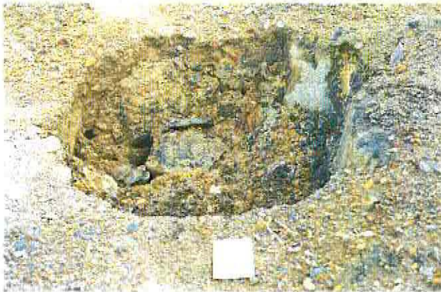
Photo 11-2. Subsidence over adit workings, near the McLeod Shaft. The collapsed area measures approximately one meter across.
