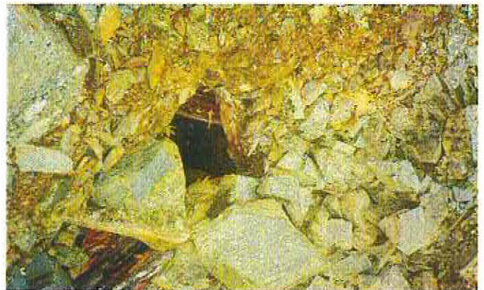
Photo 29-2: Northern partly collapsed adit, upper workings.
