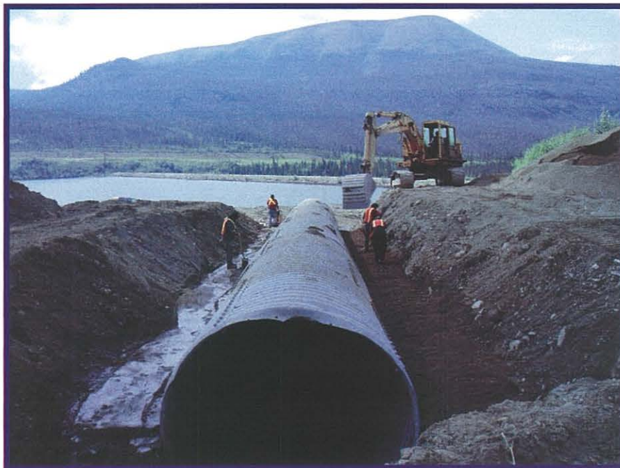
Photo 6: Placing and compacting sand and gravel along the sides of the culvert.
