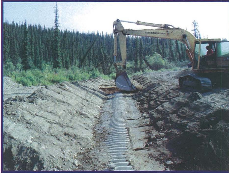
Photo 9: Placing sand and gravel over top of culvert.
