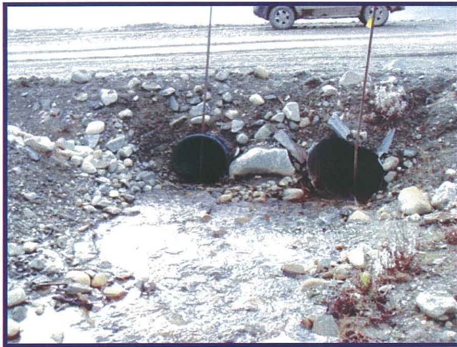
Photo 1: View of inlet of old culverts prior to construction activities. (Photo taken September 29, 2002)
