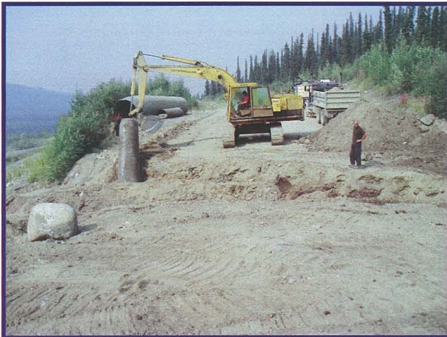
Photo 10: Removing the two old culverts.
