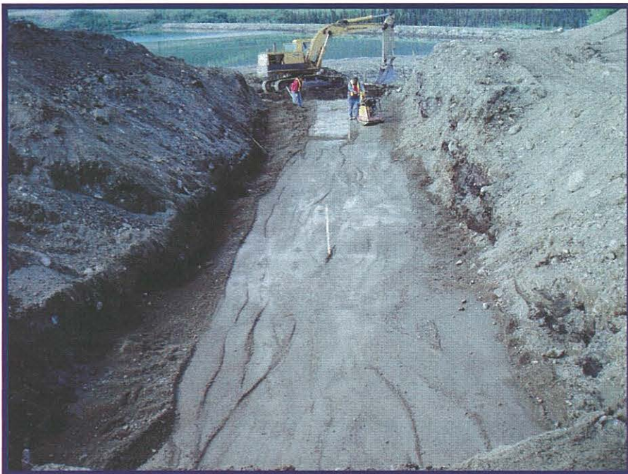
Photo 4: Compacting the sand and gravel base prior to culvert placement.
