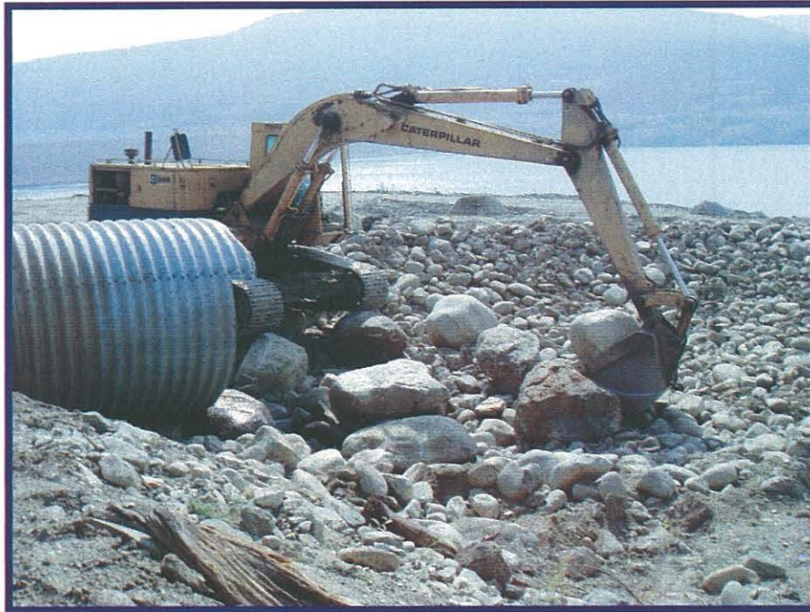
Photo 11: Placing large boulders in the plunge pool.
