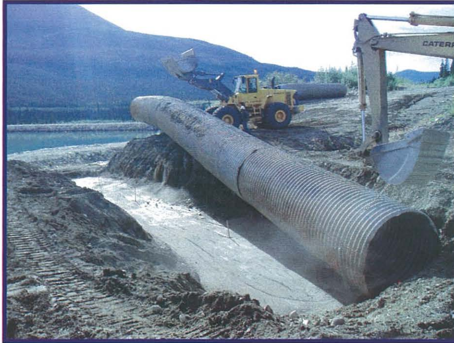
Photo 5: Placing the culvert in the trench.
