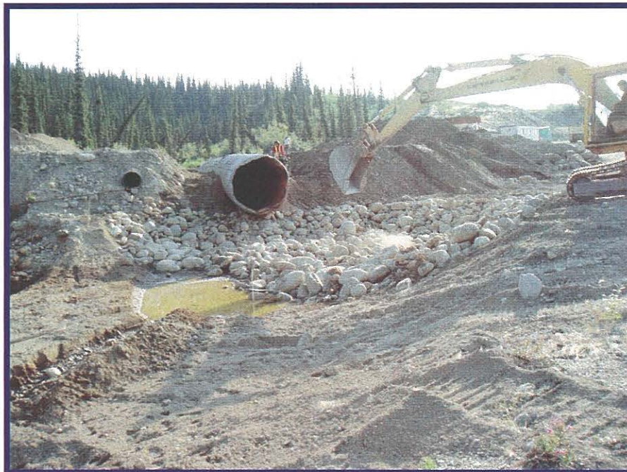
Photo 8: Placing rip-rap over sand and gravel base in plunge pool.
