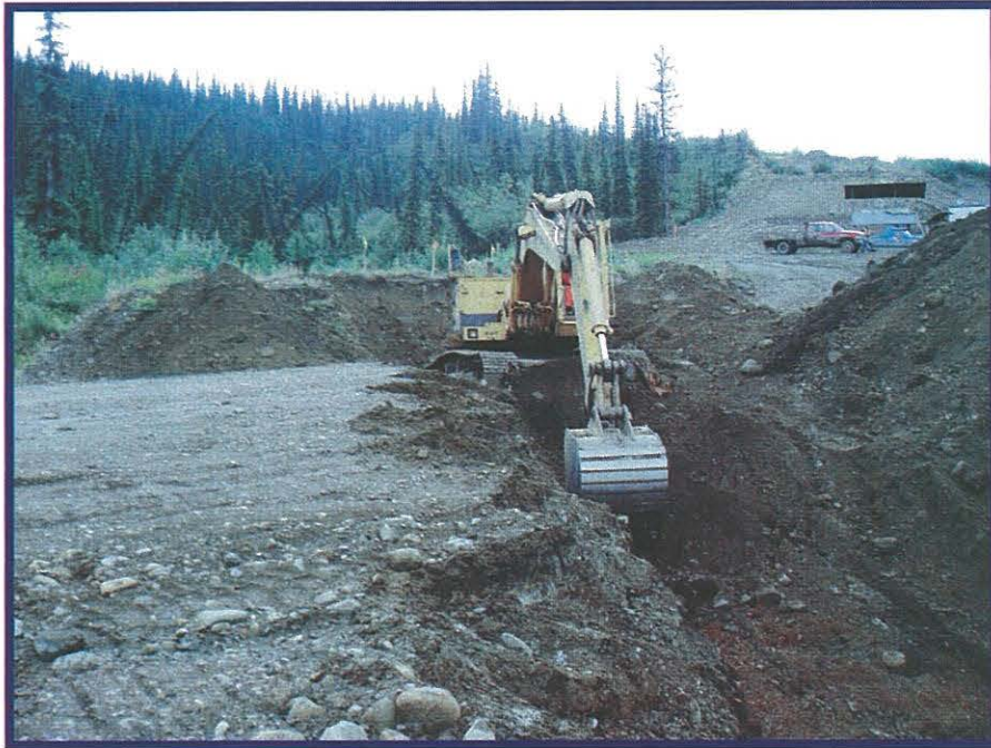
Photo 3: Starting the excavation for the culvert installation.
