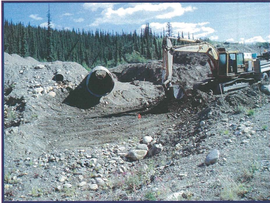
Photo 7: Excavating the plunge pool.
