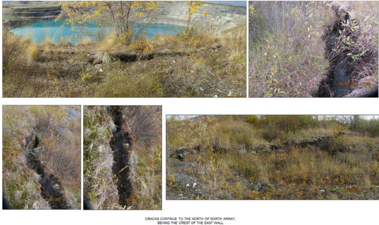
Figure 15: Cracks behind Crest of East Wall – Grum Pit
