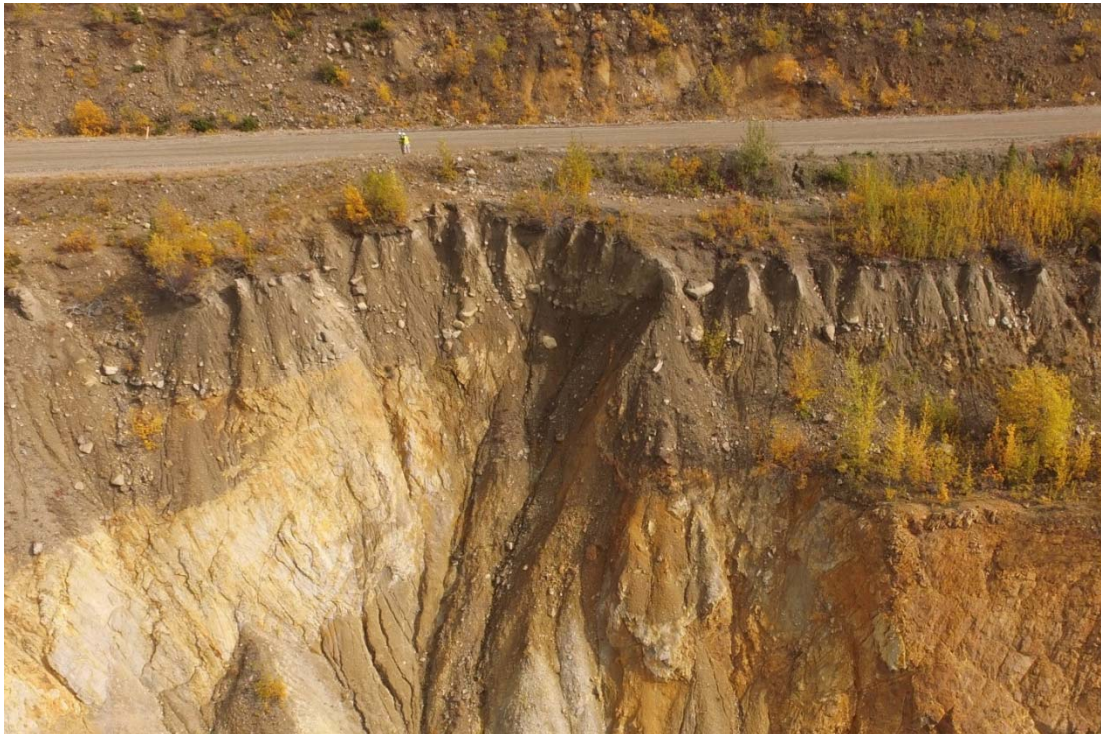
Figure 9: Critical Crest Regression Area in Faro Pit
