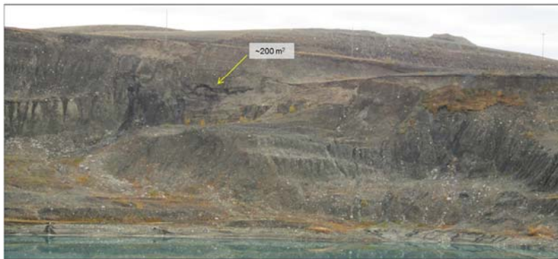
Figure 10: Example of Sloughing – Grum Pit
