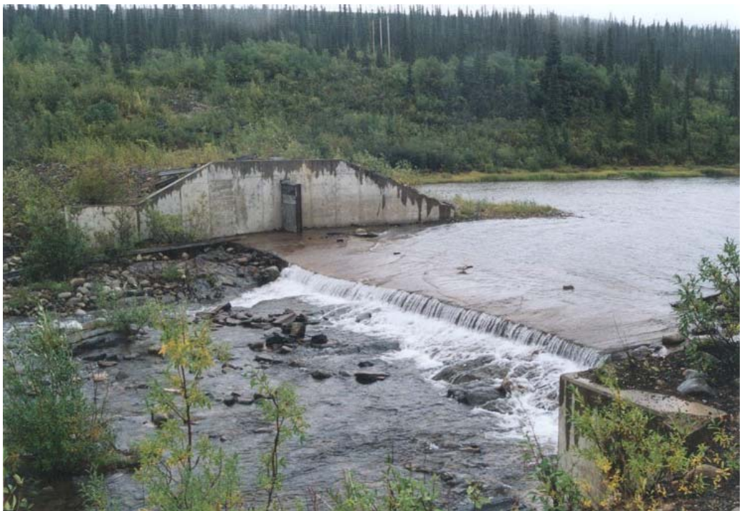
Photo 2: Spillway near North Abutment of FWSD
