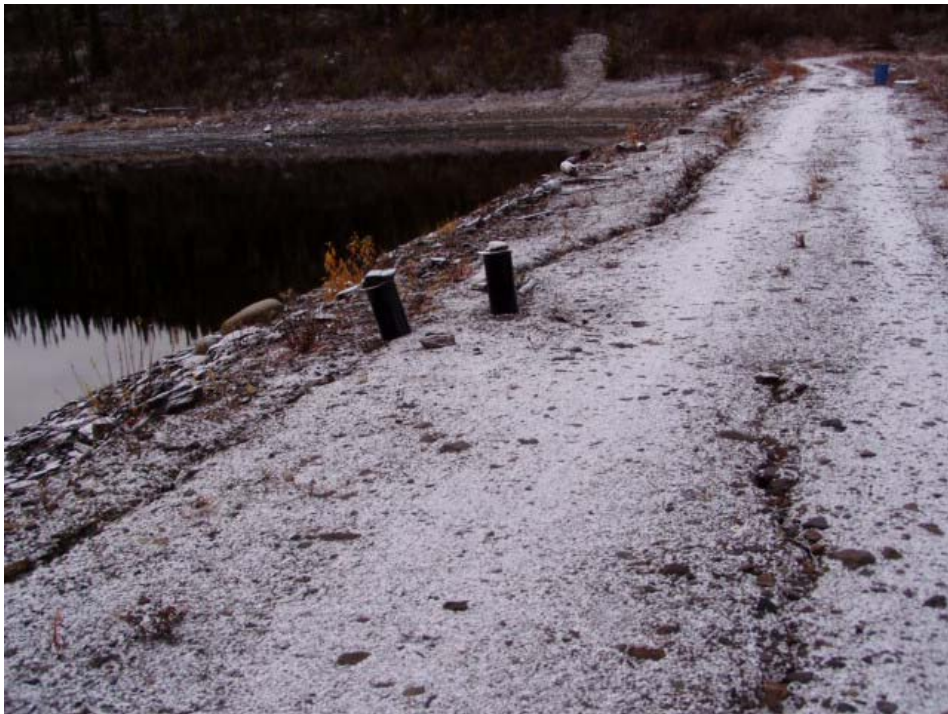
Photo 6: Cracking on the crest of the FWSD
