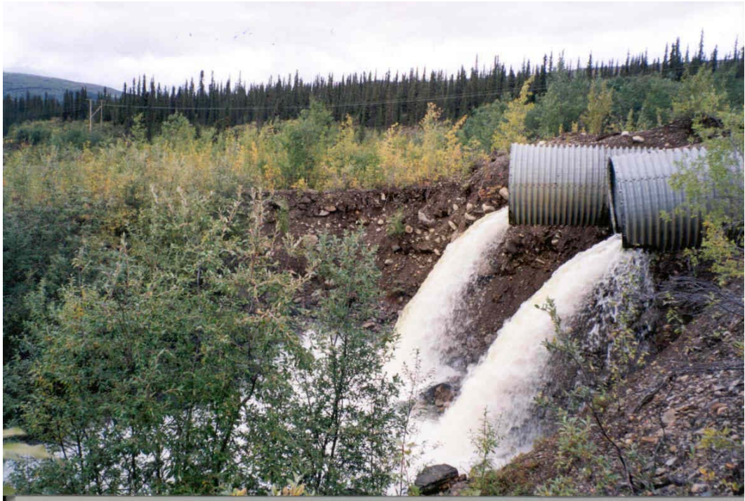
Photo 5: Culvert Discharge at downstream end of spillway
