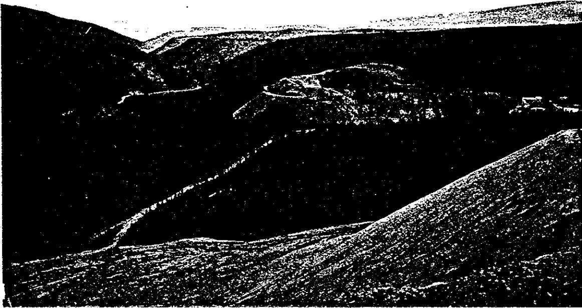
FIGURE 13 CLINTON CREEK TAILINGS IN FOREGROUND AND WASTE ROCK PILE IN MIDGROUND. BOTH EMBANKMENTS ARE UNSTABLE. NOTE CRACKING IN LOWER LEFT HAND CORNER.
