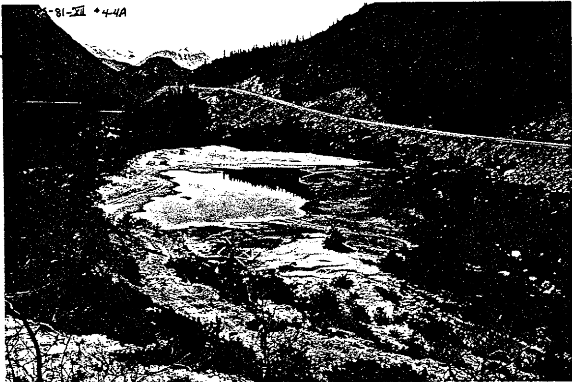
FIGURE 25 TAILINGS POND OF VENUS PROPERTY. WHILE IT HAS DRIED UP CONSIDERABLY SINCE TIME OF ABANDONMENT, HIGH WATER LEVELS IN THE POND (DURING SPRING MELT) MAY FLOW OVER THE BREACHED BERM (IN UPPER LEFT-HAND CORNER OF POND).
