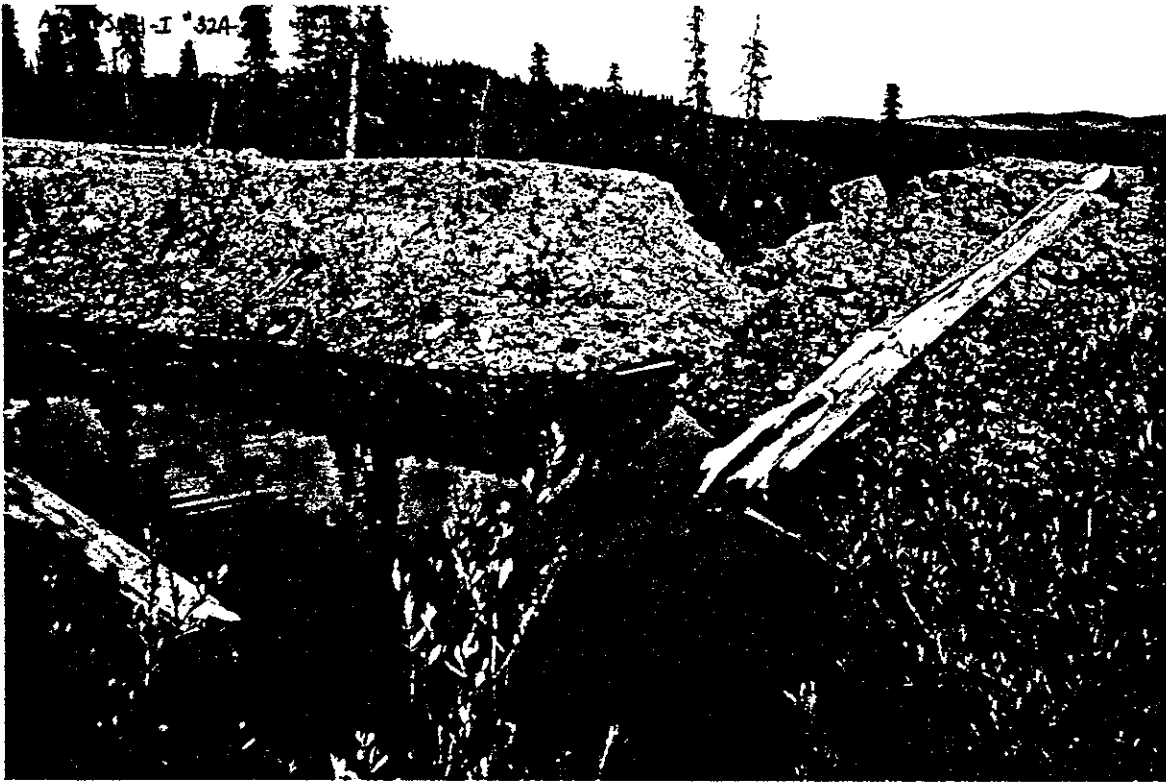
FIGURE 26 SECOND TAILINGS POND AT MOUNT NANSEN SHOWS A BREACHED EMBANKMENT.
