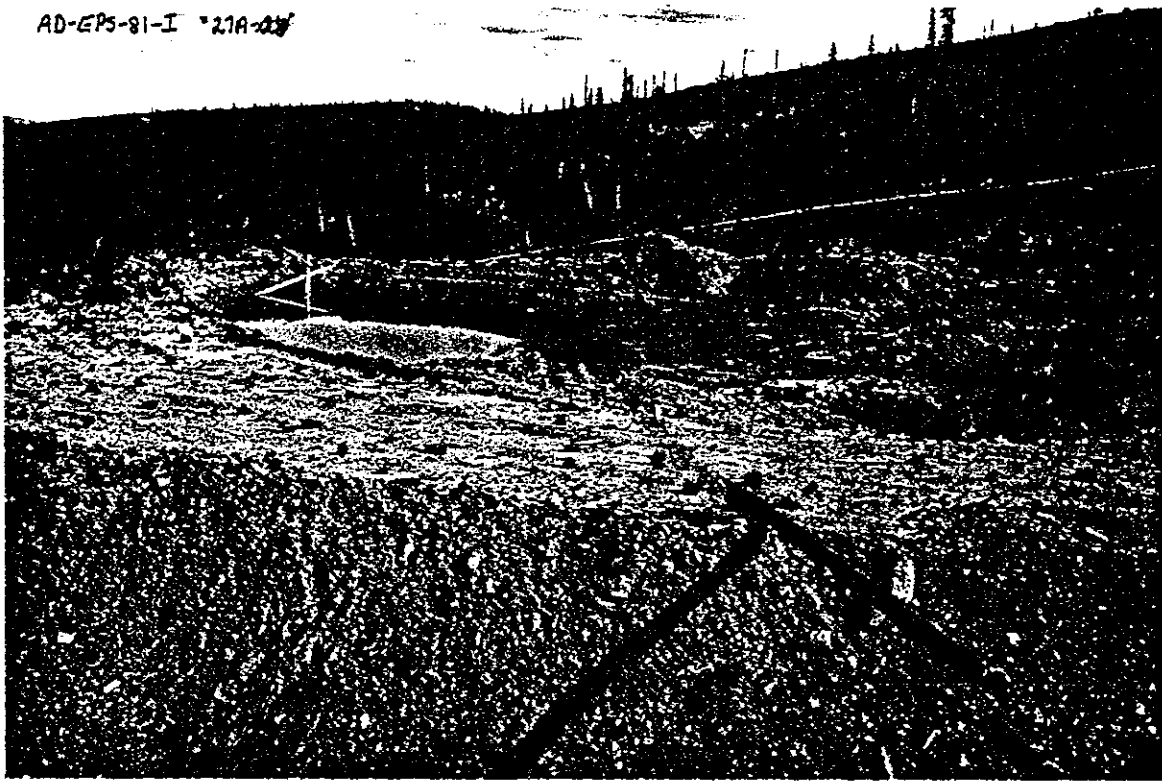
FIGURE 27 A SEVERED PIPE CONNECTING TAILINGS PONDS 2 AND 3 AT THE MOUNT NANSEN PROPERTY IS EVIDENT. (LOWER RIGHT HAND CORNER).
