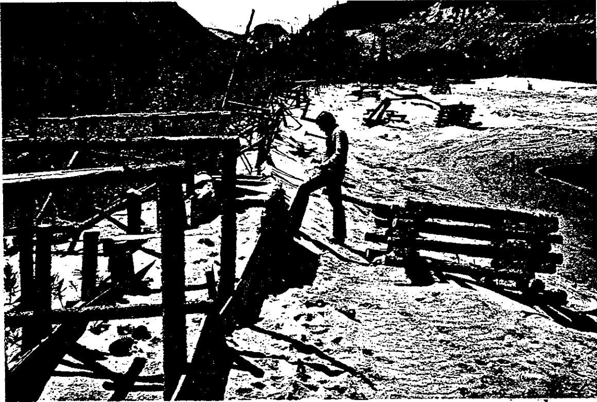
FIGURE 24 BERM OF THE TAILINGS POND AT VENUS MINE HAS COLLAPSED.
