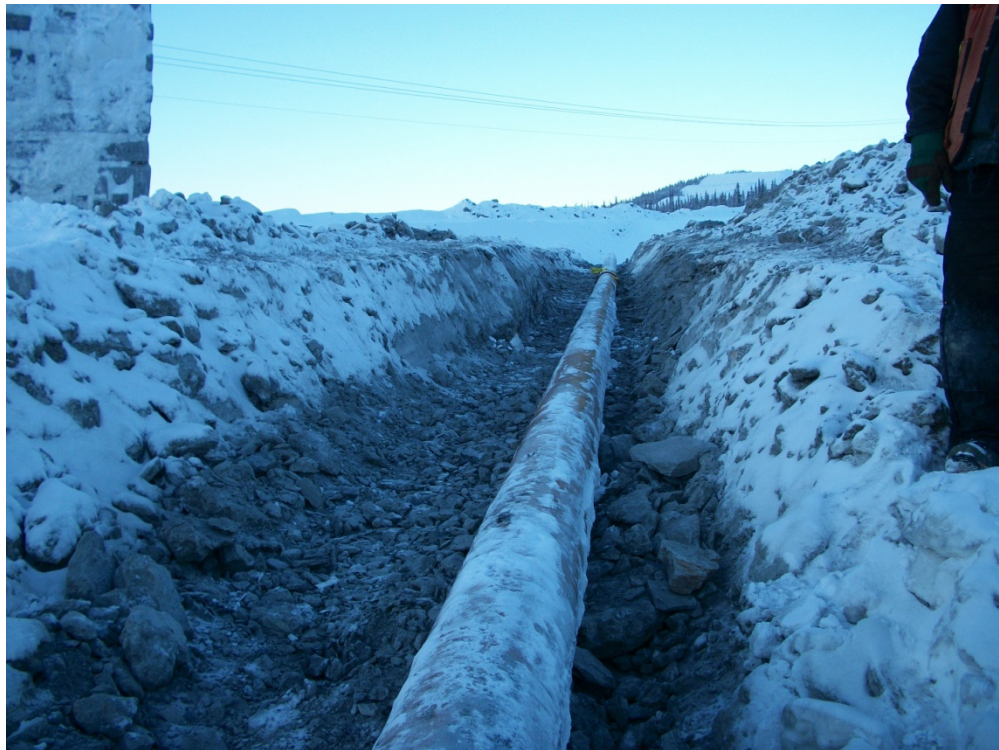
Installing V15 Pipeline Culvert
