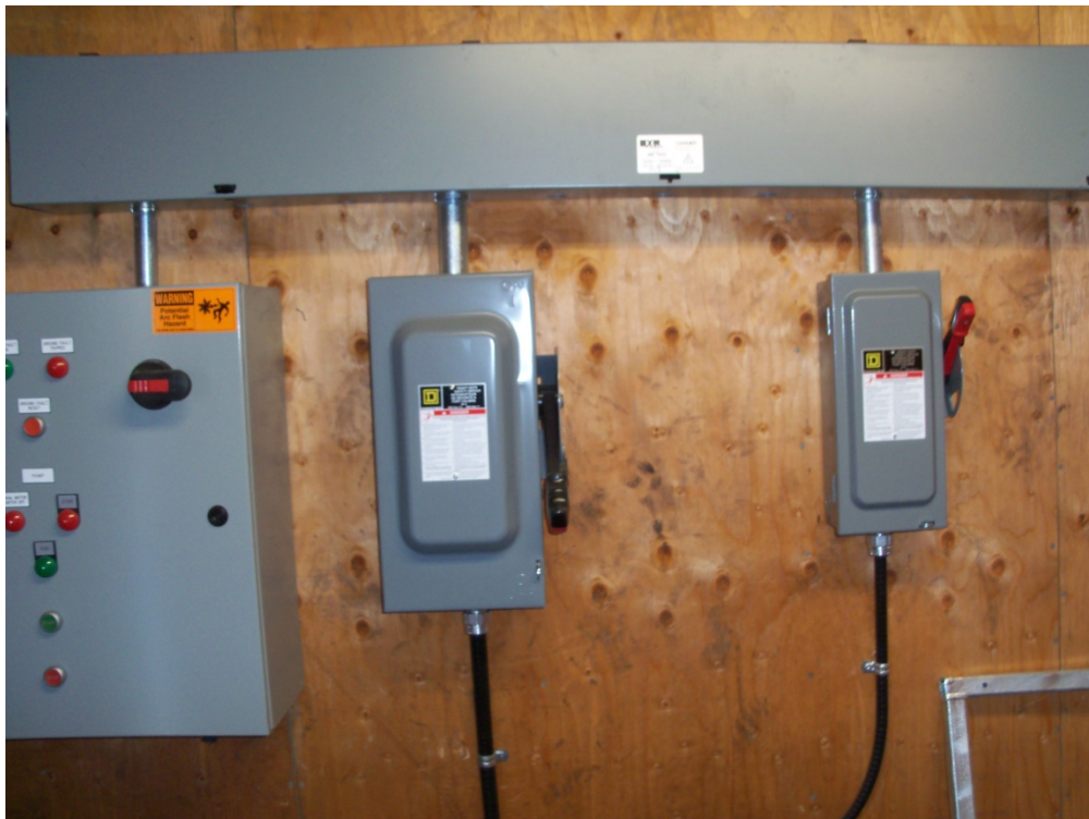
60A Heat Trace Disconnect – 30A Heater Disconnect
