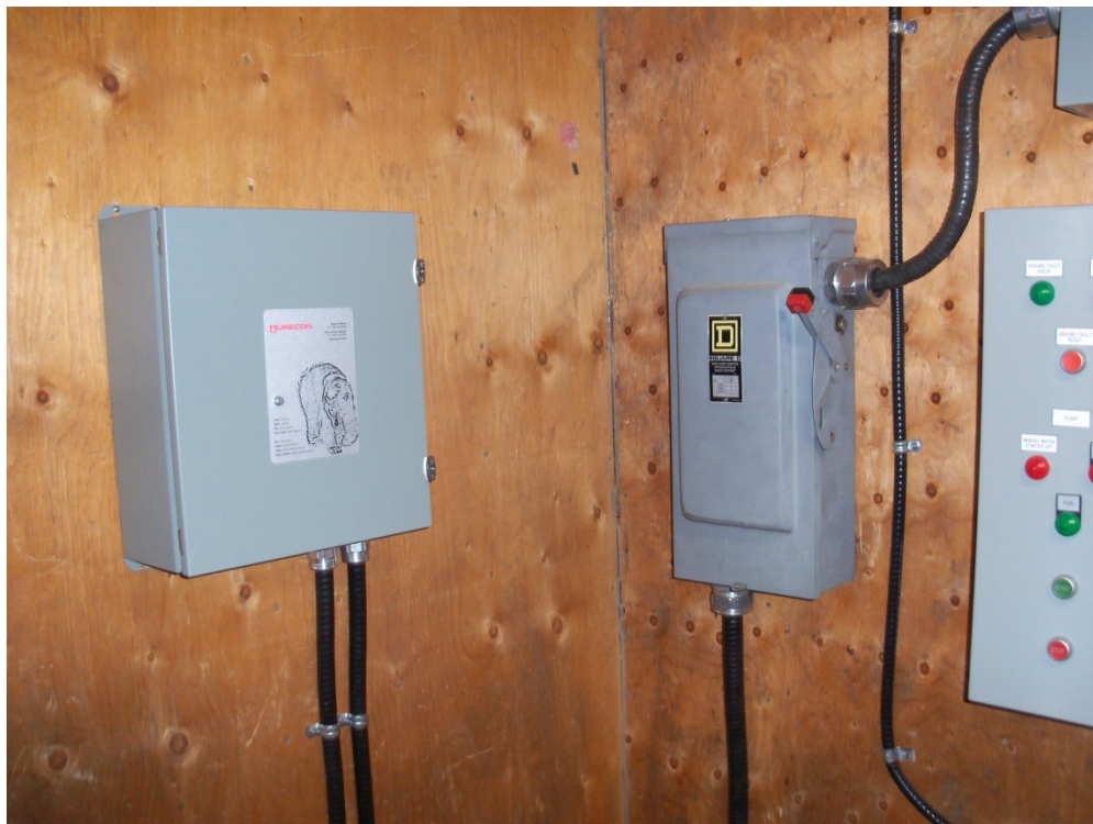
Heat Trace Controller and 100A Main Disconnect
