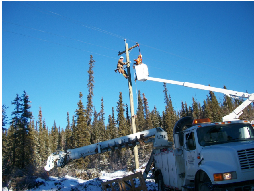
Installing Highline Switch
