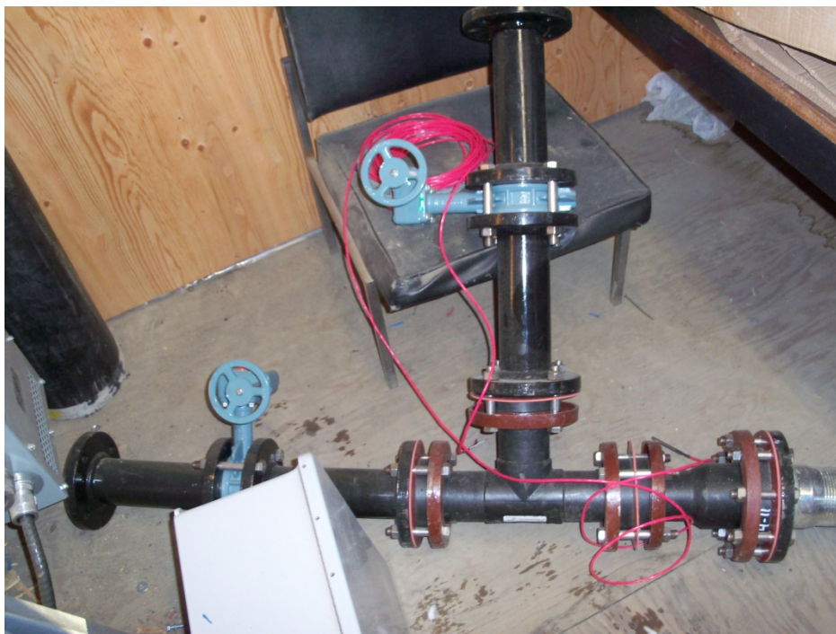
Pump Bypass / Drain Manifold
