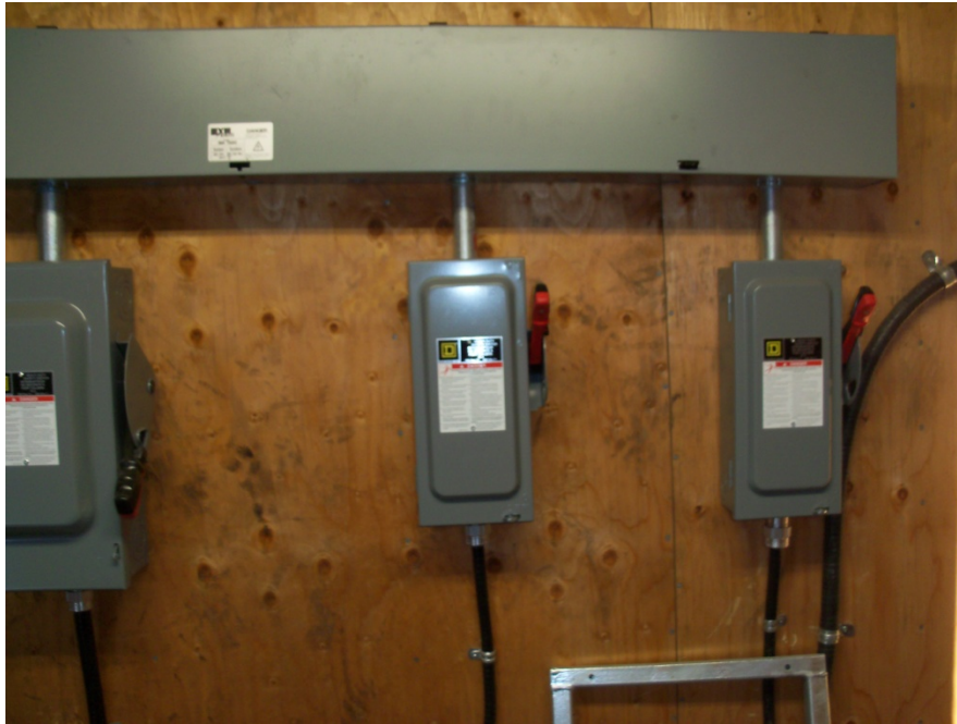
30A Heater Disconnect – 30A Lighting Trans. Disconnect
