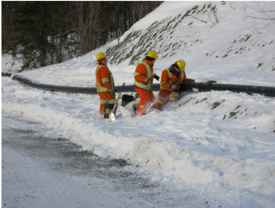
Installing Insulation Joint Kits
