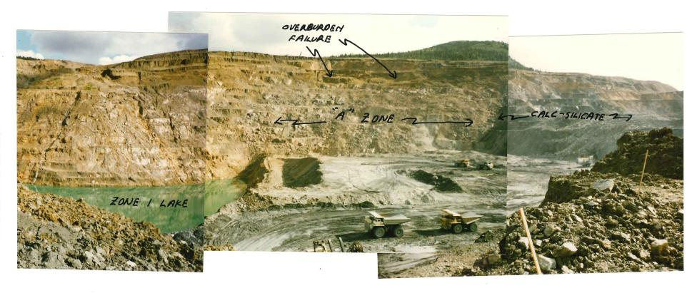
PHOTO 1. Northern portion of East Wall. Note "A" Zone and calc-silicate portions of wall. Also note overburden failure on "A" Zone wall.
