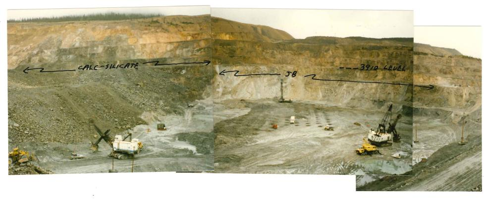
PHOTO 2. Southern portion of East Wall. Note calc-silicate and JB portions of wall. Also note 120 ft (36m) high slope below 3910 level and failure next to calc-silicate buttress.
