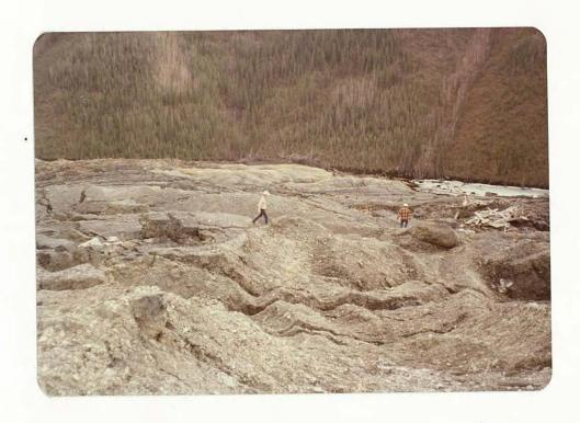
6. Porcupine Creek dump, looking East from crest. Note extremely broken surface in foreground, indicating large vertical and horizontal movement, and graben-like development. Note also debris and trees pushed up against the valley wall at the base of the dump.
