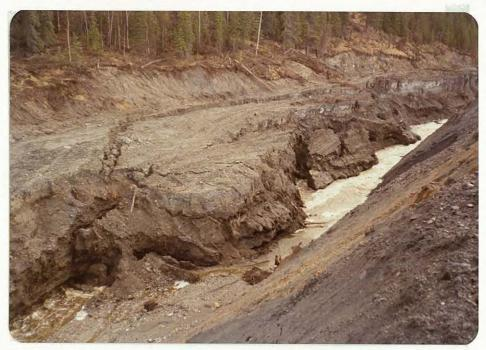
4. Clinton Creek discharge, May 5, 1976, looking downstream at a location opposite dump monitor No. 3. Note undercutting of in situ material on left bank.
