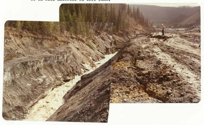
5. Clinton Creek discharge looking downstream, between dump monitors Nos. 1 and 2. Note cracking at top of oversteepened right bank.
