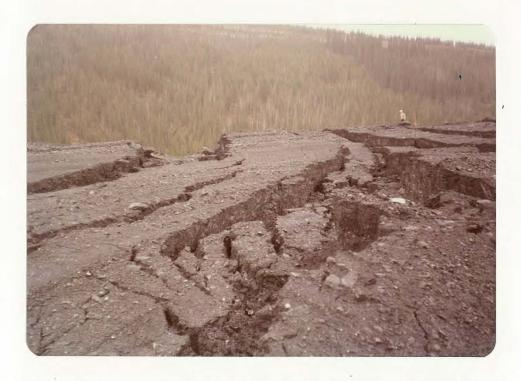
View looking North showing cracks in Clinton Waste Dump. Dump monitor No. 7 on right.
