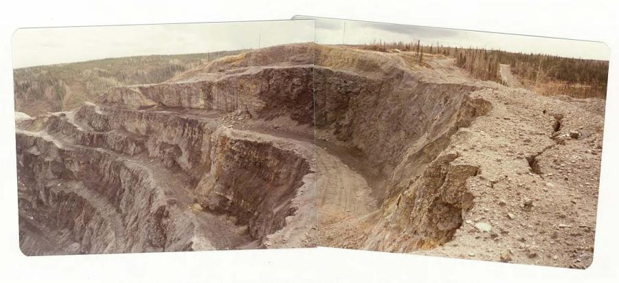
9. West wall of Porcupine Pit. Note cracking at rim of pit, and numerous cases of ravelling on the inter-bench slopes.
