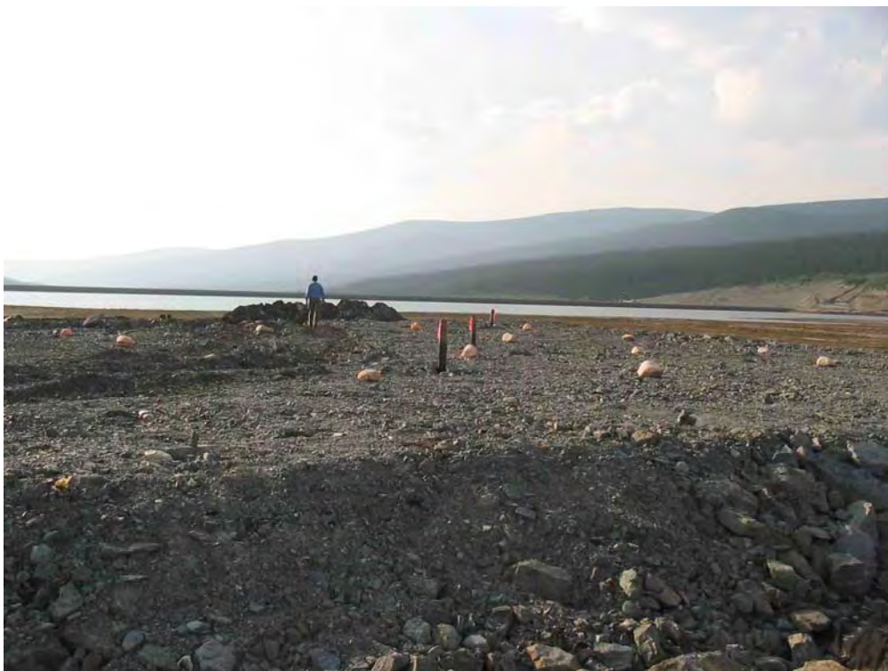
Figure 24. West test cover: Comparison of damaged SW and pristine NE portions of test cover.
