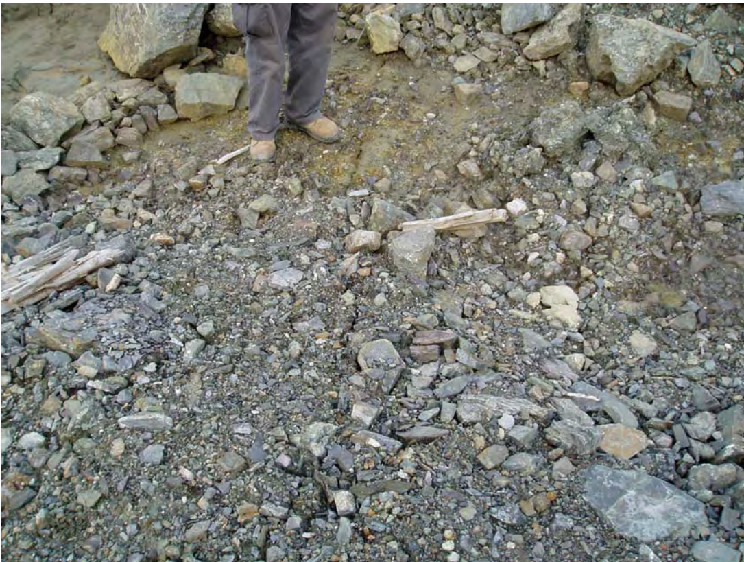
Photo 7: Close-up view of a crack on the corner of the East Pad. Note the crack continues from the tailings and on through the pad.
