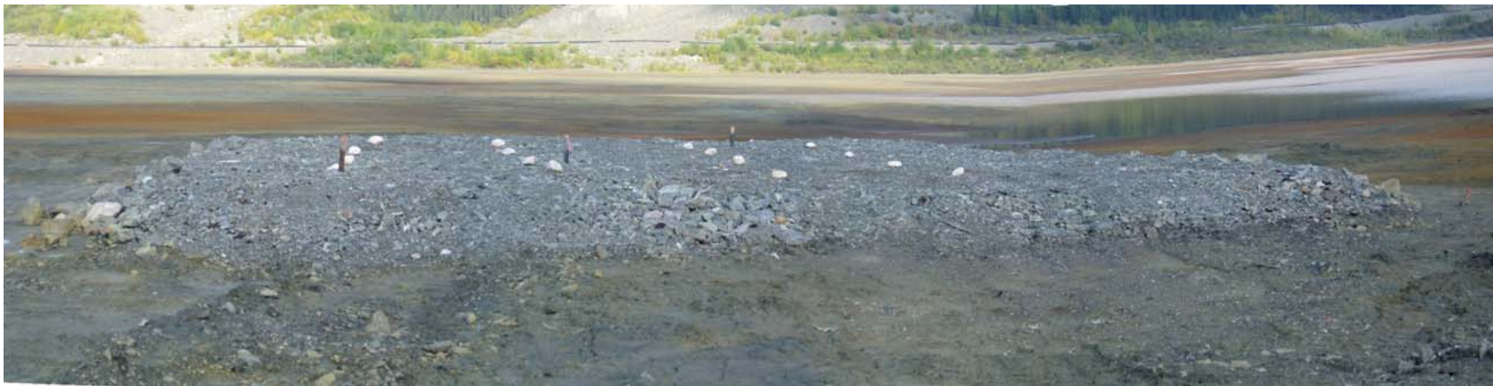
Photo 5: Panoramic of the East Pad from the south. Note the presence of standing water behind the pad. This water is not dammed up against the pad.
