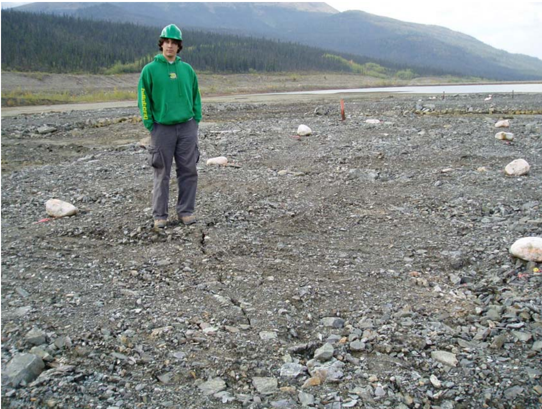
Photo 8: Close-up view of a crack on the surface of the East Pad. The crack is curved and measures approximately 5 m long, 10 to 20 mm wide and 10 to 100 mm deep.
