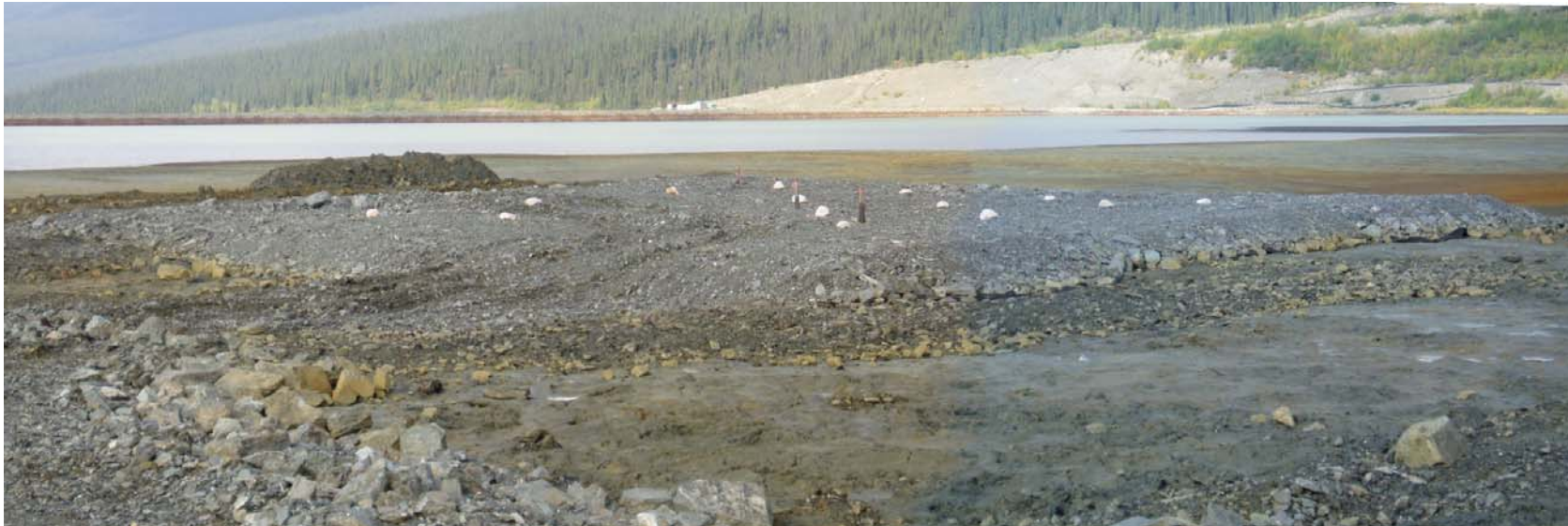
Photo 4: Panoramic view of the West Pad (including geotextile) from the south-west. Note the permanent pond in the background and the damage caused by the dozer in the foreground.
