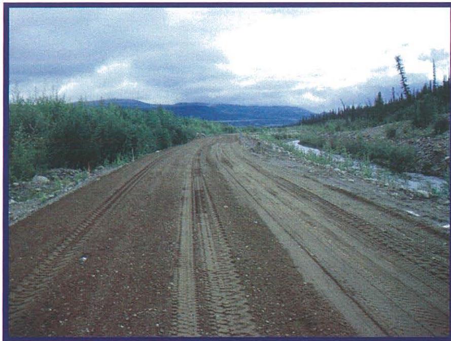
Photo 13 view looking to the east from station 0+650. In this section the third lift of gravel has been placed and bladed level in preparation for compaction.
