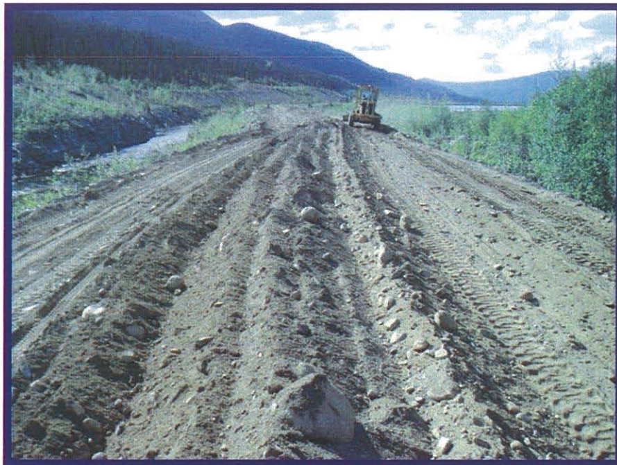
Photo 3 shows a view looking to the west from Station 0+750. Note this section is currently having the winter placed fill removed. This material is being windrowed into the central section. This material is being reused (with large cobbles removed) in the dike raising.
