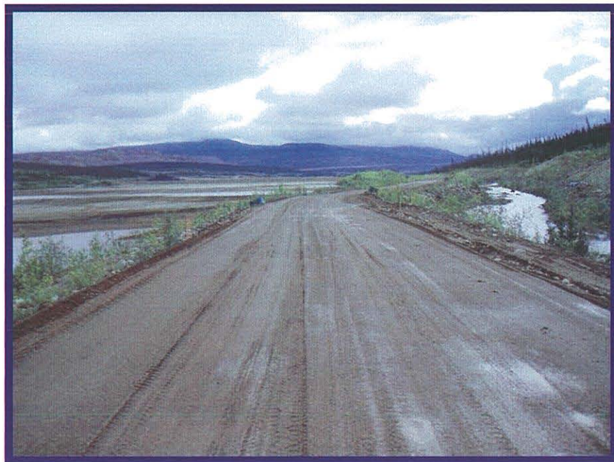
Photo 12 shows a view looking to the east from station 0+150. This shows the second lift of general fill (sand and gravel) currently being compacted.
