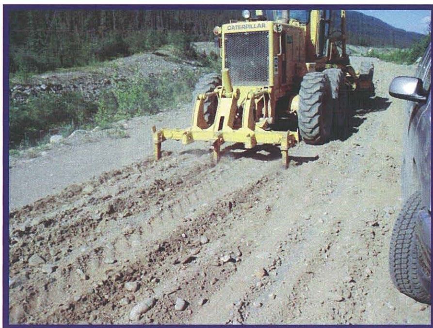
Photo 4 shows a view of the 160G grader as it starts to scarify the surface of the Canal Dike.
