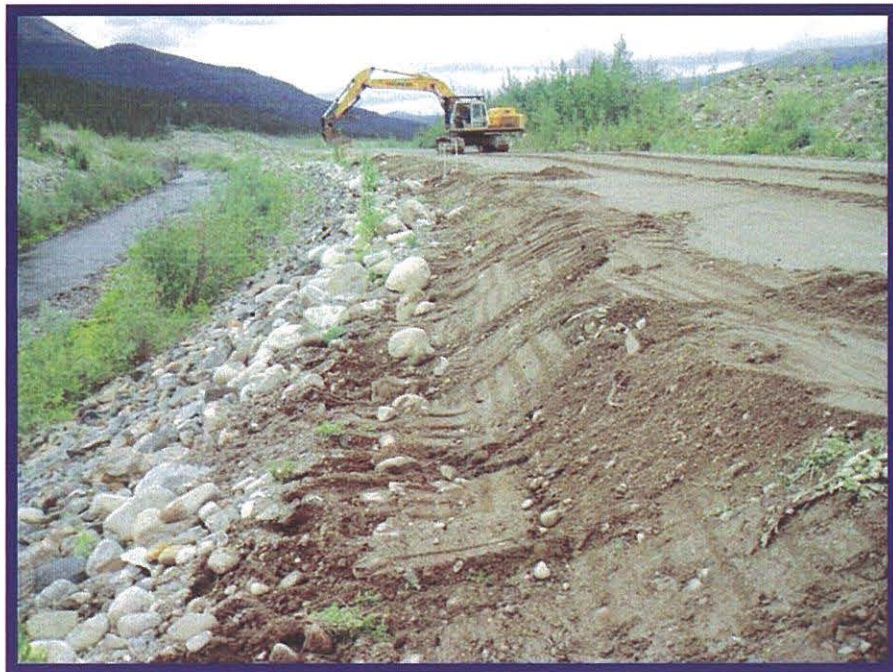
Photo 20 shows a view at station 0+825 of the prepared surface for riprap placement.
