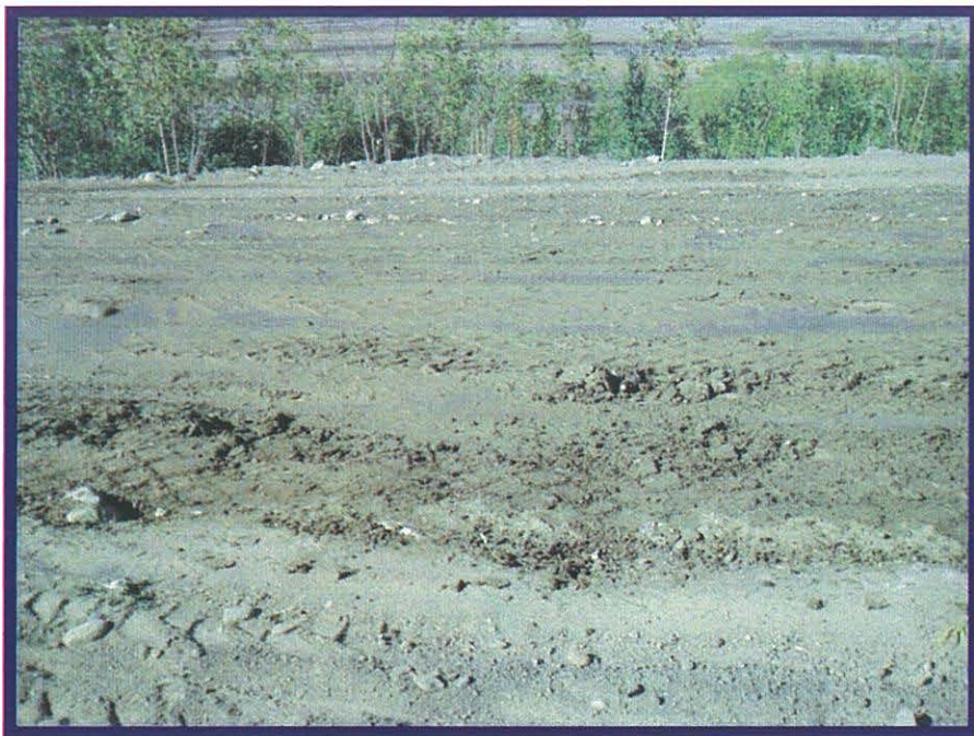
Photo 9 shows a view of the first scarified and compacted section of the Rose Creek Diversion Canal Dike, looking to the north from station 1+000. Note the application of water.
