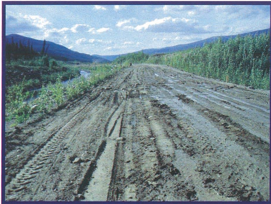
Photo 7 shows a view looking towards the west from Station 0+950. Note on the right hand side of this photo that water has been placed and compaction started and on the left hand side no water has yet been placed.
