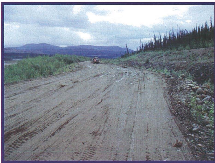
Photo 10 shows the surface of the scarified and re-compacted surface. This photo is taken looking to the east from Station 0+525.
