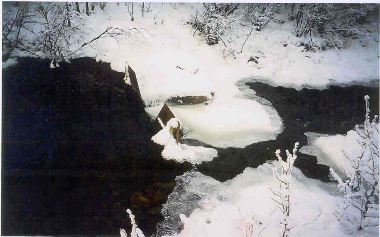
Photo. 6 V-notch weir plate in discharge channel. Note flow bypassing plate on right hand side.
