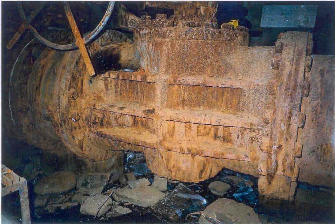
Photo. 3 Close up of plug valve. Downstream end unsupported except for what appeared to be a piece of timber
