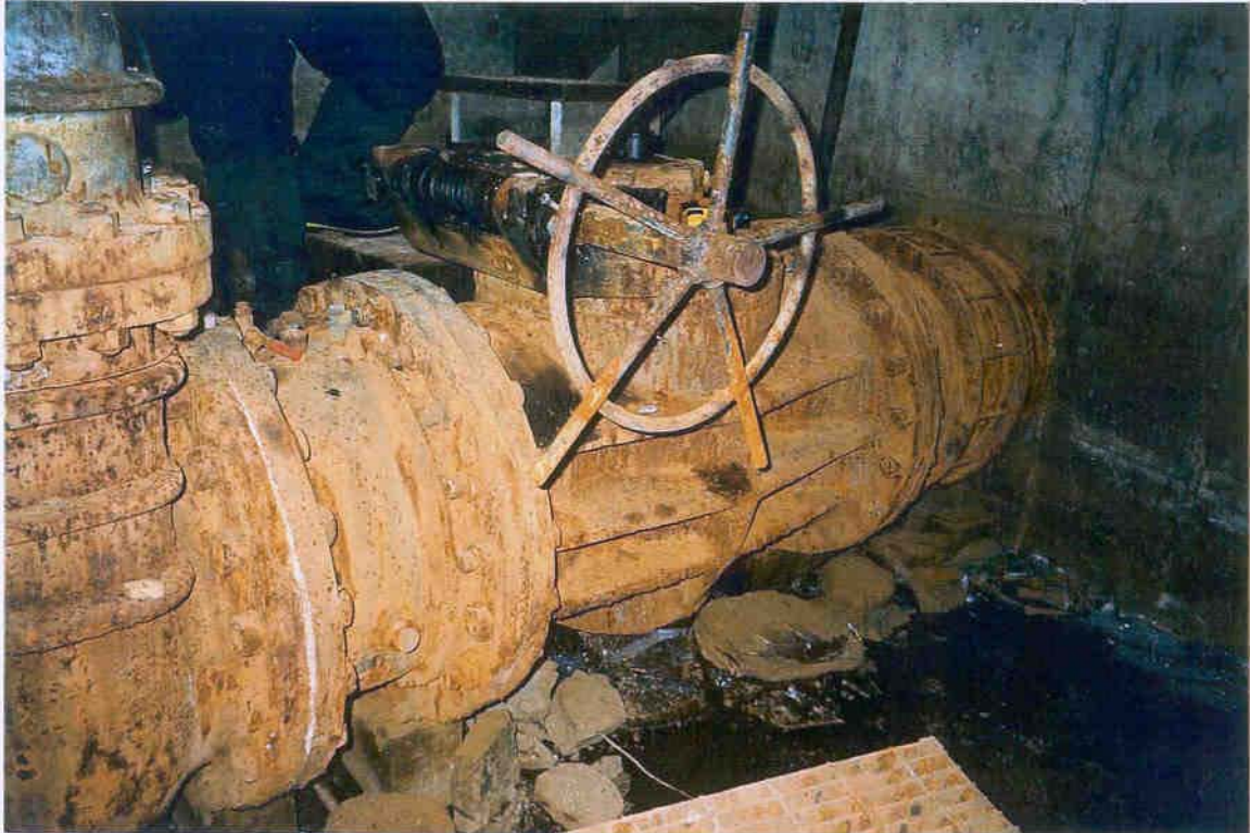
Photo. 2 Side view of spool piece and plug valve. Note small concrete plinths beneath flanges of spool piece, but not beneath d/s plug valve flange.
