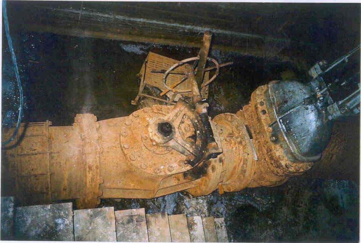
Photo. 1 Outlet structure valve chamber pipe work, flow is from right to left. Note spool piece between gate valve (at right) and plug valve.
