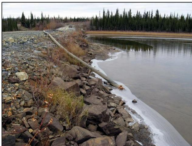
Figure 14 Upstream Armouring Along N Half
