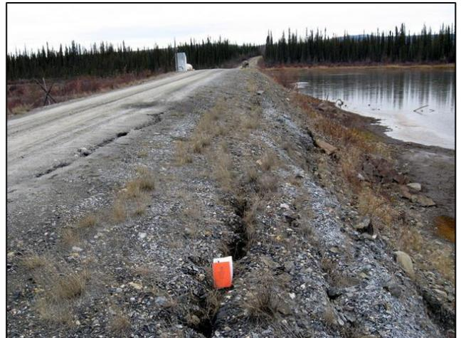
Figure 23 Tension Cracks Extending to CL
