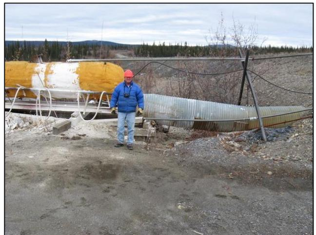
Figure 11 Settlement of Lime Plant Inlet Pipe
