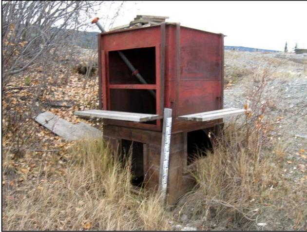
Figure 08 U/S Decant Weir in S Abutment of Dam 1
