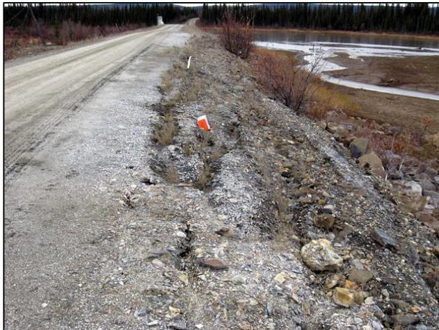
Figure 22 Tension Cracks and Slumping
