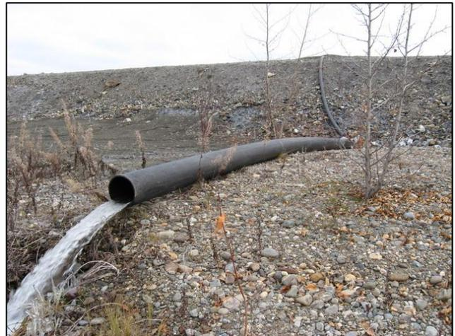
Figure 07 Siphon Discharge into Pond 2
