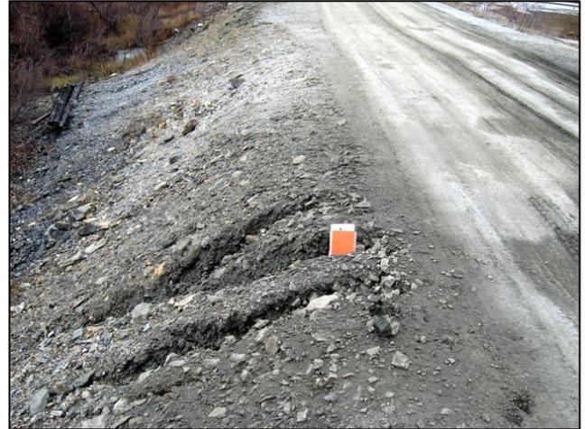
Figure 21 Rilling on D/S Edge of Crest
