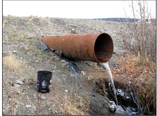
Figure 41 Decant Structure Outlet Pipe
