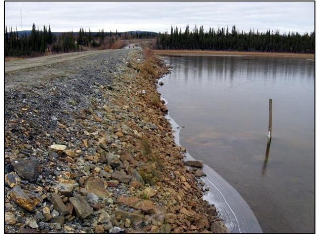
Figure 13 Upstream Slope at Staff Gauge
