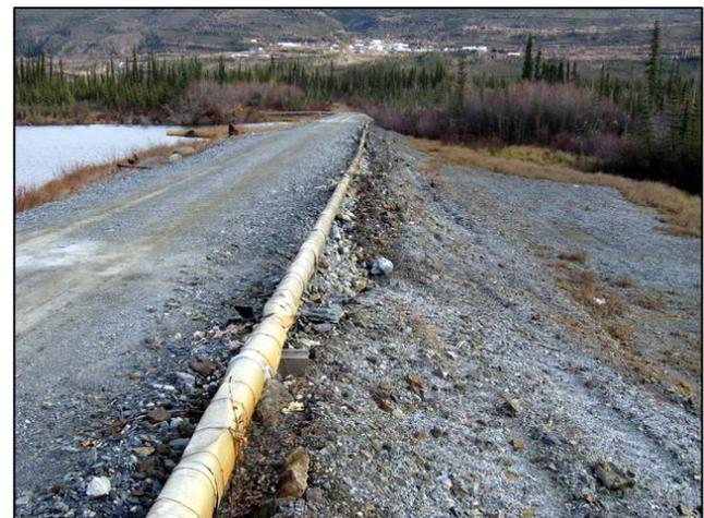
Figure 35 Granular Blanket on D/S Side of Dam 3
