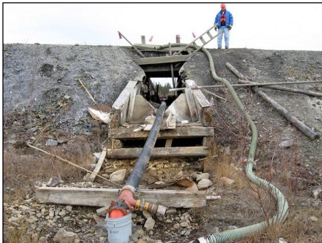
Figure 26 D/S Side of Weir Showing Siphon
