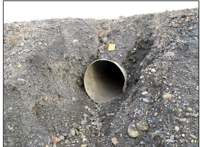
Figure 37 Erosion at Culvert Outlet
