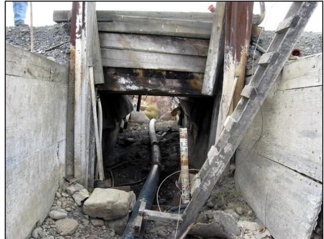
Figure 25 Upstream Side of Decant Weir
