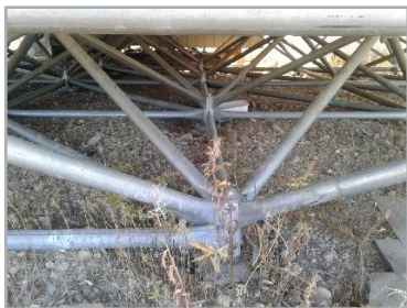
Figure 19: Shallow Foundation - Space Frame, Old Crow.
