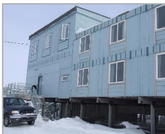
Figure 21: Adfreeze Piles Supporting Building, Barrow, Alaska (Thester11, 2008).
