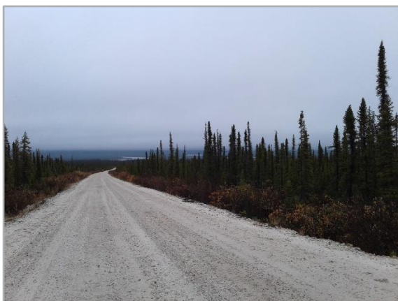
Figure 26: Light Coloured Crushed Quarry Rock Forming the Crow Mountain Road.
