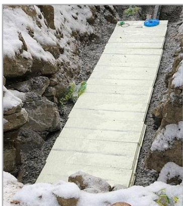
Figure 30: Extruded Polystyrene Insulation Mats Installed in Ground for New Water/Wastewater Trench in Norway (Øyvind Holmstad, 2017).
