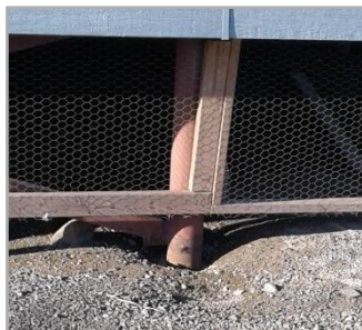
Figure 20: Pile Foundation for Building in Iqaluit, Nunavut.
