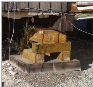
Figure 18: Shallow Foundation - Pad and Wedge, Old Crow.
