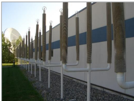
Figure 22: Thermosyphons at the Fairbanks Airport in Alaska, Used to Chill the Permafrost Beneath the Airport Structure (Ryu, 2008).
