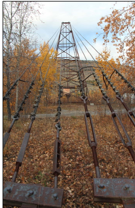
Figure 3. South Elevation of South Tower and Suspension Cable Members
