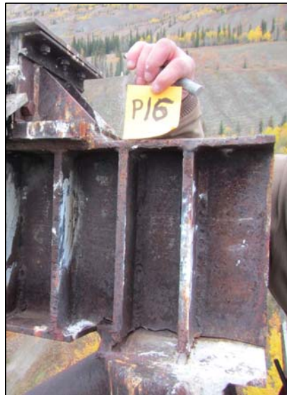
Figure 4. Damaged Steel Head Beam located on top of North Tower
