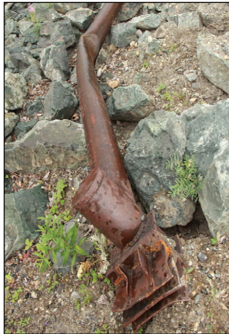
Figure 1. SW Sway Cable Anchor destroyed by flooding of Pelly River in early 2013
