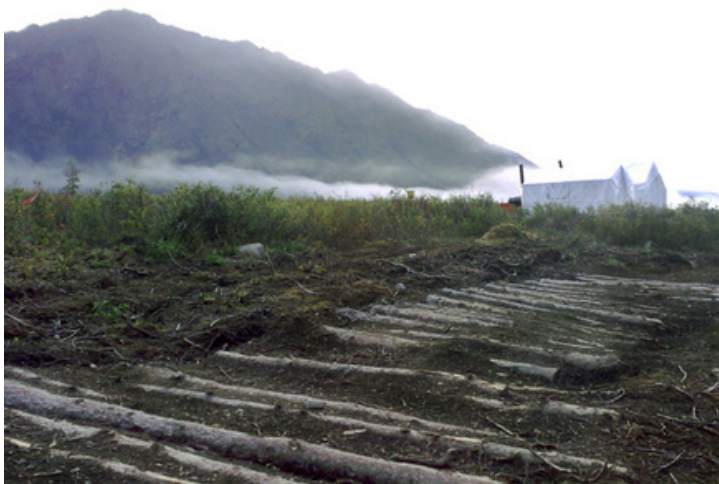
Corduroy road protecting permafrost to wall tents in Beaver River camp, Wernecke Mountains (Crawford, 2006)
