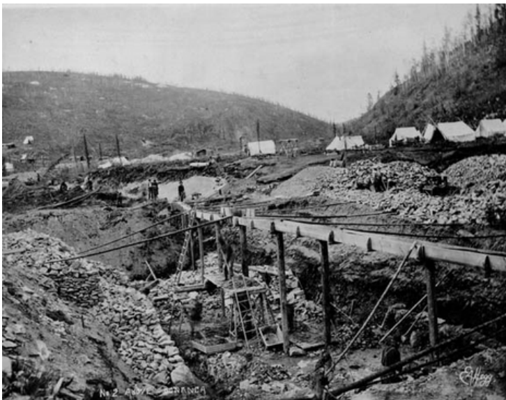
Working gold trenches and sluices, Klondike circa 1899 (Yukon Archives, photo 2190)
