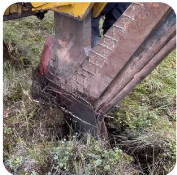
Middle left: the Rolligon plow in action as it cuts a trench and buries the orange conduit. Minimal impacts to the terrain are visible.
