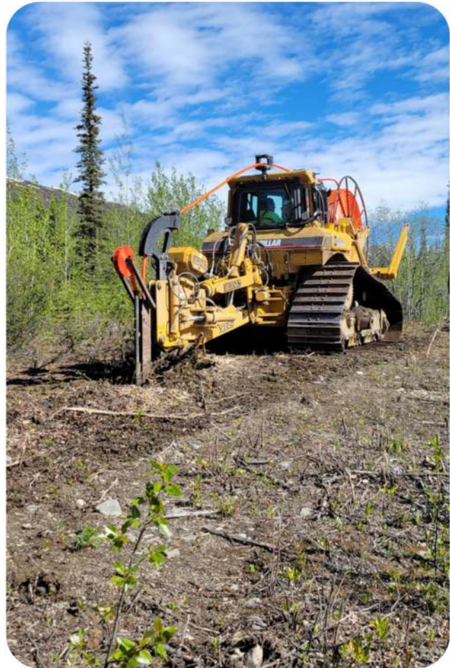
A conventional plow installing conduit.
