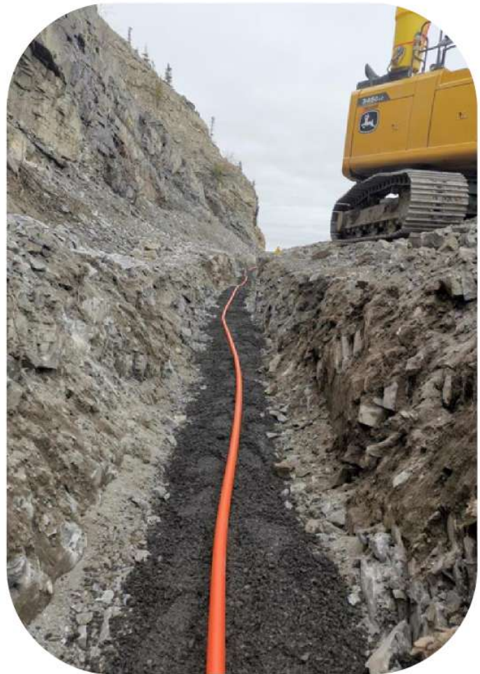
Conduit placed in a shallow trench, ready to be buried.
