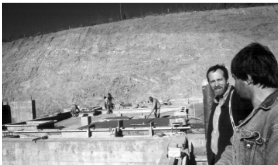
Figure 8. Jim Prock (foreground) of Minto Explorations explains construction of the mill of the Minto Cu-Au-Ag project to Hugh Copland (facing camera).
