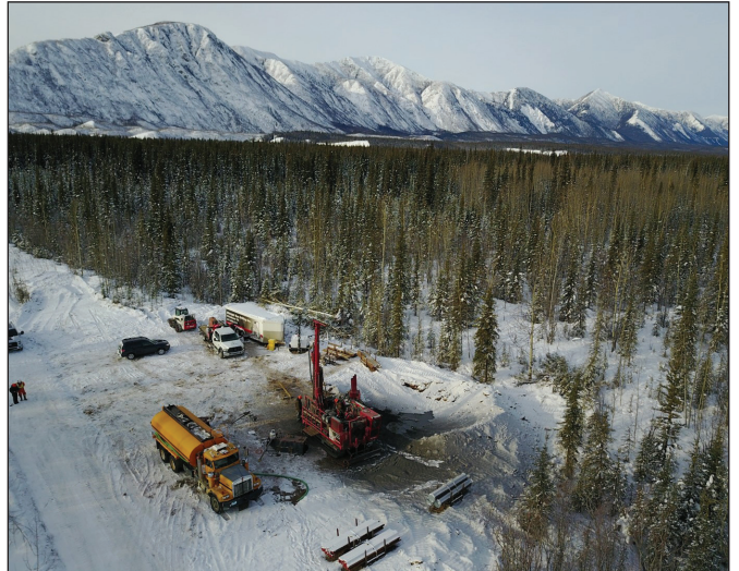
Figure 7. Photo of rig drilling the ground temperature monitoring well in the Tintina Trench near Ross River.
