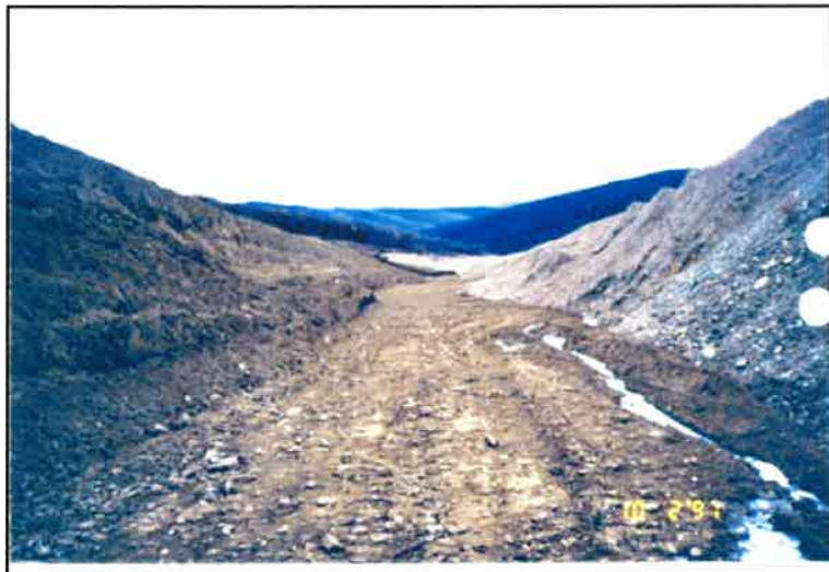
Figure 11. Looking downstream at flood plain during construction of stream channel.
