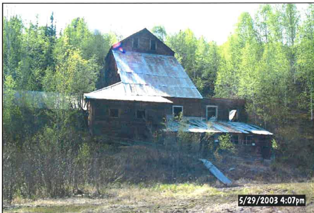
Figure 5. Historic Hi-YU mill building.
