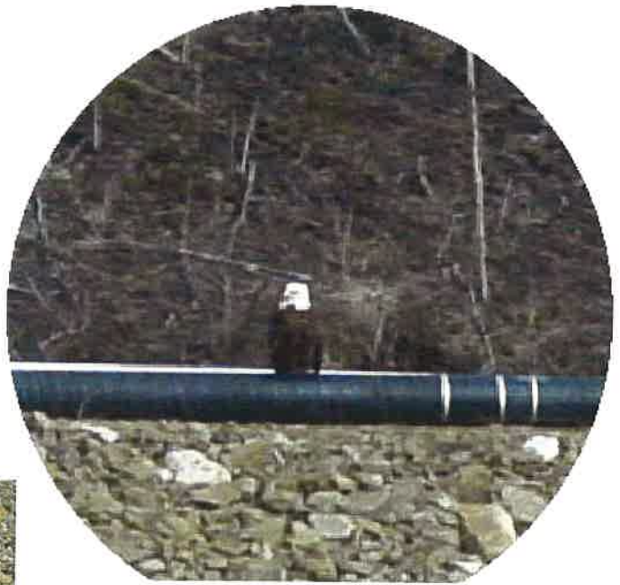
Figure 47: Bald Eagle perched on water pipeline next to road, with a good view to fishing grayling in the wetlands, May 2003
