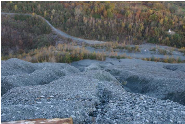
Crushed rock cover erosion
