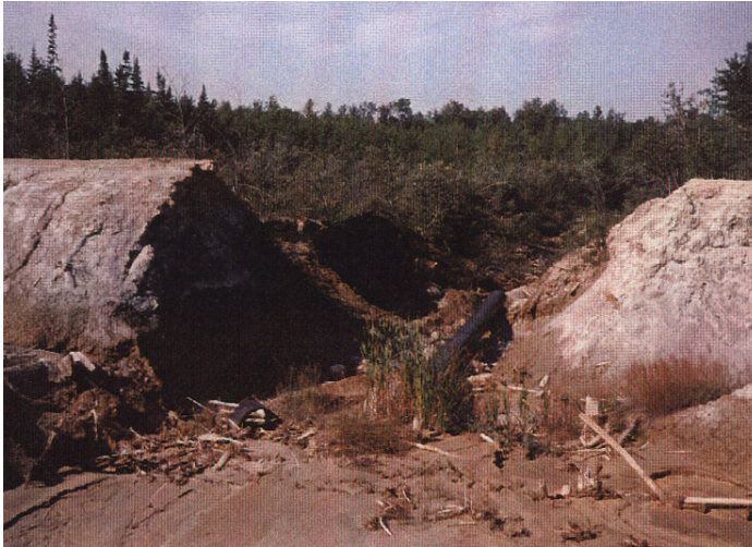
Tailings dam failure
