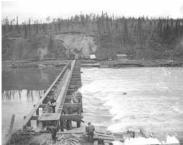
Above: Construction of the Marsh Lake dam in 1924.
