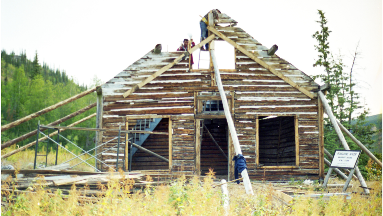
Cadzow Store, Rampart House, undergoing conservation, 2001. YG photo
