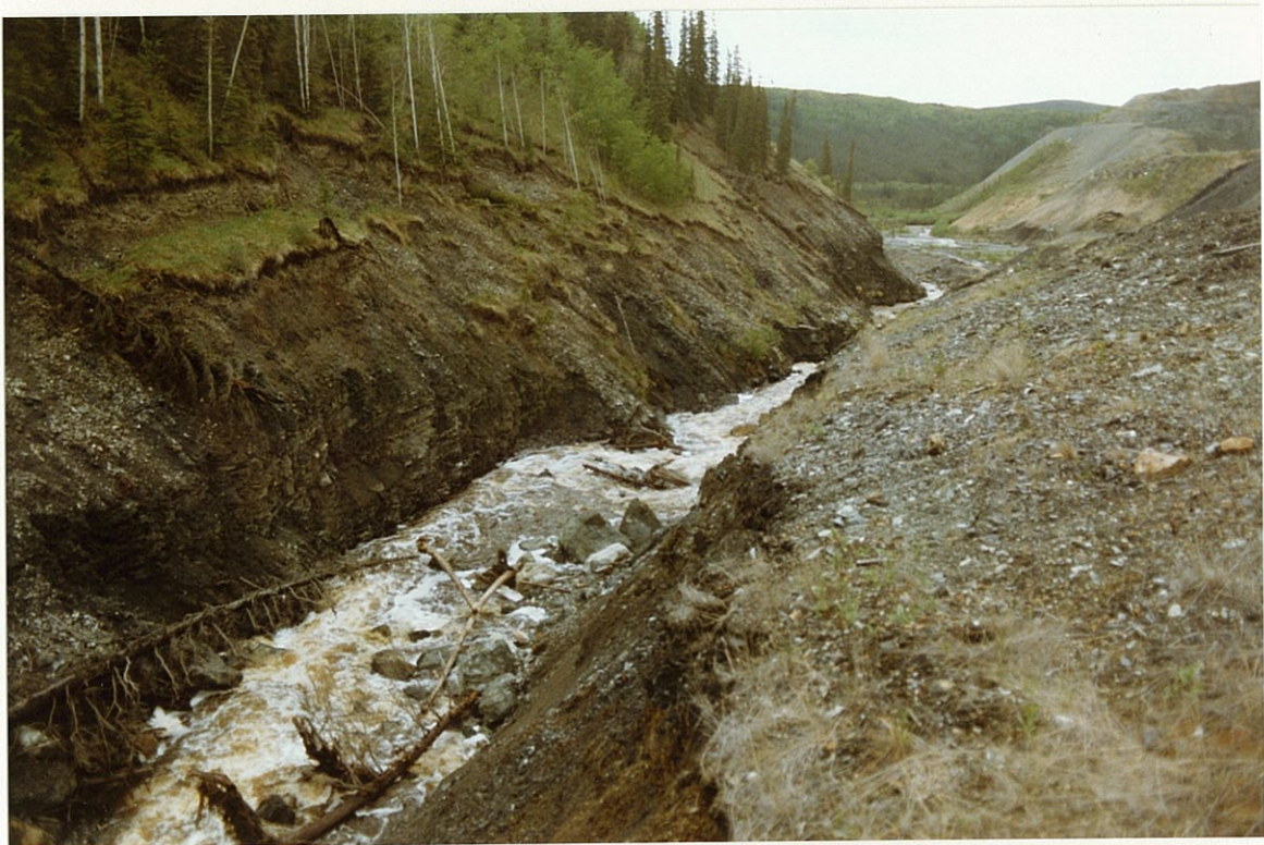
Photo 6: Waste dump channel looking downstream. Note left bank is protected by bedrock and stream bottom is armoured by large boulders from waste dump. June 1985.
