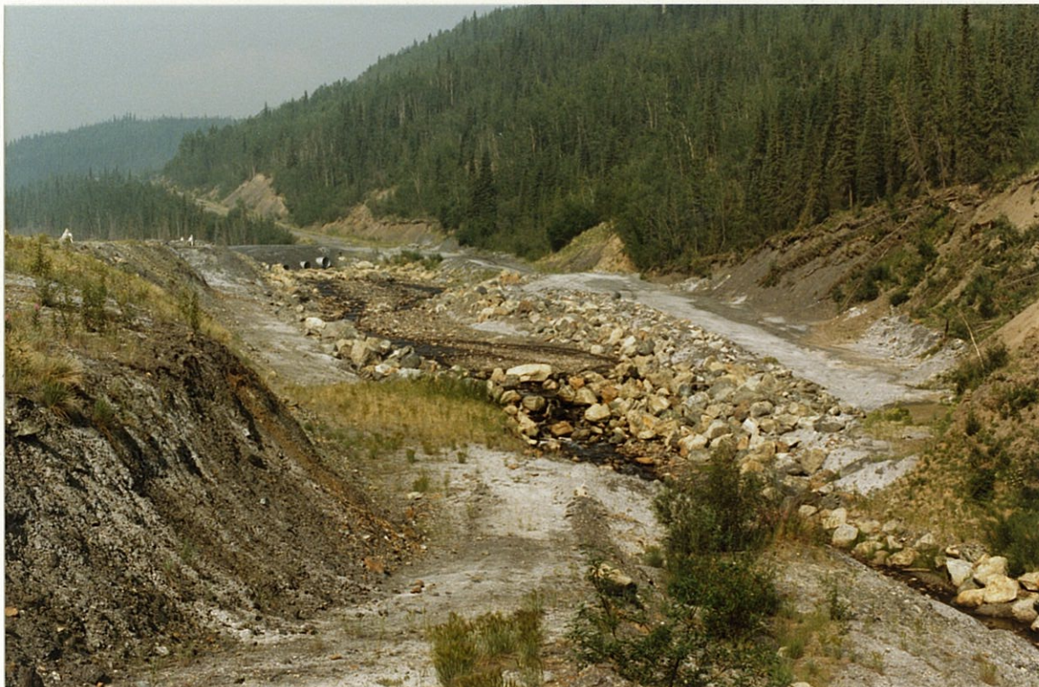
Photo 4: Rock lined section at upper end of Clinton Creek channel over waste dump. Access road culverts at upper left. July 1986.
