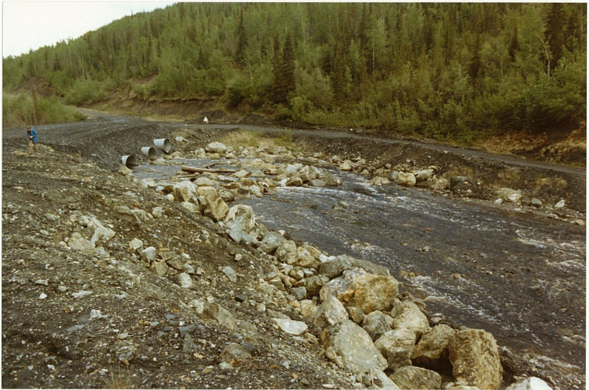
Photo 5: Access road culverts at upper end of waste dump channel. June 1985.
