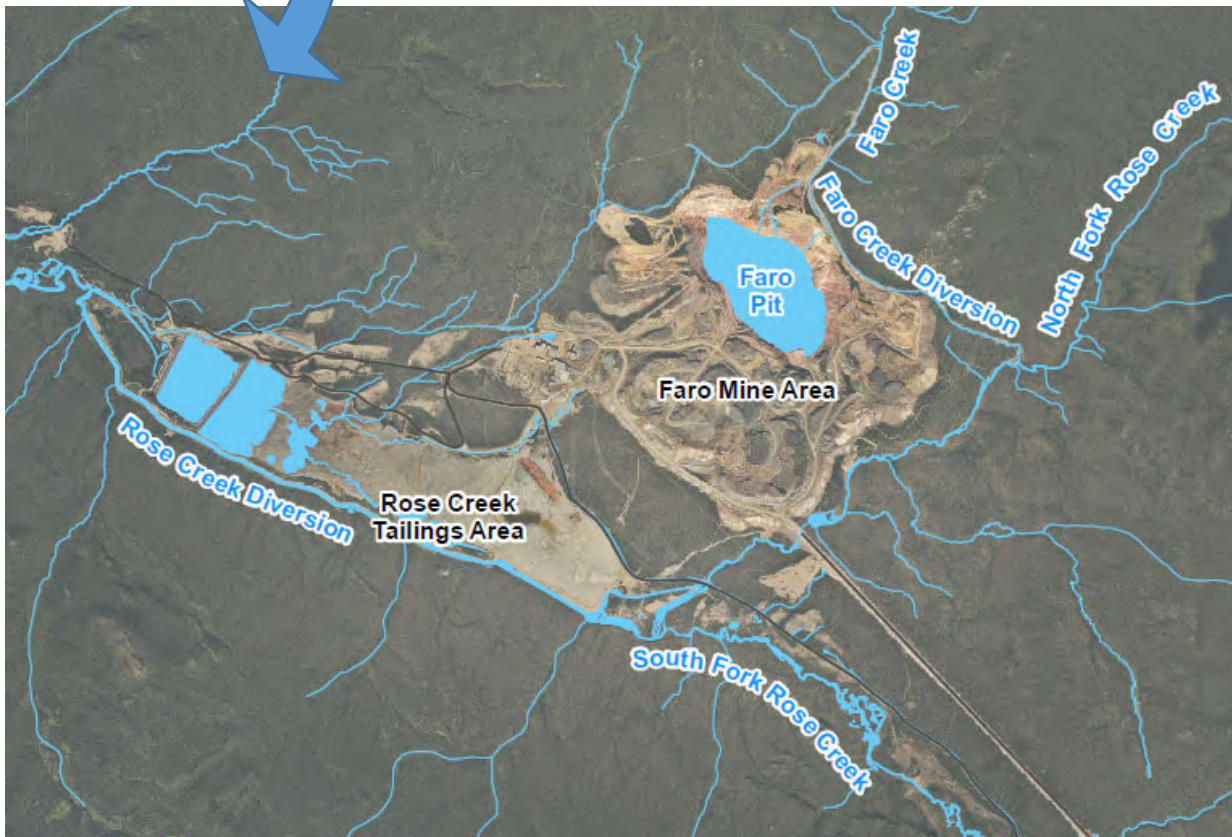
The Faro Pit, Waste Rock Dumps, Faro Mill, and Emergency Tailings Area
