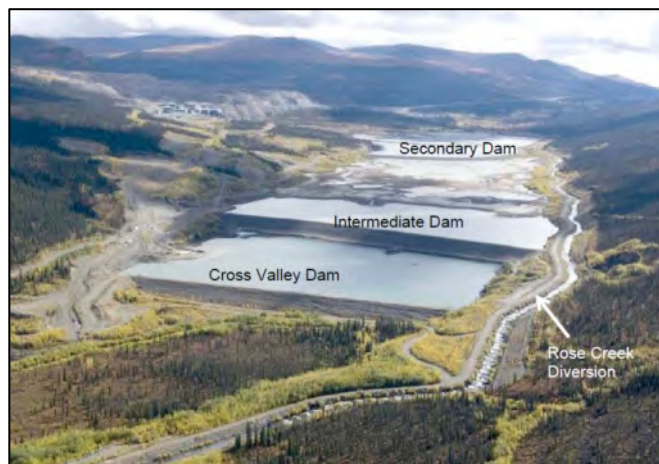
Tailings Dams in the Rose Creek Tailings Area
